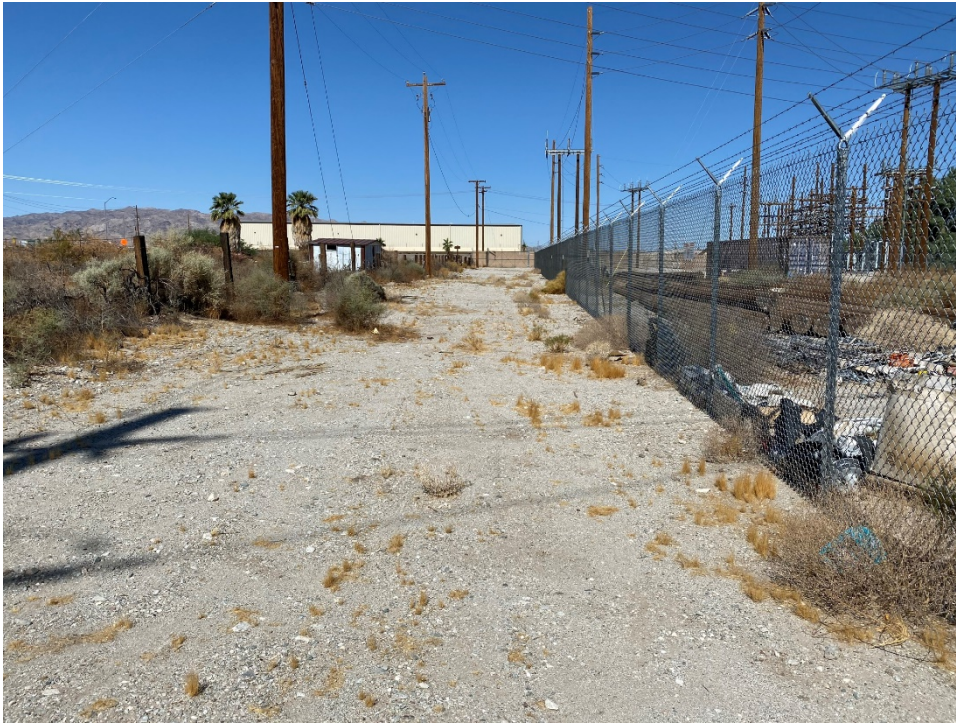
Photo 3 – Southern edge of parcel, facing west. Showing existing access road alignment.
