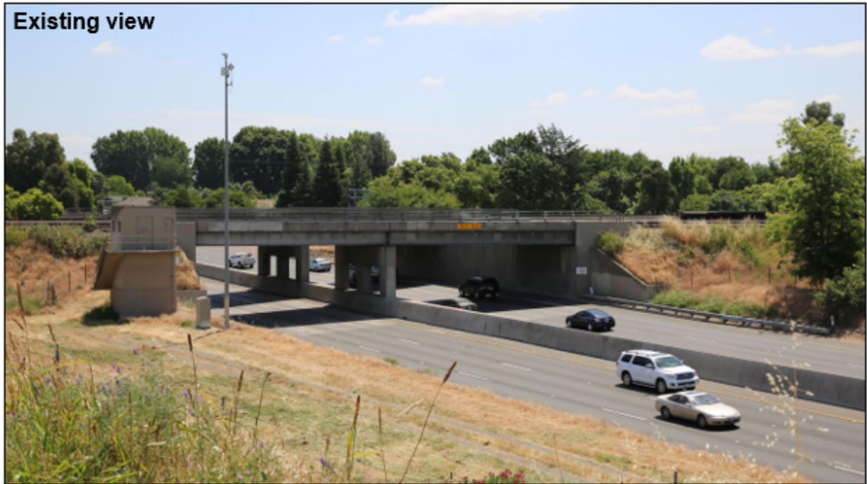
Figure 3.1-3. Key Viewpoint #2 - Existing and Simulated Views of Elvas Railroad Bridge Crossing near UPRR Wye (view looking southeast from westbound shoulder of Capital City Freeway)
