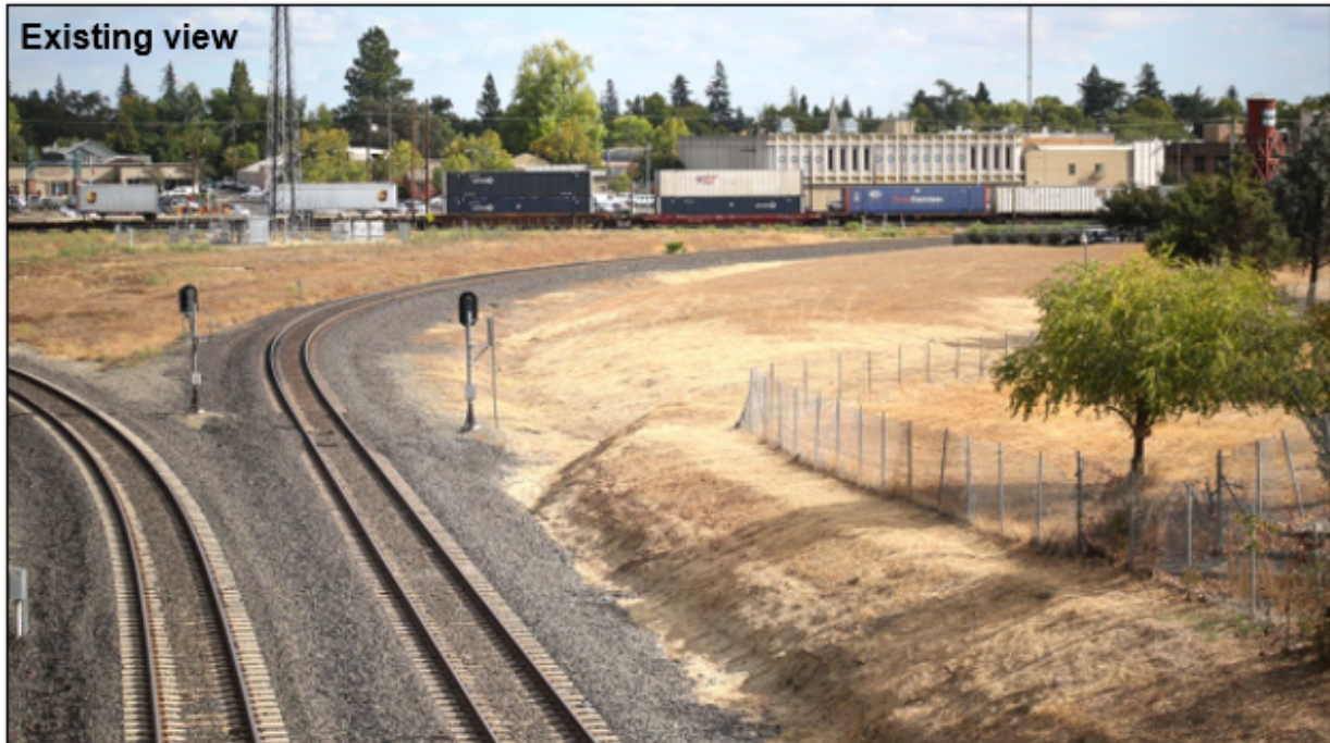
Figure 3.1-6. Key Viewpoint #9 - Existing and Simulated Views of 2015 EIR Passenger Train Layover Facility Site (view looking southeast from Sierra Boulevard overpass)
