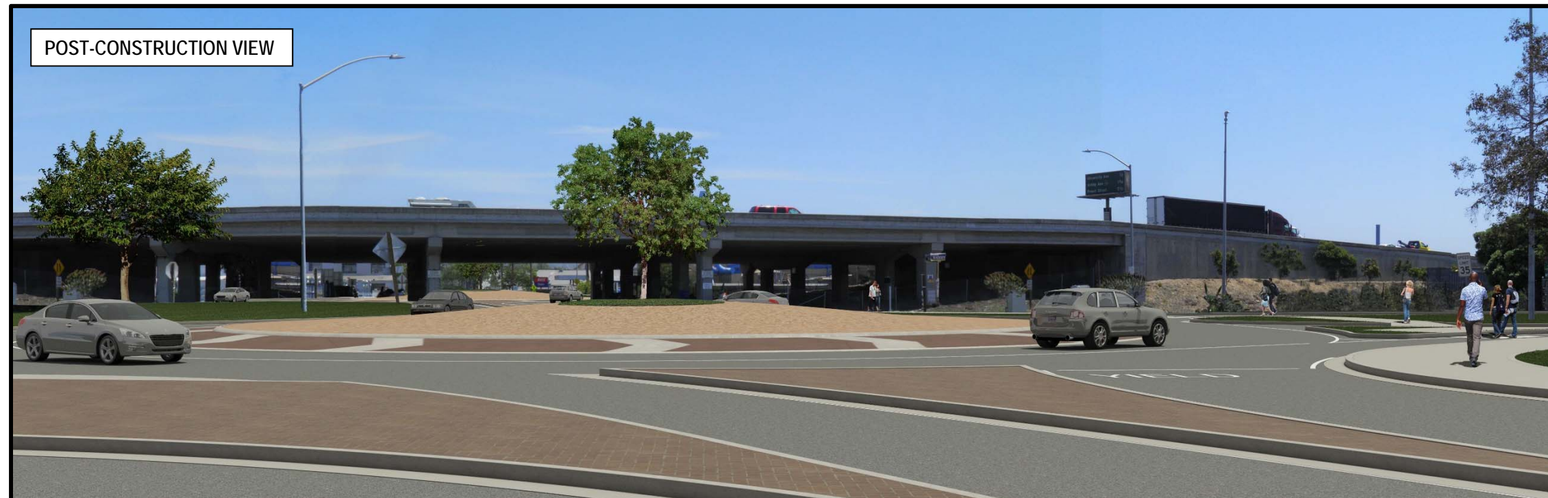
Figure 19: Key View #4 from the Golden Gate Fields Service Entrance looking southeast towards the existing Gilman Street undercrossing and the WB on-ramp. Note that the treatment of the islands, including the planting and paver etc. designs, are subject to approval and may not represent the final constructed conditions.
