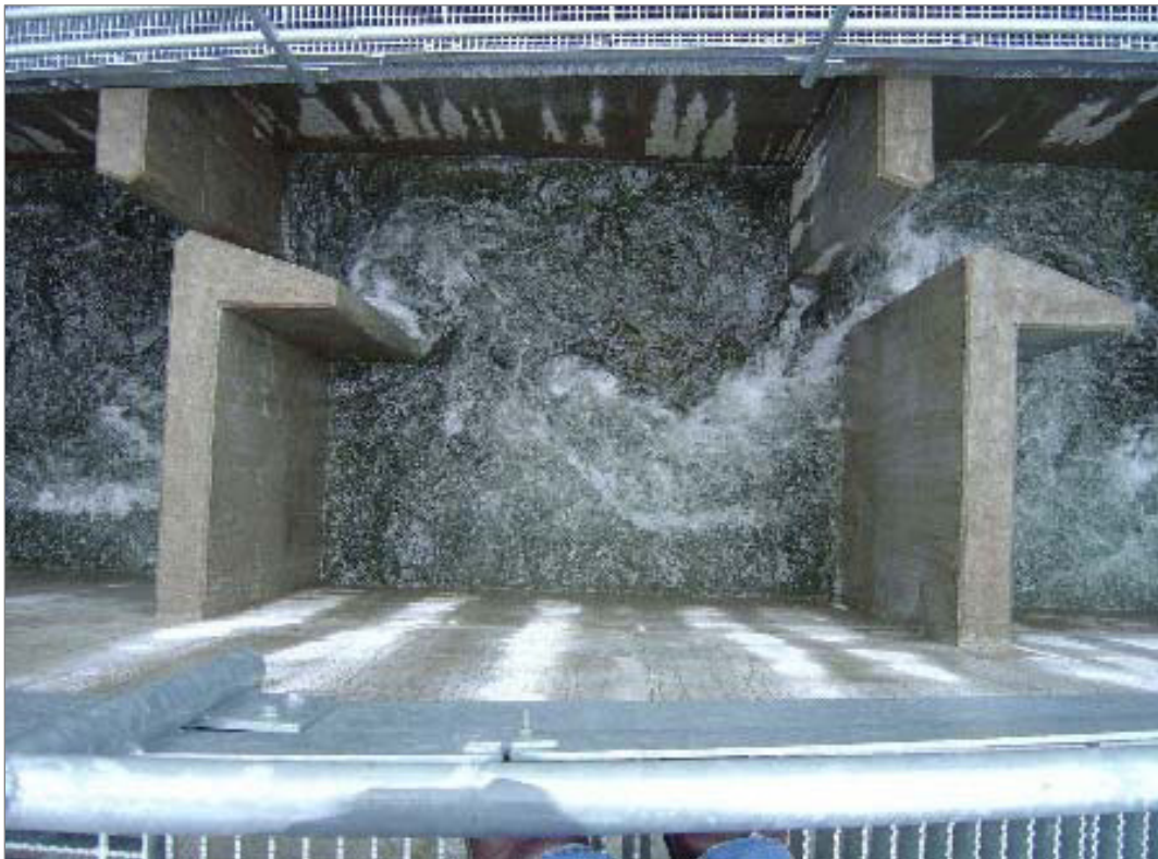
Figure 9 Typical Vertical Slot Ladder Pool
