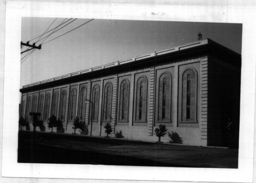
217-15 601-45 Embarcadero (P.G. & E. Station C) 5/82
