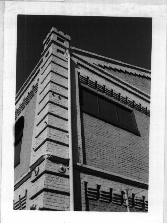
219-15 Corner detail, 64 Grove St. 5/82
