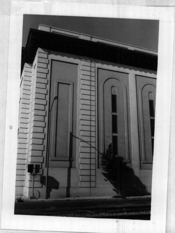
217-24 601 & 605 Embarcadero (P.G. & E. Station C) 5/82
