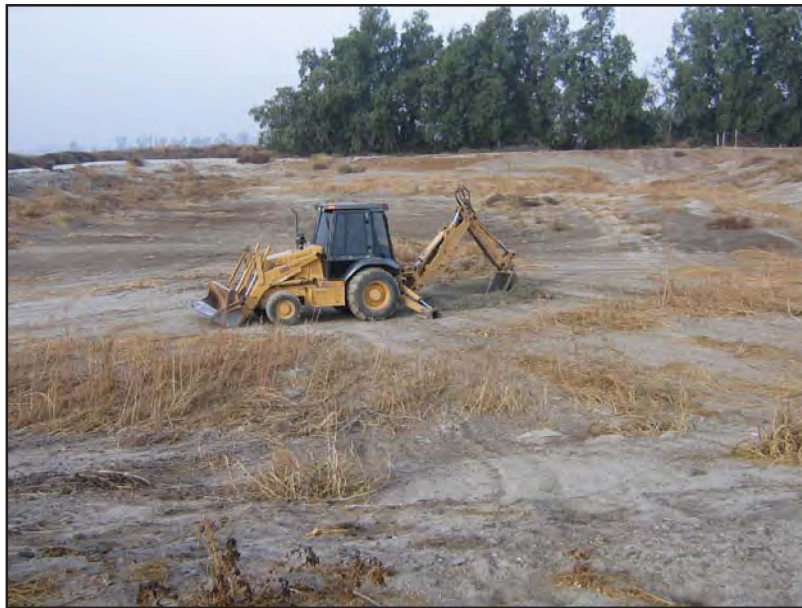
Southwest Wastewater Pond
