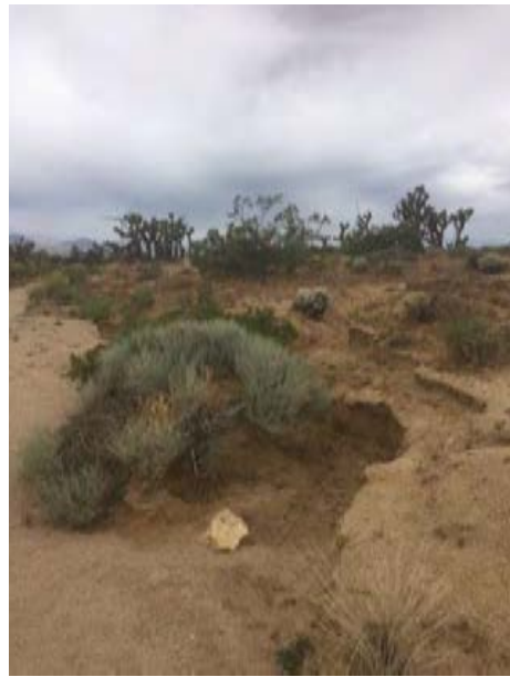
Photo 14: Data Station #4. Evidence of scouring.
