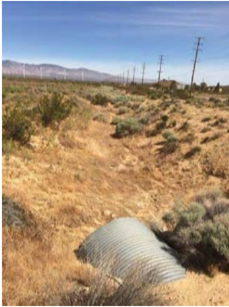
Photo 45: Data Station #14. Culvert (inlet); facing north.
