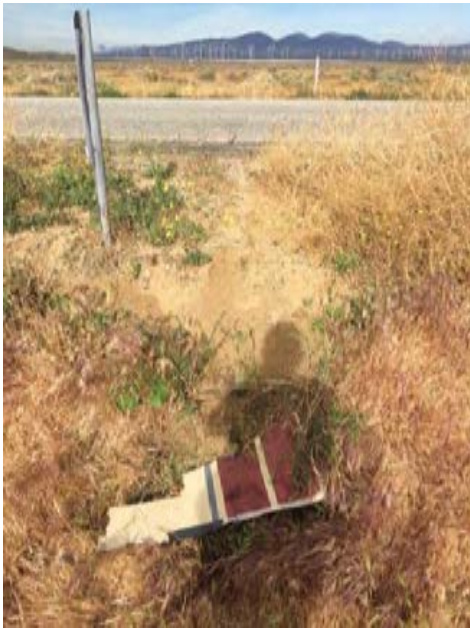
Photo 43: Data Station #13. Culvert; facing west.
