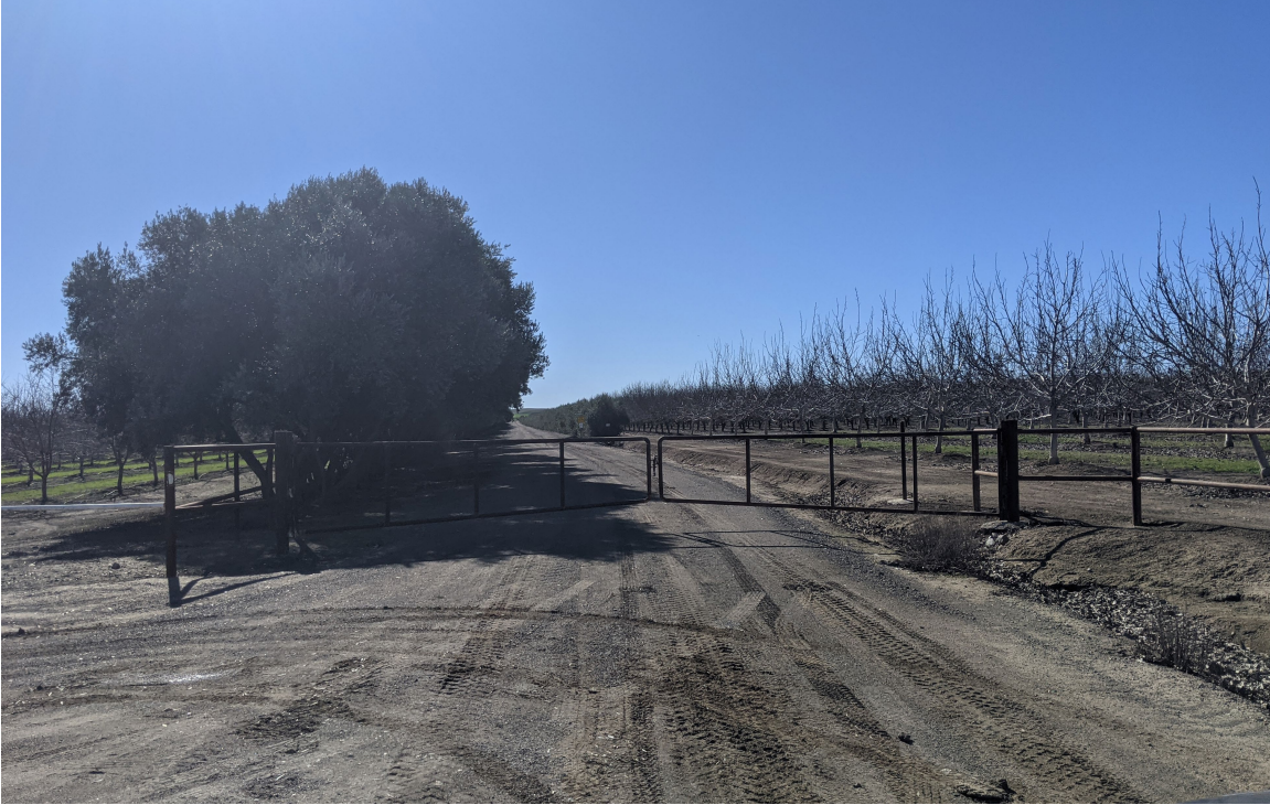
Photo 1: View of Dunnigan Pipeline alignment looking west from the intersection of Road 8 and Road 89A (Alternatives 1, 2, and 3)
