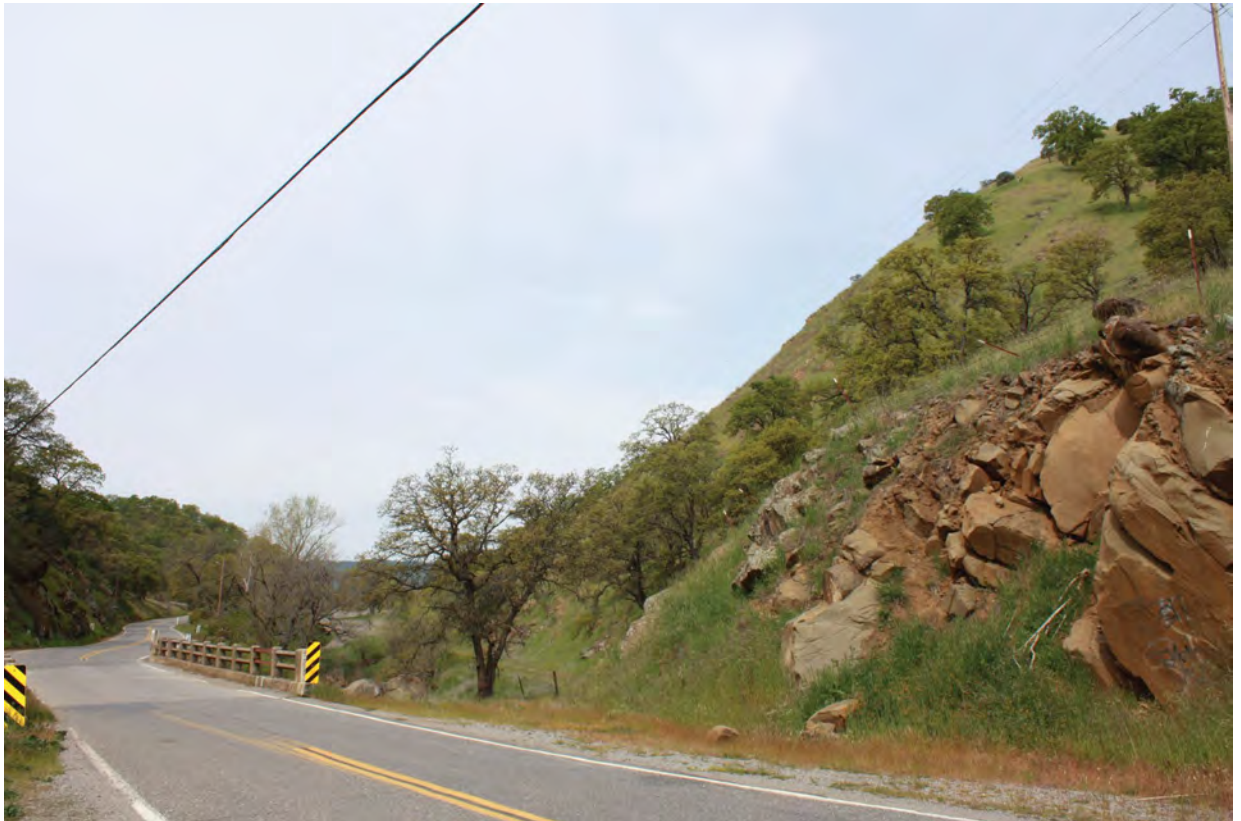
Photo 9: Looking west along Maxwell Sites Road toward the Sites Dam left abutment location, from outside of the inundation area.
