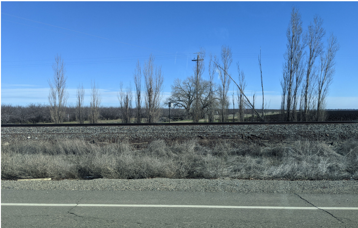
Photo 5: View of Dunnigan Pipeline alignment looking east from Road 99W (Alternatives 1, 2, and 3)
