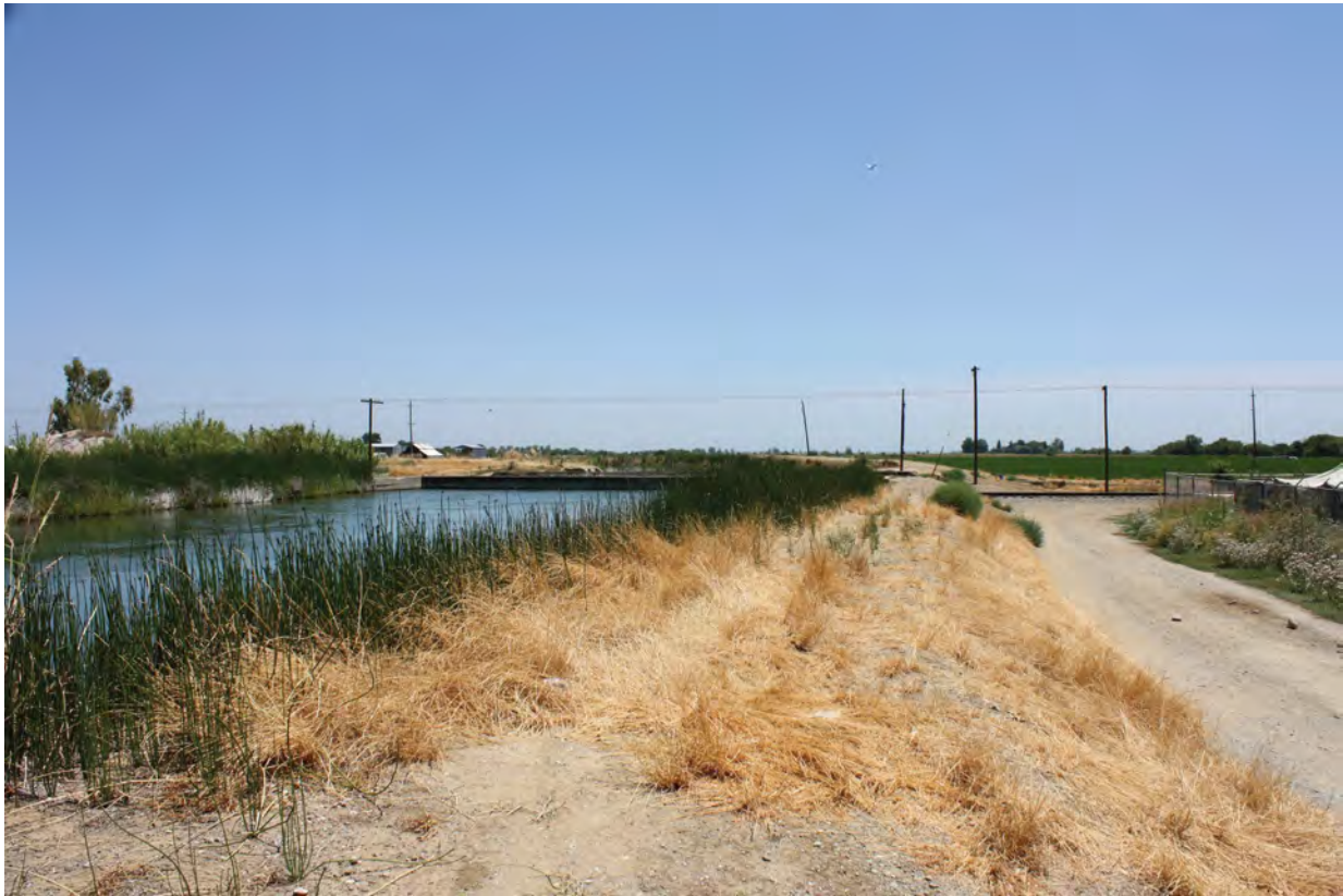
Photo 24: Looking east toward the proposed GCID Canal Railroad Siphon Replacement location from the east side of Tehama Street/Highway 99W atop the GCID Canal berm.
