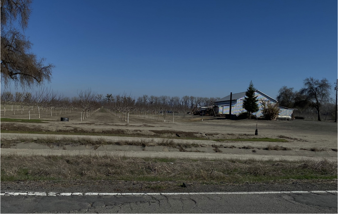
Photo 6: View of Dunnigan Pipeline alignment looking west from State Route 45 (Alternative 2)
