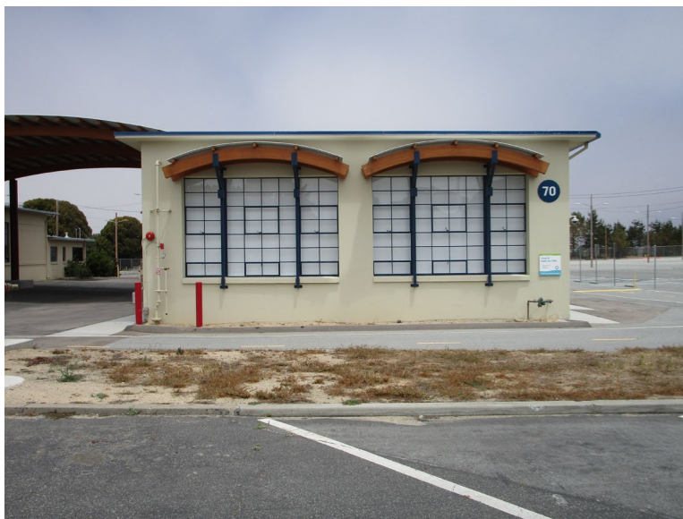
Figure 1. Main (south) elevation, looking north (IMG_0335)
