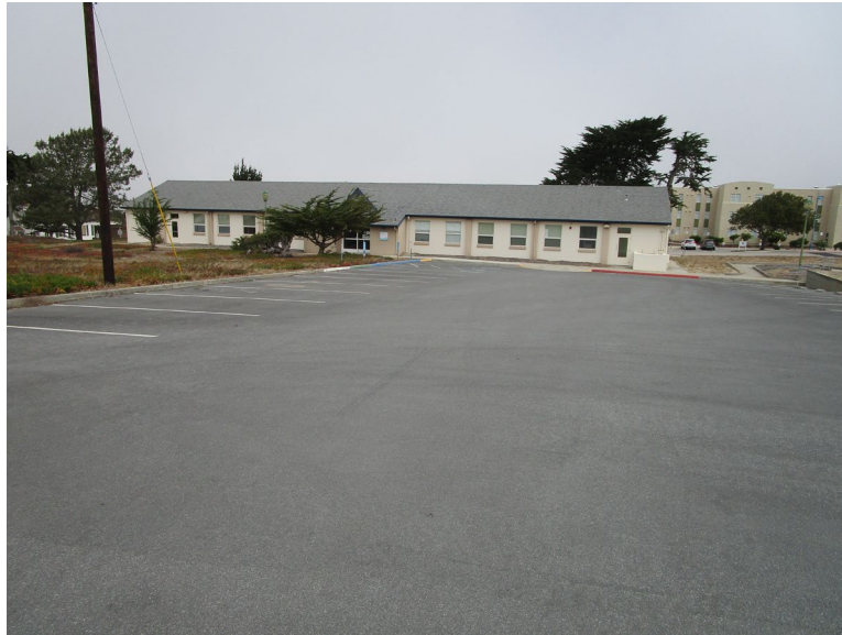
Figure 1. Main (south) elevation, looking north (IMG_0292)
