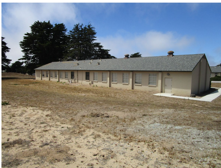
Figure 2. South elevation, looking northwest (IMG_0576)
