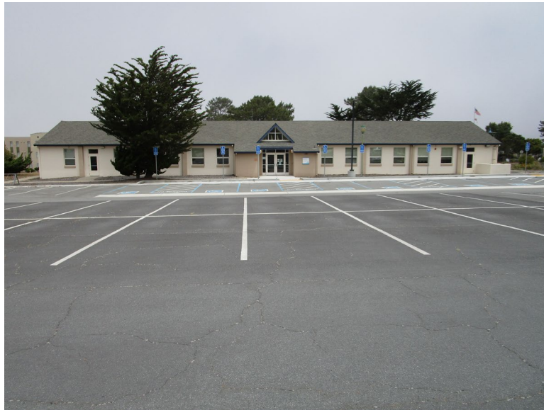
Figure 1. Main (south) elevation, looking north (IMG_0302)
