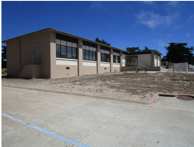
Figure 1. Main (west) elevation and north elevation, looking southeast (IMG_0604)
