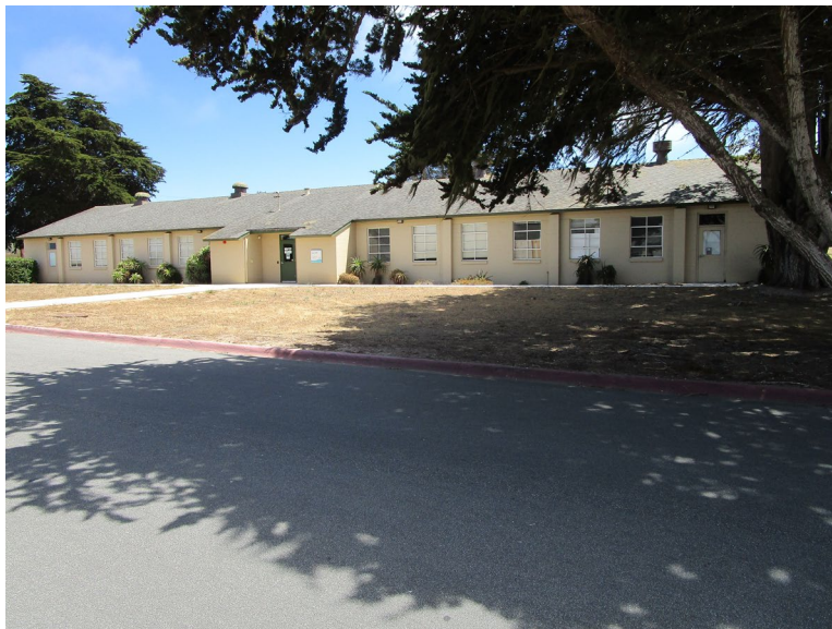
Figure 1. Main (north) elevation, looking southeast (IMG_0566)
