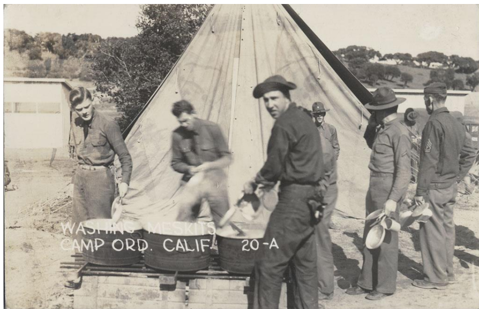
Figure 3. Impermanent, temporary tents and buildings at Fort Ord c. 1939 (CSUMB 2021: Image 121).
