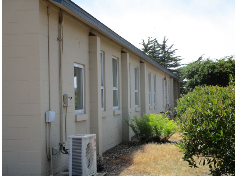
Figure 2. north elevation, looking southwest (IMG_0598)
