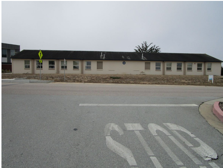
Figure 2. North elevation, looking south (IMG_0314)
