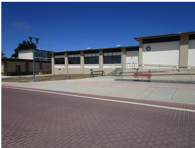
Figure 2. Main (west) elevation, looking northeast (IMG_0654)
