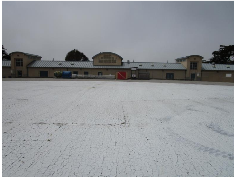
Figure 2. East elevation, looking west (IMG_0477)
