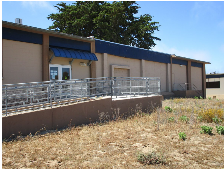
Figure 2. East elevation, rear entrance, awning, and filled in area that originally connected to the multi-story wing, looking northwest. (IMG_0639)
