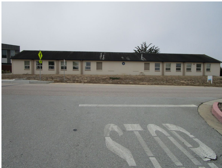
Figure 2. North elevation, looking south (IMG_0314)
