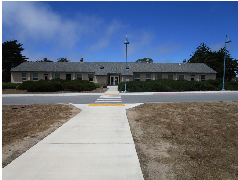
Figure 1. Main (south) elevation, looking north (IMG_0581)
