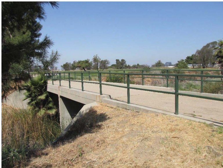
Figure 20. Bridge 1, view to northwest, Image No. IMG_5524.
