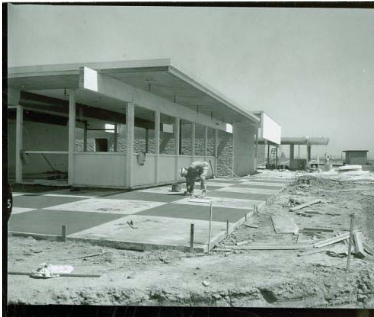
Figure 7. Rear (Southwest) Elevation of the Clubhouse Under Construction, 1966 (COLAPL 1966c)
