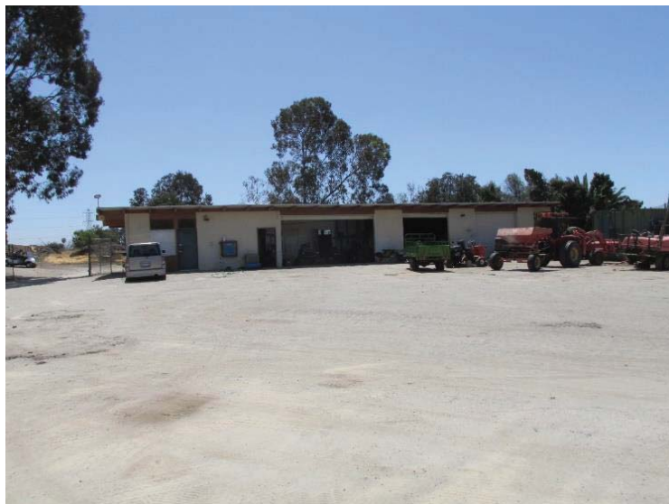
Figure 18. Outbuilding 1 Northwest Elevation, view to southwest, Image No. IMG_5768.
