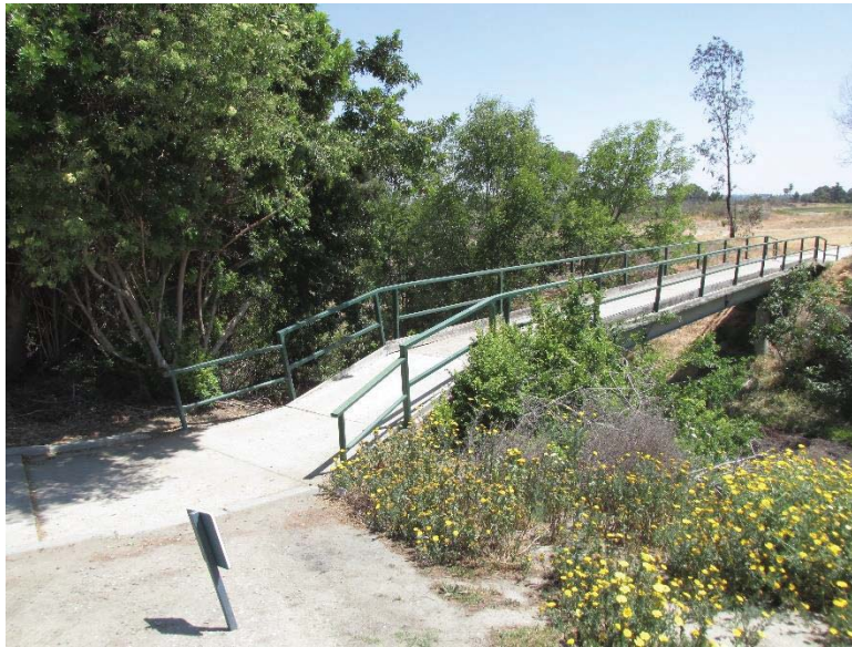
Figure 21. Bridge 2, view to northeast, Image No. IMG_5649.
