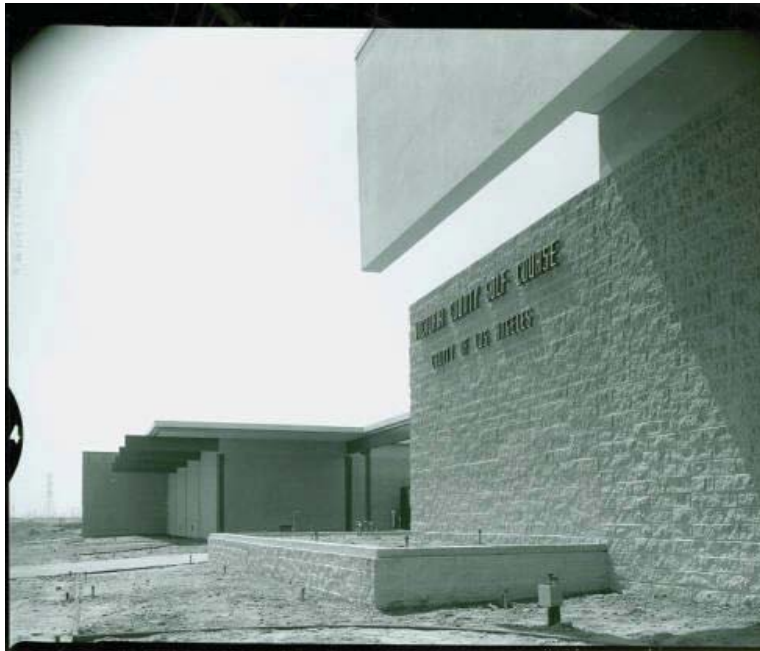
Figure 6. Clubhouse Façade (Northeast Elevation), 1966 (COLAPL 1966b)
