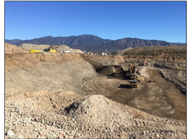
Photograph 3 - View of one of the active quarry pits, facing northwest.
