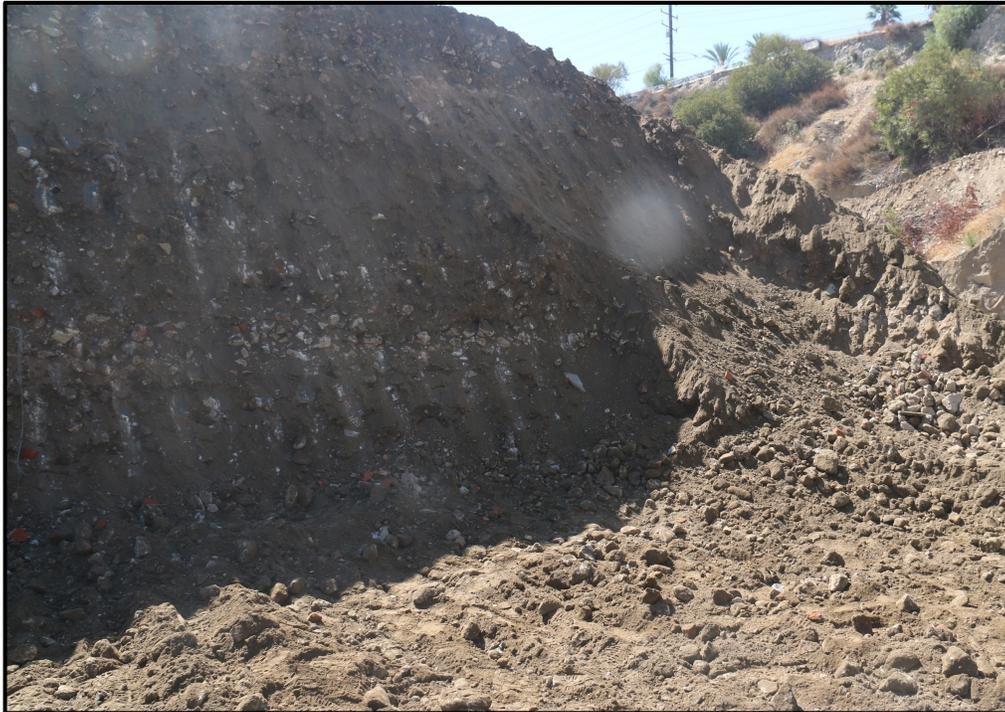
**2017 April** – Southeast Pit (Area 3S). Face of new engineered fill slope cleaned of slough. View to southeast.
