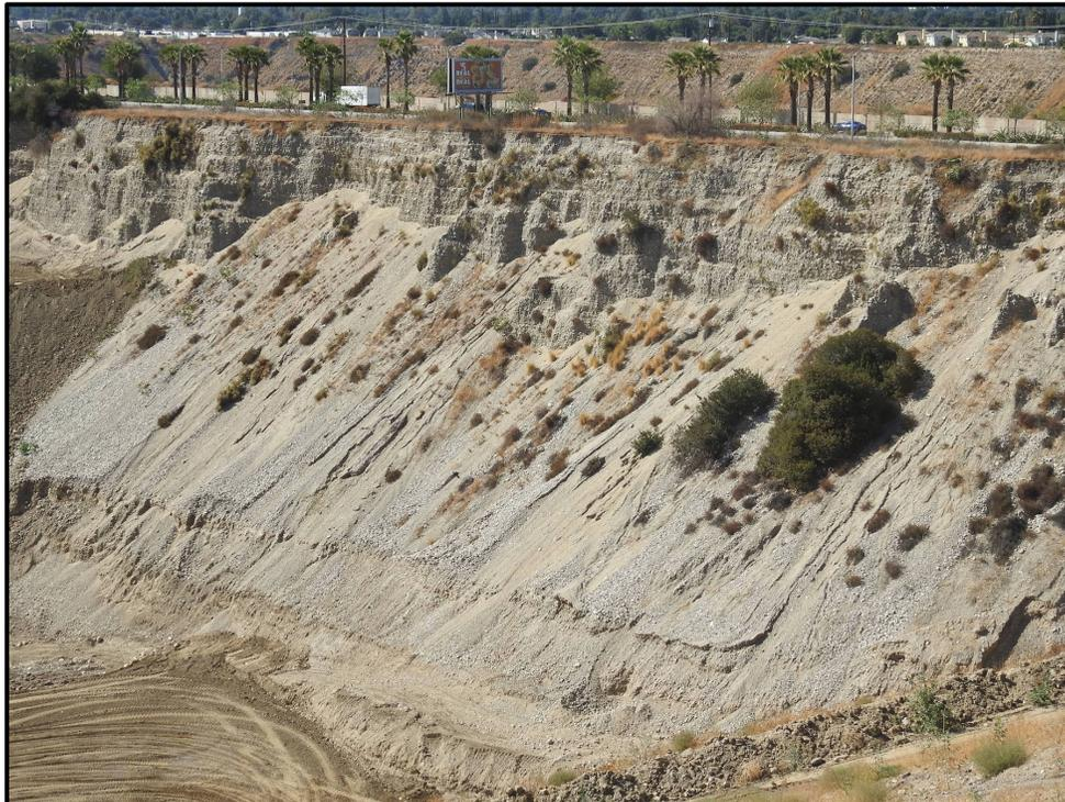
**2017 September** – West Pit (Area 1). Overview of north side wall. Veneer of talus material covering lower (diagonally-inclined) portion of slope. View to northwest.
