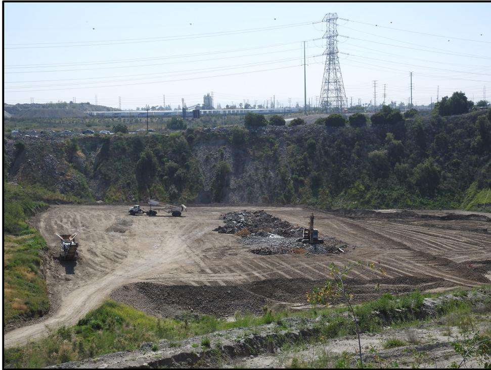
**2017 April** – Southeast Pit (Area 3S). Truck discharging inert debris and pulverization of oversized material. View to east; I-605 Freeway in background.
