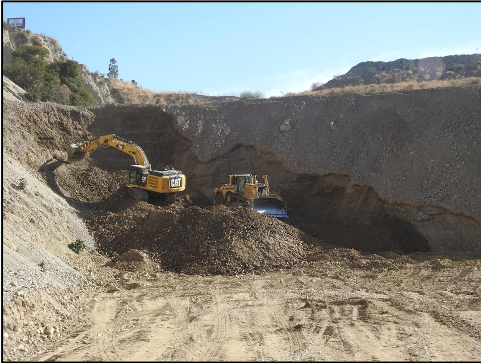
**2018 February** – West Pit (Area 1). Removals of sloughed material at slope face and exposing new engineered fill. View to east.
