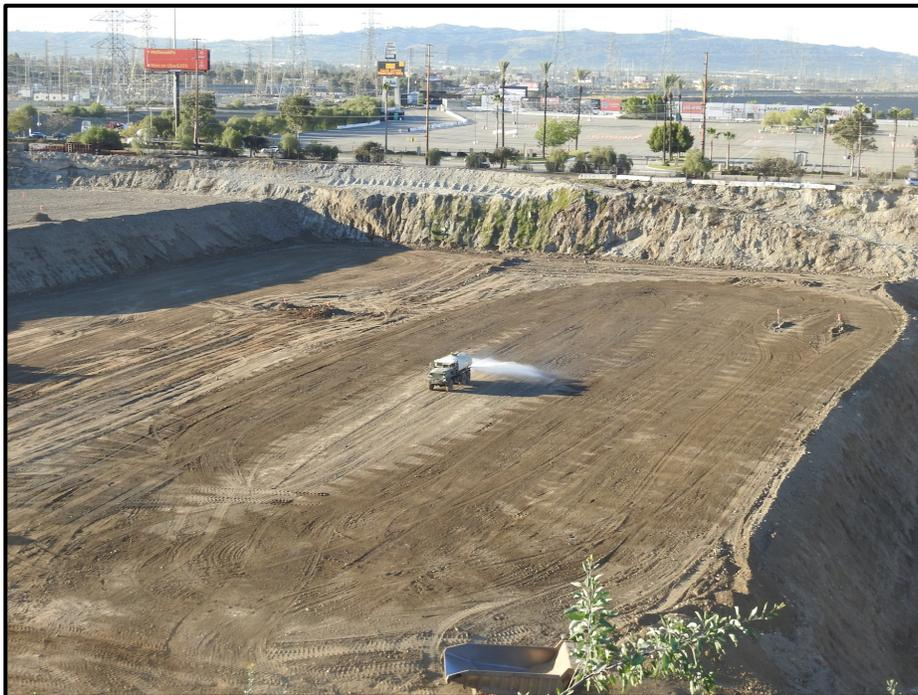
**2018 March** – Southeast Pit (Area 3S). Overview of engineered fill. Settlement monument cluster at background-right of water truck (SM301, SM308), at background-left of water truck (SM300, SM310), and SM307 is at far left on next bench up. View to southeast.
