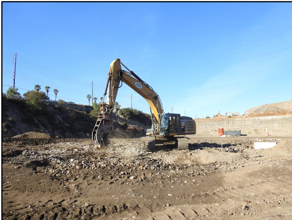
**2017 November** – Southeast Pit (Area 3S). Pulverization of oversized inert debris material. Settlement monument SM300 at right. New settlement monument SM310 with exposed base at far right. View to southwest.
