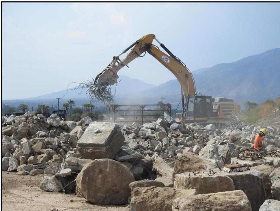
**2018 January** – South-Central Area (Area 2S). Removal of steel from inert debris. Large-scale field sieve in background. View to west.
