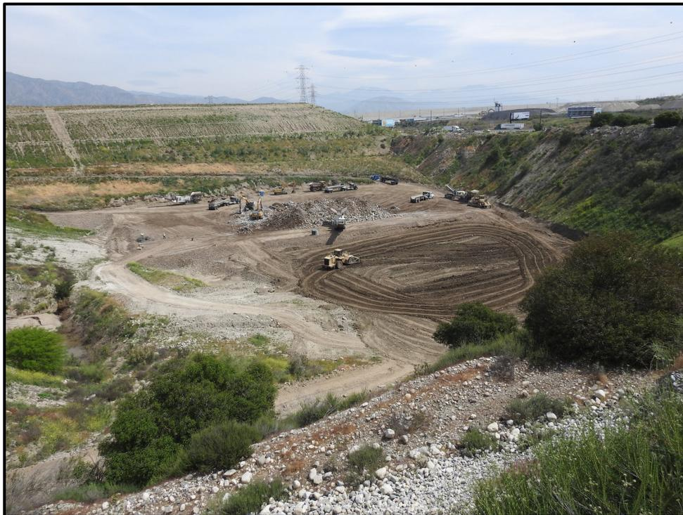
**2017 April** – Southeast Pit (Area 3S). Compaction of blended rubble fill. Area 3N surcharge fill in background. View to northeast.
