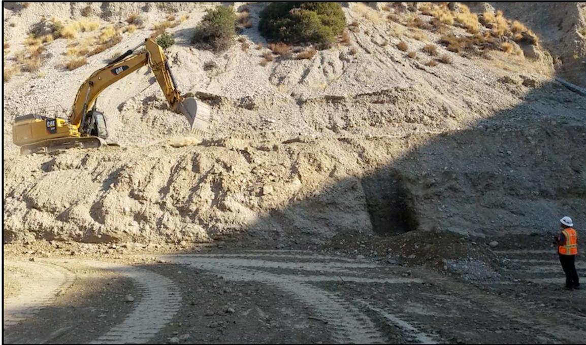
**2017 September** – West Pit (Area 1). Geologic evaluation of side wall materials by means of excavated pits. View to north.
