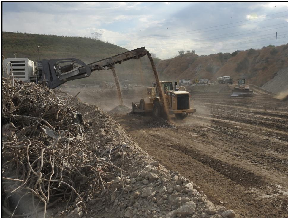
**2017 August** – Southeast Pit (Area 3S). Crushing of pulverized inert debris, and compaction of blended rubble fill. View to northeast.
