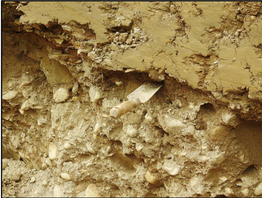
**2017 August** – West Pit (Area 1). Geologic characterization of West Pit bottom materials. Trowel is stuck into side wall at contact of previously-placed silt and clay wash products and the underlying native sands and gravels. The wash products were removed in preparation for placement of engineered fill.
