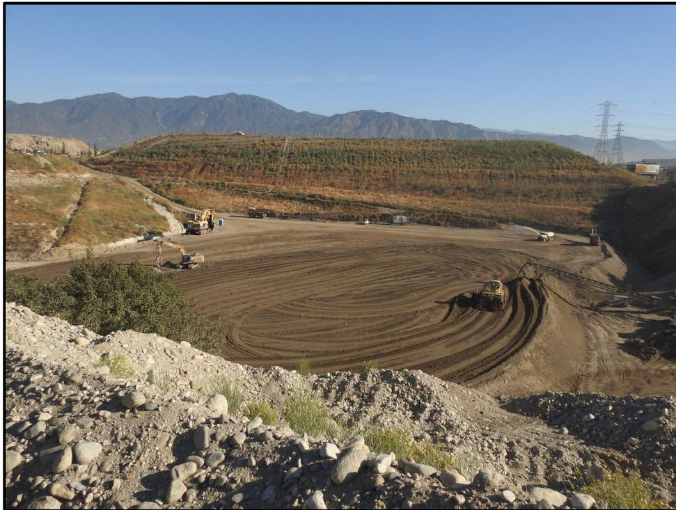
**2017 September** – Southeast Pit (Area 3S). Engineered fill pad, Area 3N surcharge fill in background, and Zone A material at background-left. View to north.
