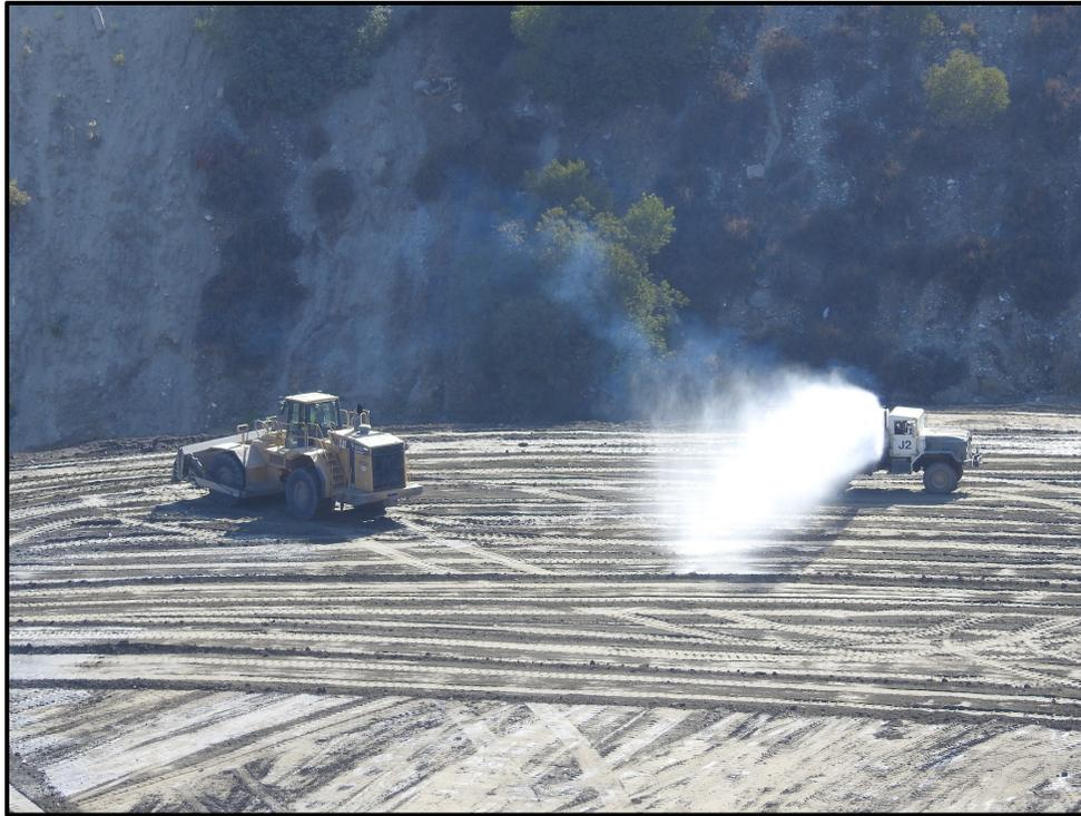
**2017 October** – Southeast Pit (Area 3S). Moisture conditioning and compaction at engineered fill pad. View to southeast.
