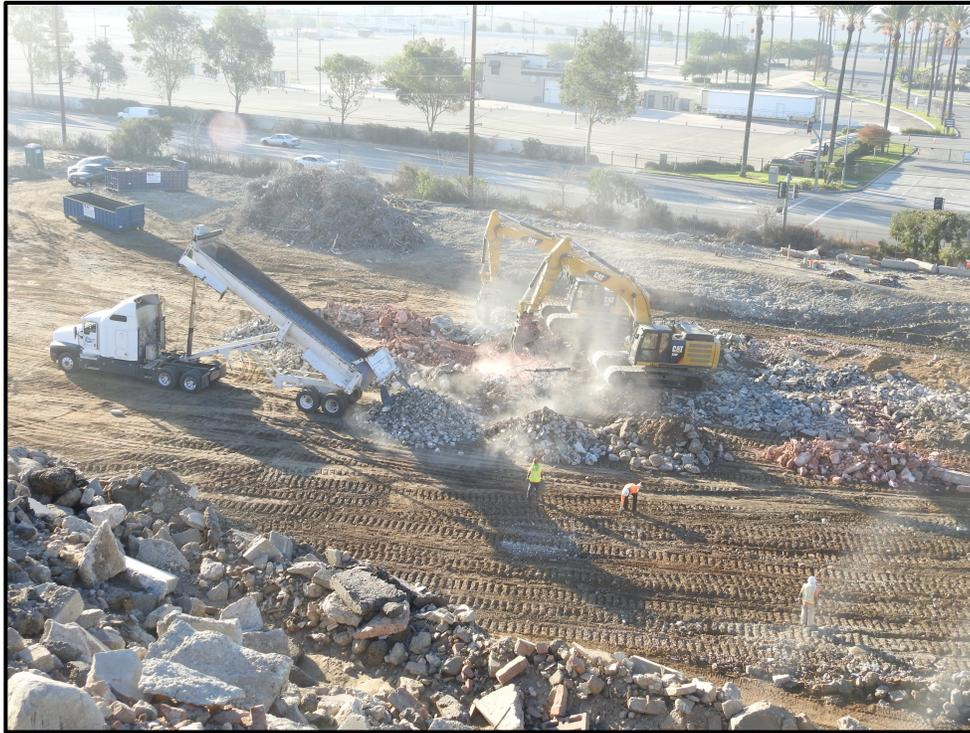
**2018 January** – South-Central Area (Area 2S). Truck discharging inert debris to be processed and placed. At right, pulverization in advance of crushing. Stockpiling of extracted steel in background. View to southeast.
