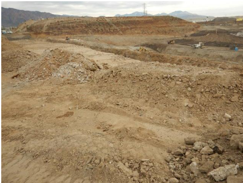
Photograph No. 4: Staging Area foreground, surcharge stockpile in background - view NE
