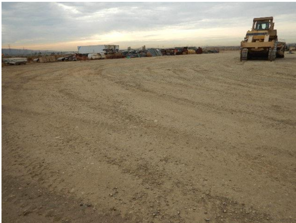
Photograph No. 10: Staged equipment on top of surcharge fill – view WSW
