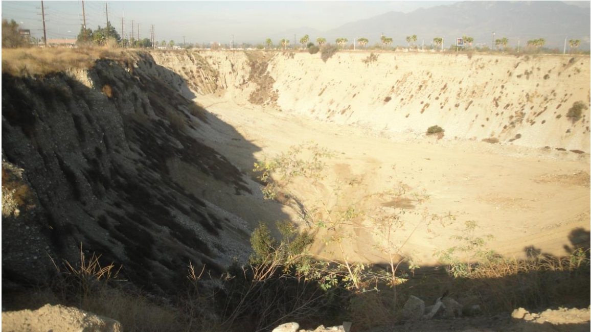
Photograph No. 11: West quarry excavation after clearing and grubbing – view NW
