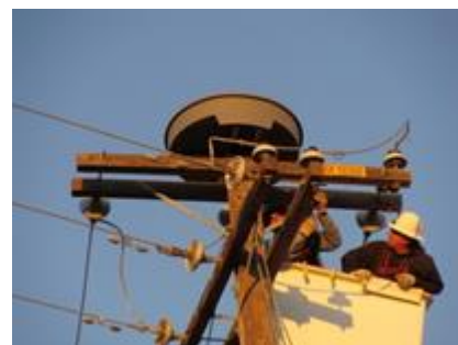
Installation of Osprey Nesting Platform
