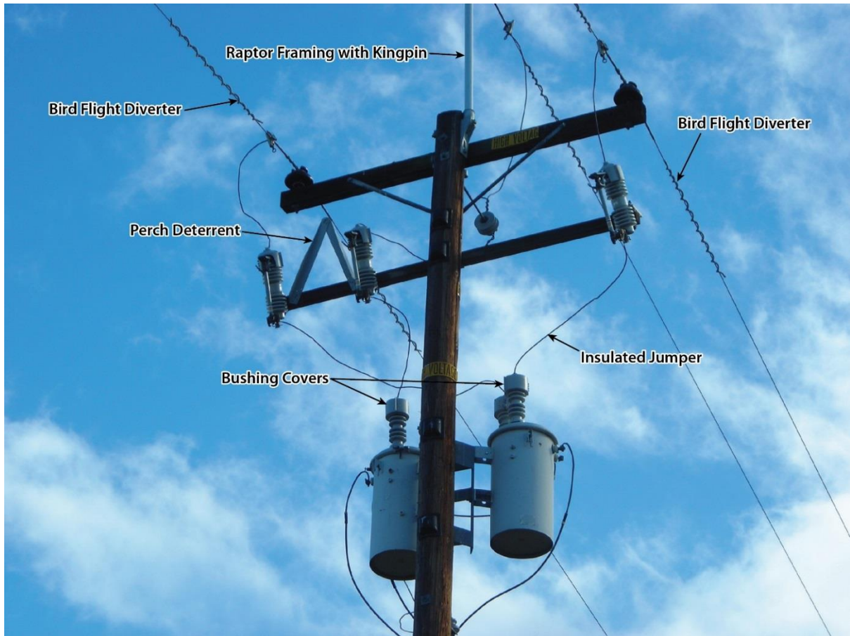
Figure 3. Important Avian Protection Hardware on Electric Facilities
