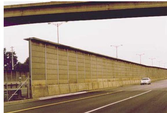
**Figure 25. T-profile top barrier**
