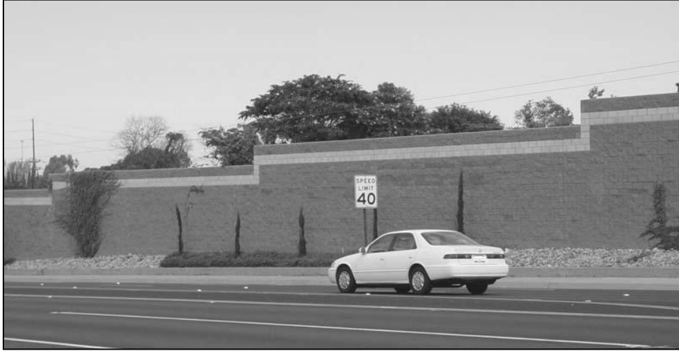
Sound attenuation walls and limits on speed help to shield residential neighborhoods from automobile noise on Imperial Highway.
