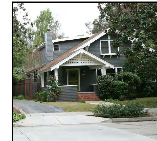
EXISTING KELLOGG HOUSE
