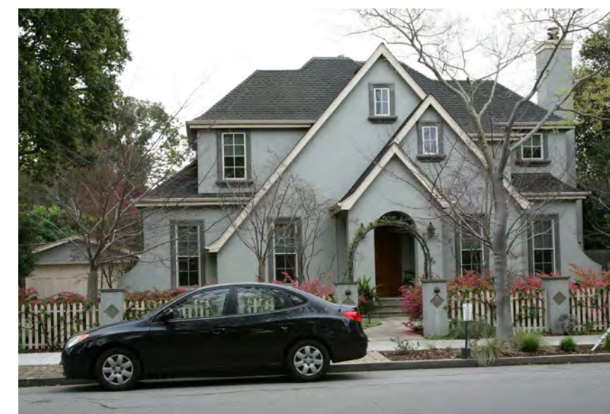
EXISTING EMERSON HOUSE
