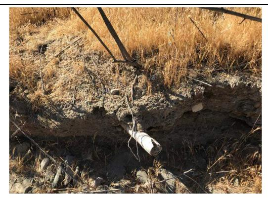
Photo 19: Additional PVC pipe entering into the Bouquet Creek riverbed.
