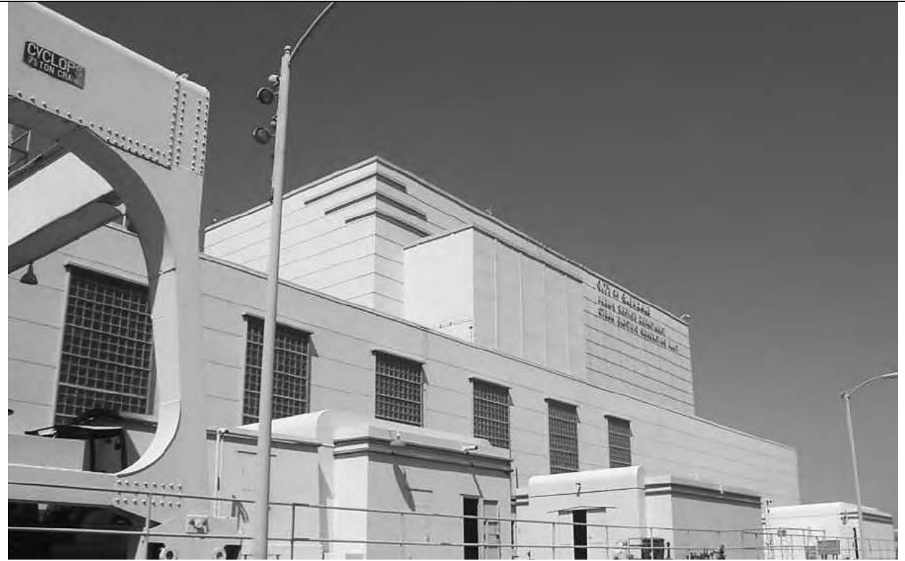
Figure 3: Excerpted, cropped photograph from Initial Study, Architectural Resource Evaluation of The Grayson Power Plant For City of Glendale, California, Figure 18 (page 6.6). View is of the northwest, main façade, no date (estimated 2016). Note the staggered green horizontal bands at the left corner of the tower, the sign at the right side, sets of multi-story, glass block windows of the boiler portion of the building, original, riveted “Cyclops” crane at left foreground and Units 3, 2 and 1 (left-to-right) in the foreground. The turbine covers for Units 1-3 have radiused roof-wall connections on the main volumes at each endwall, modulating the appearances of otherwise entirely utilitarian structures. Double fillet bands wrap around their lower cornices and corners, emphasizing the carefully expressed scale and proportion.
