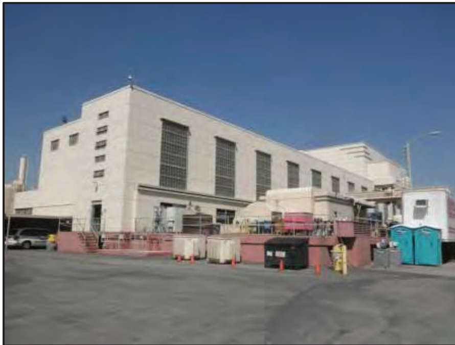
Photograph 3. Grayson Boiler Building, View Looking Northwest (Photo by J. Terry).
