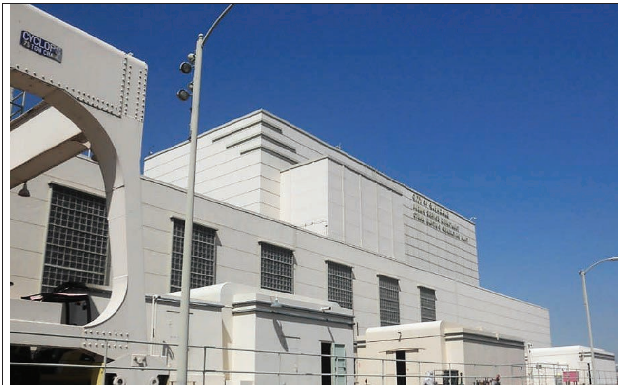
Figure 3: Excerpted, cropped photograph from Initial Study, Architectural Resource Evaluation of The Grayson Power Plant For City of Glendale, California, Figure 18 (page 6.6). View is of the northwest, main façade, no date (estimated 2016). Note the staggered green horizontal bands at the left corner, the sign at the right side, sets of multi-story glass block windows of the boiler portion of the building, original, riveted “Cyclops” crane at left foreground and Units 3, 2 and 1 (left-to-right) in the foreground. The turbine covers for Units 1-3 have radiused roof-wall connections on the main volumes at each endwall, modulating the appearances of otherwise entirely utilitarian structures. Double fillet bands wrap around their lower cornices and corners, emphasizing the carefully expressed scale and proportion.
