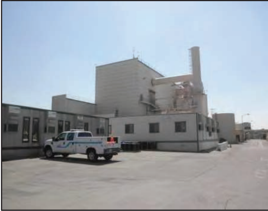
Photograph 4. Grayson Boiler Building, View Looking Southwest (Photo by J. Terry).
