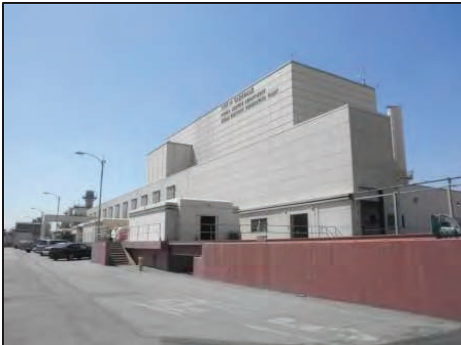
Photograph 5. Grayson Boiler Building, View Looking Southeast (Photo by J. Terry).
