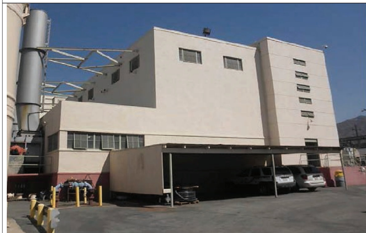
Figure 5: Excerpt from Initial Study, Architectural Resource Evaluation Of The Grayson Power Plant For City of Glendale, California, undated photograph estimated 2016,(Figure 26 Grayson Boiler Building page 6.10, same view as Figure 4 above). Note all visible awning-type, steel sash windows, exterior materials, the building configuration and Stripped Classicist design remain recognizable. Carport at lower center is an addition (year unknown). Note the stucco scoring bands at the right-hand boiler building tower and the dimensioned continuous sill and header on the left-hand bank of ribbon windows that enunciate the endwalls, providing visual interest and relief. Other than the carport, no alterations are visible.
