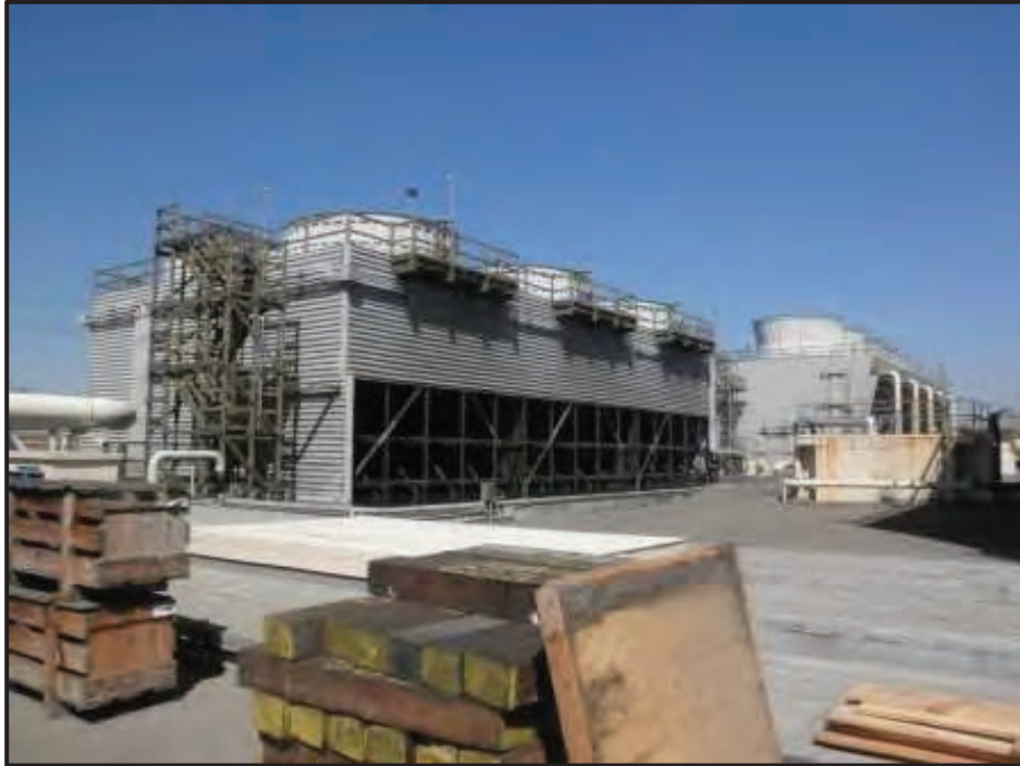
Photograph 13. Cooling Tower No. 3 (No. 5 in Background), View Looking Northwest (Photo by J. Terry).
