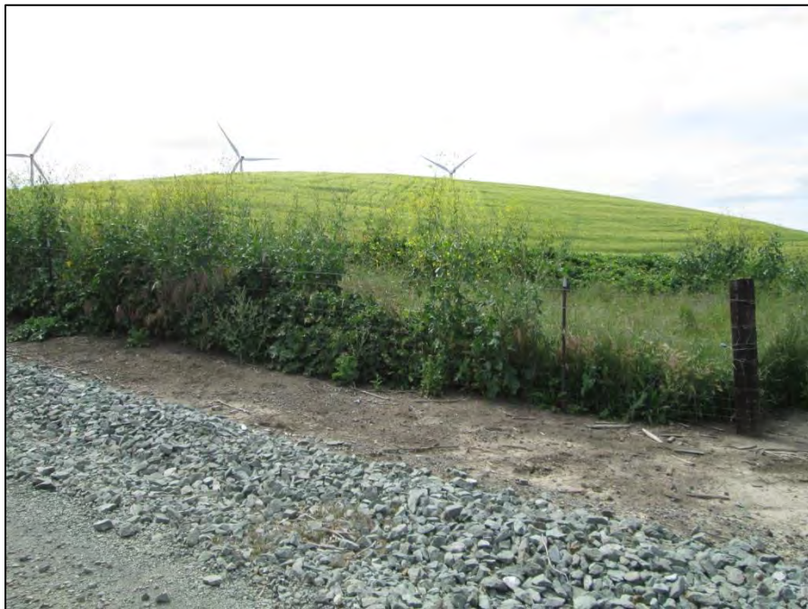
Photo 4. Invasive weeds growing along fence-line behind Operations and Maintenance building. April 25, 2017.
