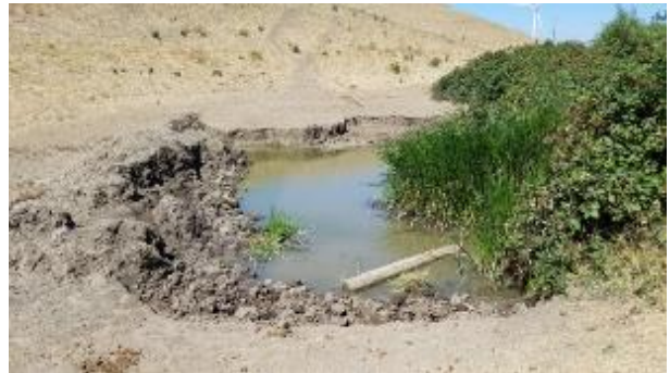
Photograph 10. Feature 52 is perennially ponded, but the relative isolation of the feature reduces the likelihood of CRLF predators, increasing its suitability for CRLF aquatic breeding habitat (facing southwest).
