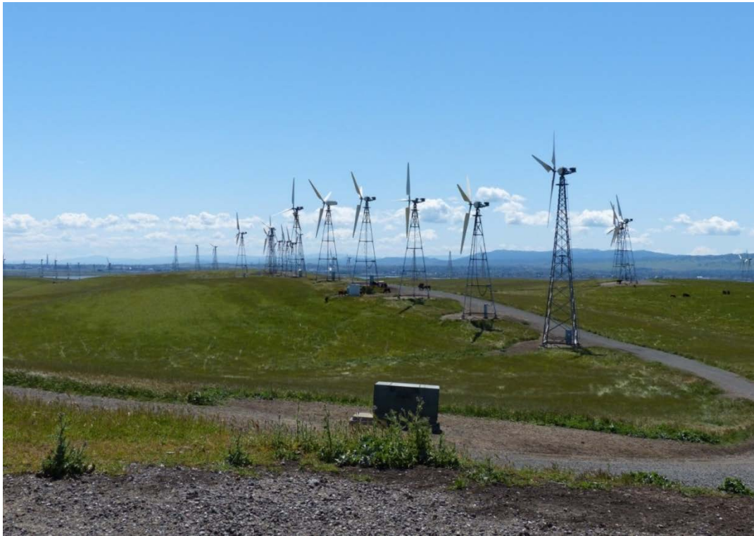
Exhibit 2-3 Former Wind Turbine Generators, Solano 4 West
