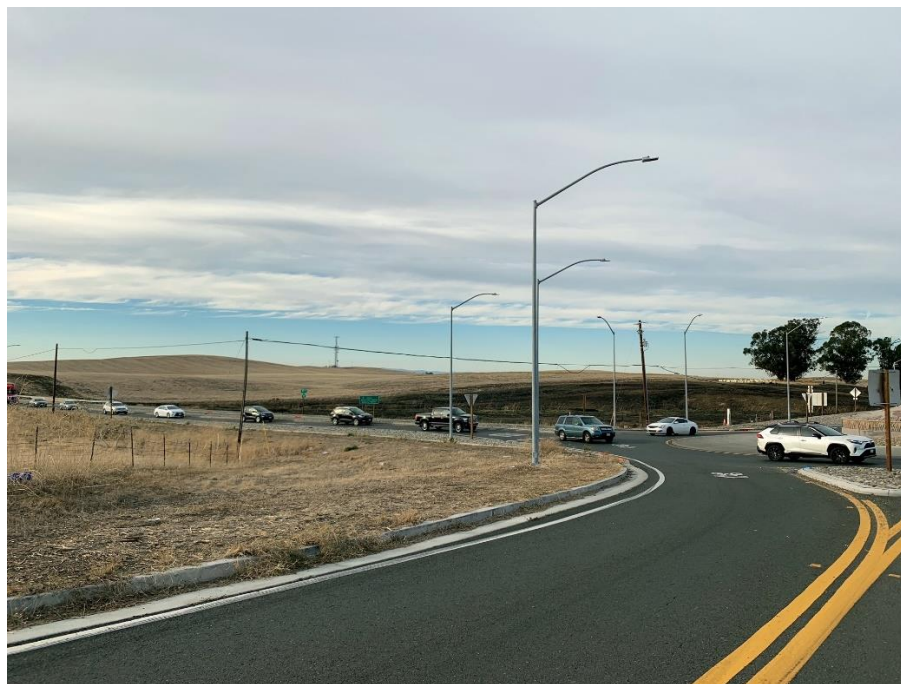
Photo 12. Photo facing northwest (38.1837, -121.8061) depicting the roundabout intersection of State Route 12, Bird's Landing Road (AECOM 2022).
