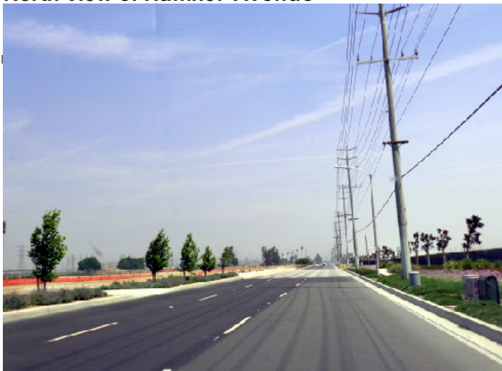
North View of Hamner Avenue
