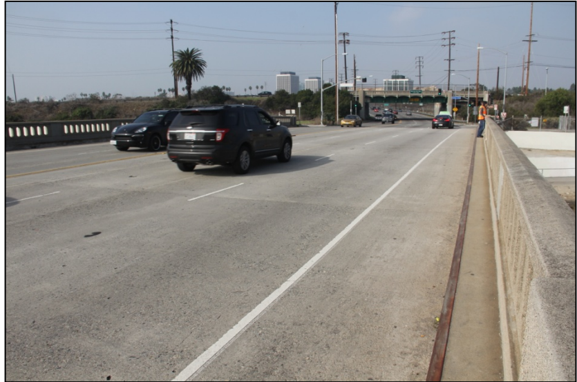
Photo 2. Existing Lincoln Boulevard Bridge over the Ballona Creek
