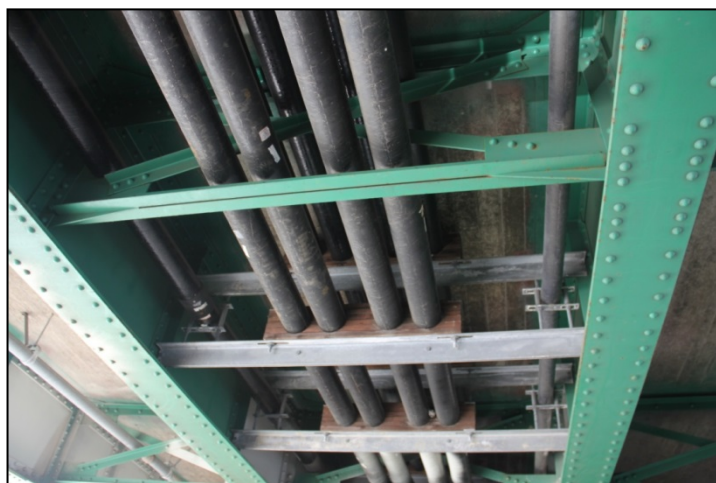
Photos 5 & 6: Utility lines under the existing Lincoln Boulevard Bridge and Culver Boulevard Overcrossing
