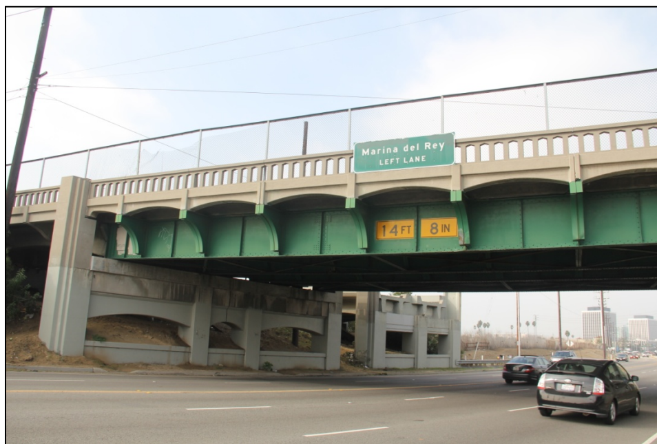
Photo 4. Existing Culver Boulevard Overcrossing
