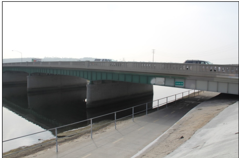
Photo 3. Existing Ballona Creek Bicycle Path
