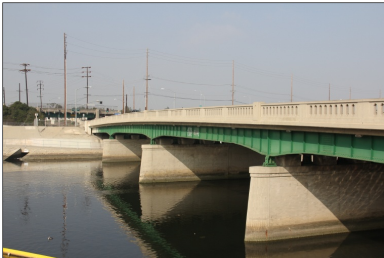
Photo 1. Existing Lincoln Boulevard Bridge over Ballona Creek
