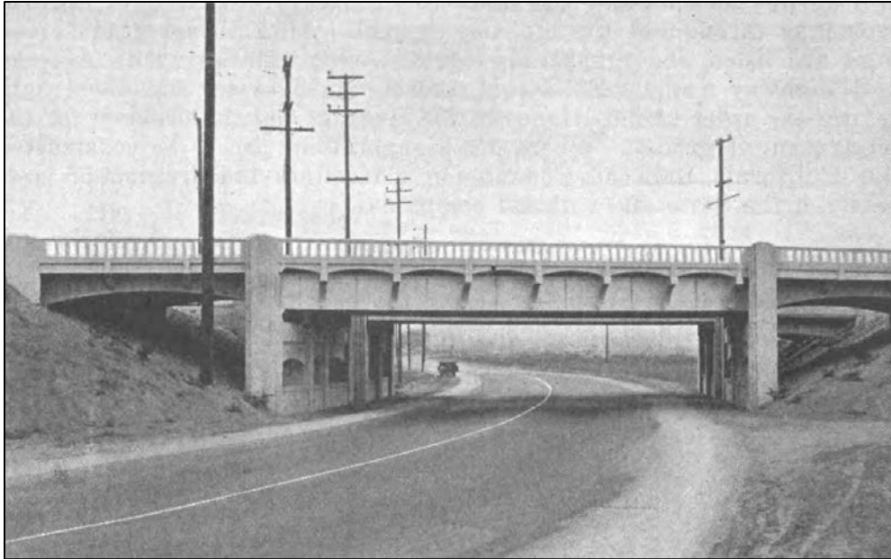
Photograph 5. Photograph of the completed grade separation looking north at Culver Boulevard overcrossing. A portion of the Pacific Electric Railway Bridge over SR 1 is behind the bridge depicted in this photograph. 46
