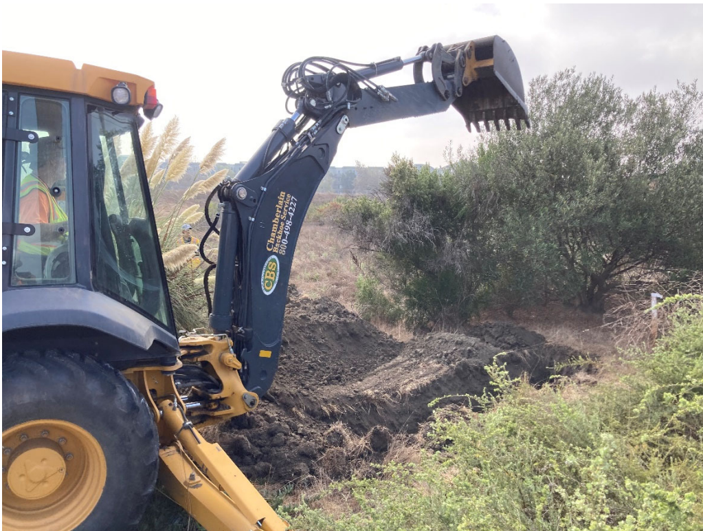
Figure 2: Chamberlain Backhoe Operator Excavating Proposed Trench
