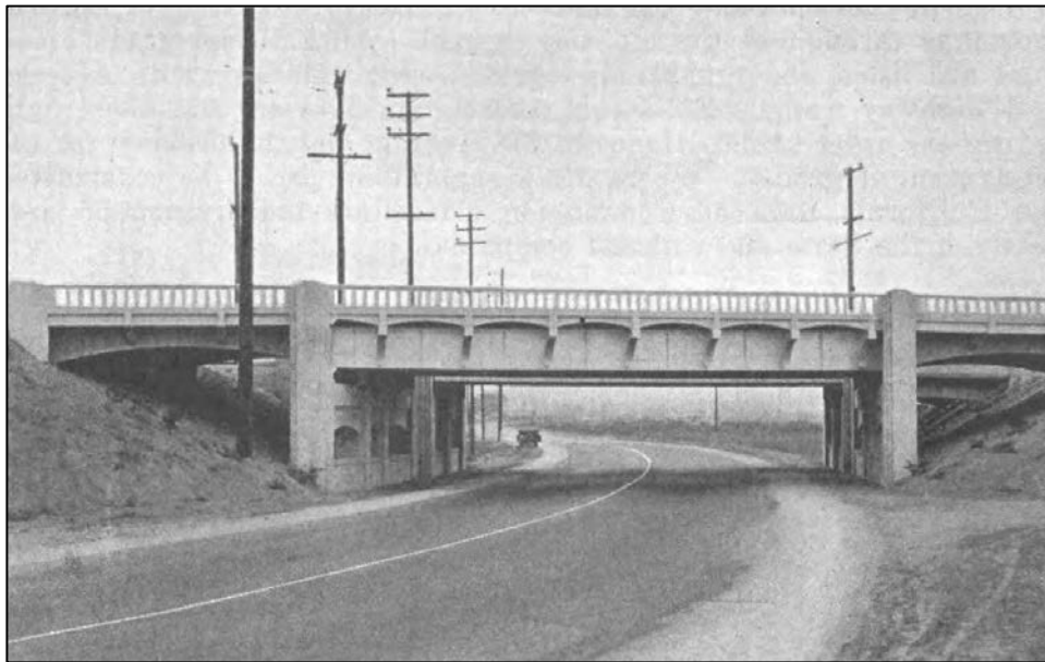
Image 2. Photograph of the completed grade separation looking north at Culver Boulevard overcrossing. A portion of the Pacific Electric Railway Bridge over SR 1 is visible behind the bridge depicted in this photograph. 24
