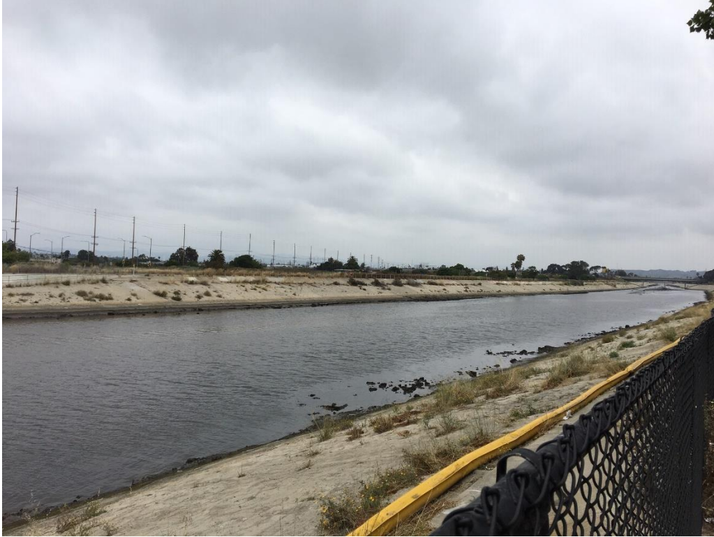
Figure 5: Ballona Creek (View Towards Northeast)
