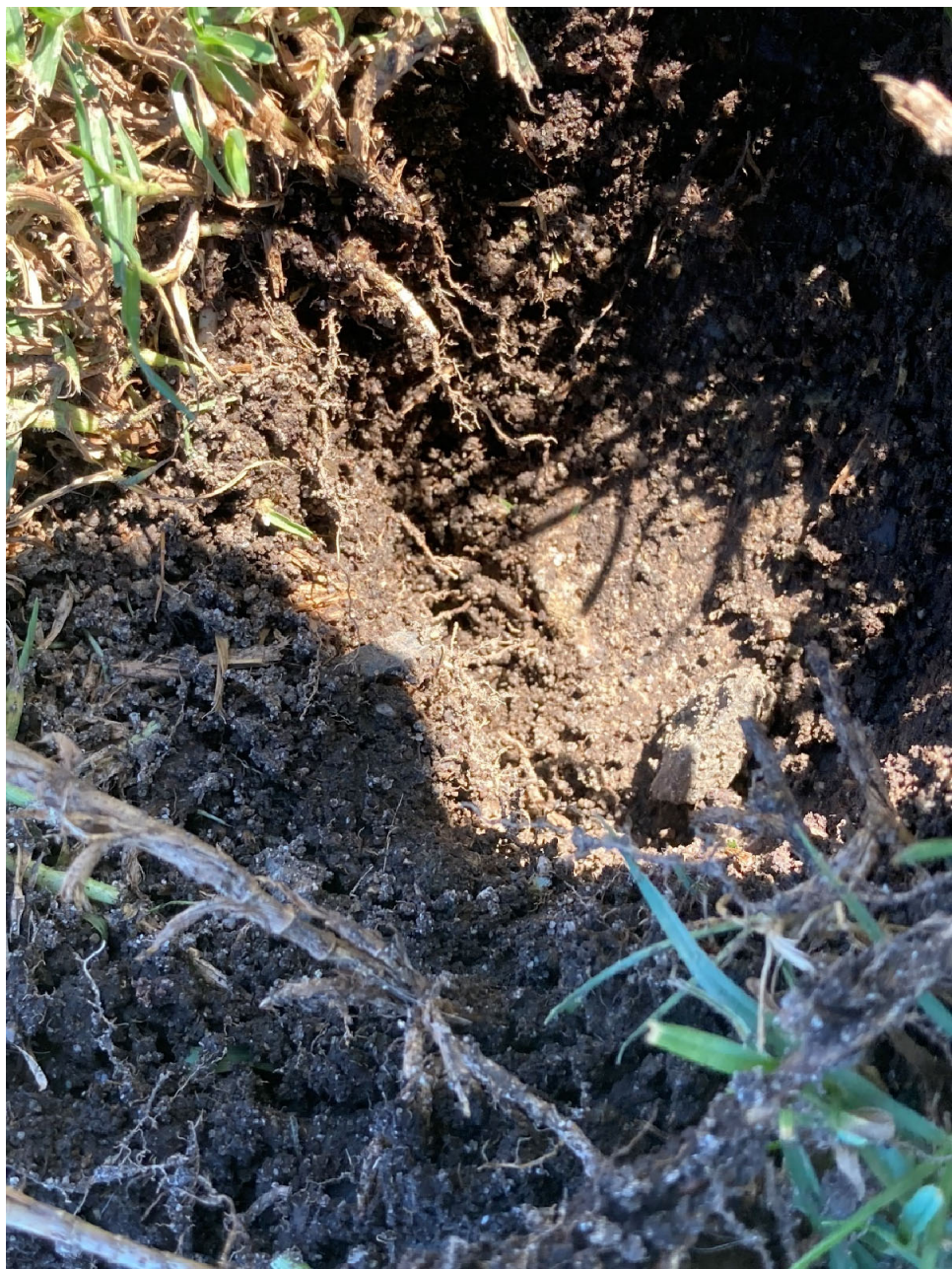
Figure 11: Cement/Asphalt Identified at 7 Inches Below Surface
