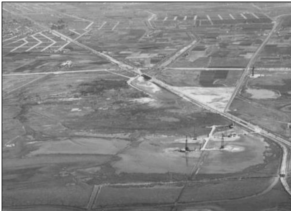
Image 1. 1933 photograph camera facing east show the incomplete Ballona Creek Channel. Grading for SR 1 has just been completed horizontally left to right. Angled road is Culver Boulevard. 22
