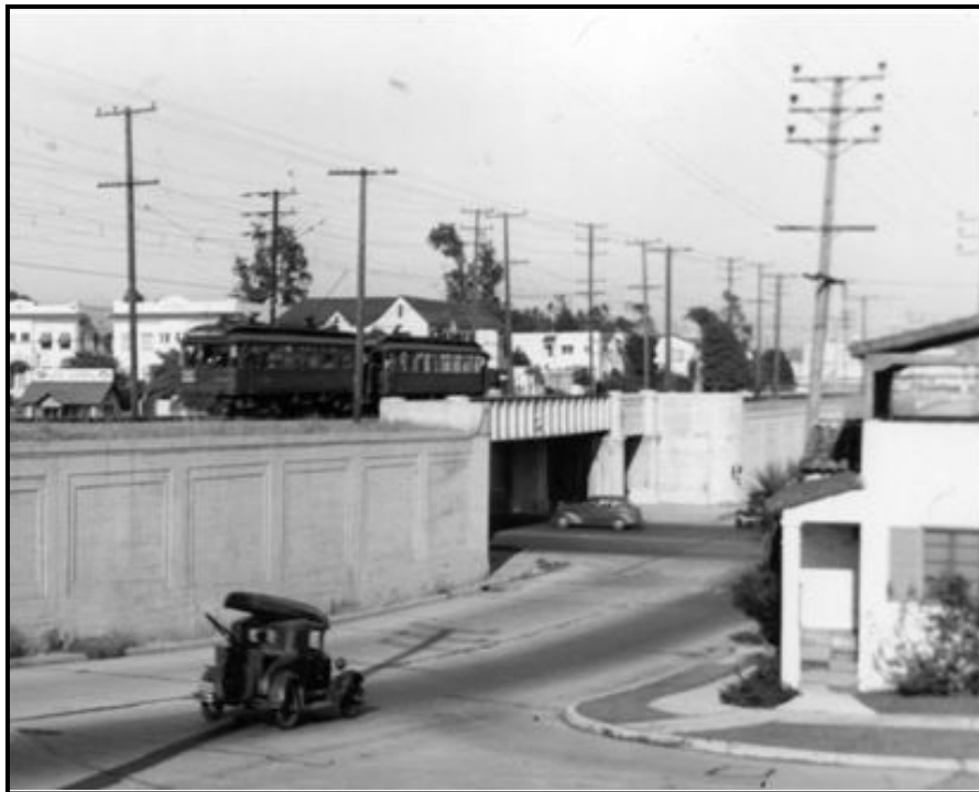
The Pacific Electric Railway crossing over La Brea Avenue in Los Angeles. The bridge has concrete abutments extending from a raised railbed. (Photograph courtesy of the Craig Rasmussen Collection, http://www.pacificelectric.org )
