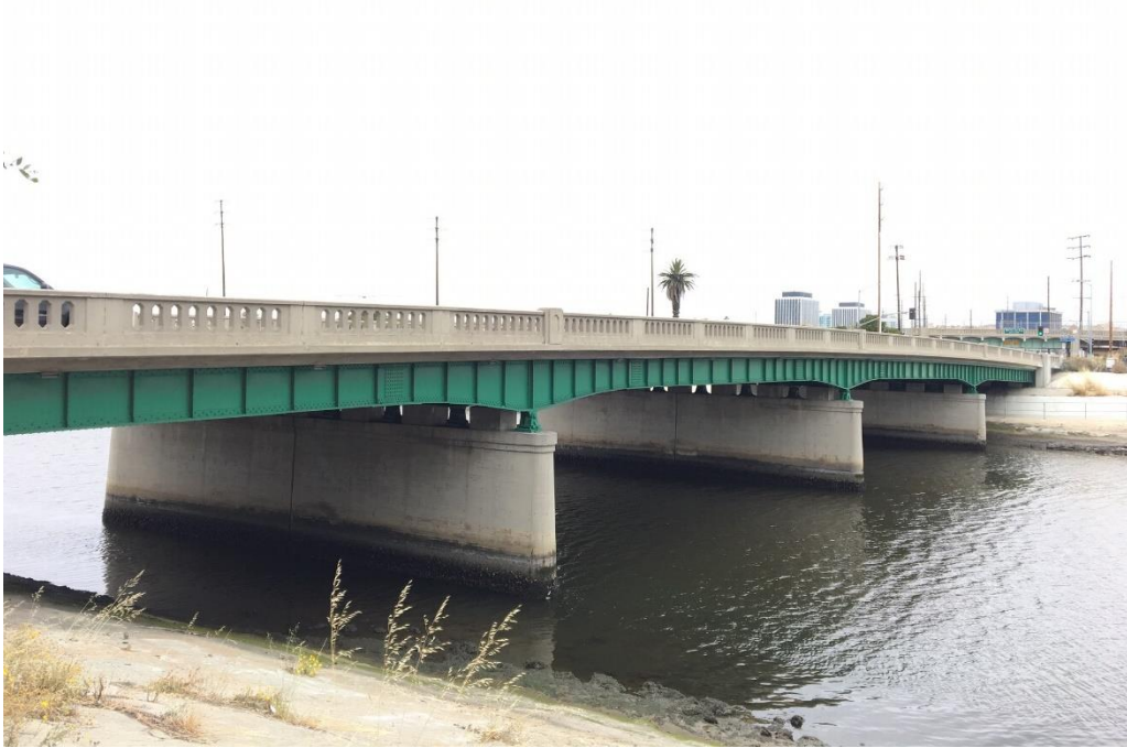
Figure 3: P-19-176734 Ballona Creek Bridge (View Towards Northwest)
