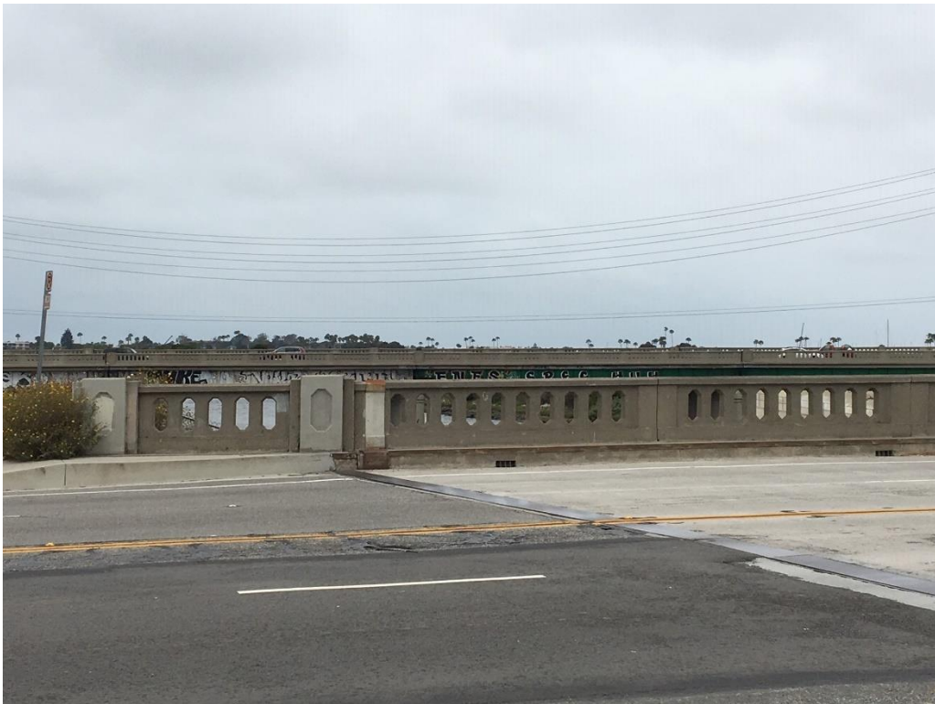
Figure 4: P-19-176734 Ballona Creek Bridge (View Towards West)
