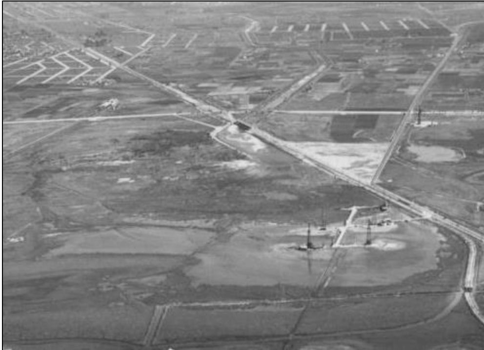
Photograph 4. 1933 photograph camera facing east show the incomplete Ballona Creek Channel. Grading for SR 1 has just been completed horizontally left to right. Angled road is Culver Boulevard. 45
