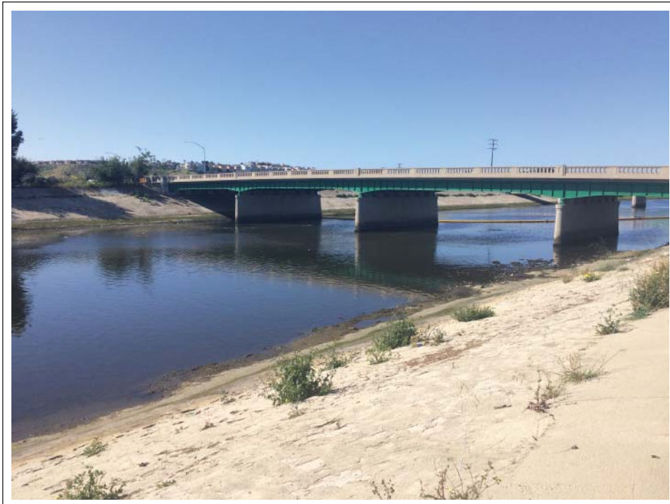
Northeast quadrant, looking west towards Lincoln Bridge.
