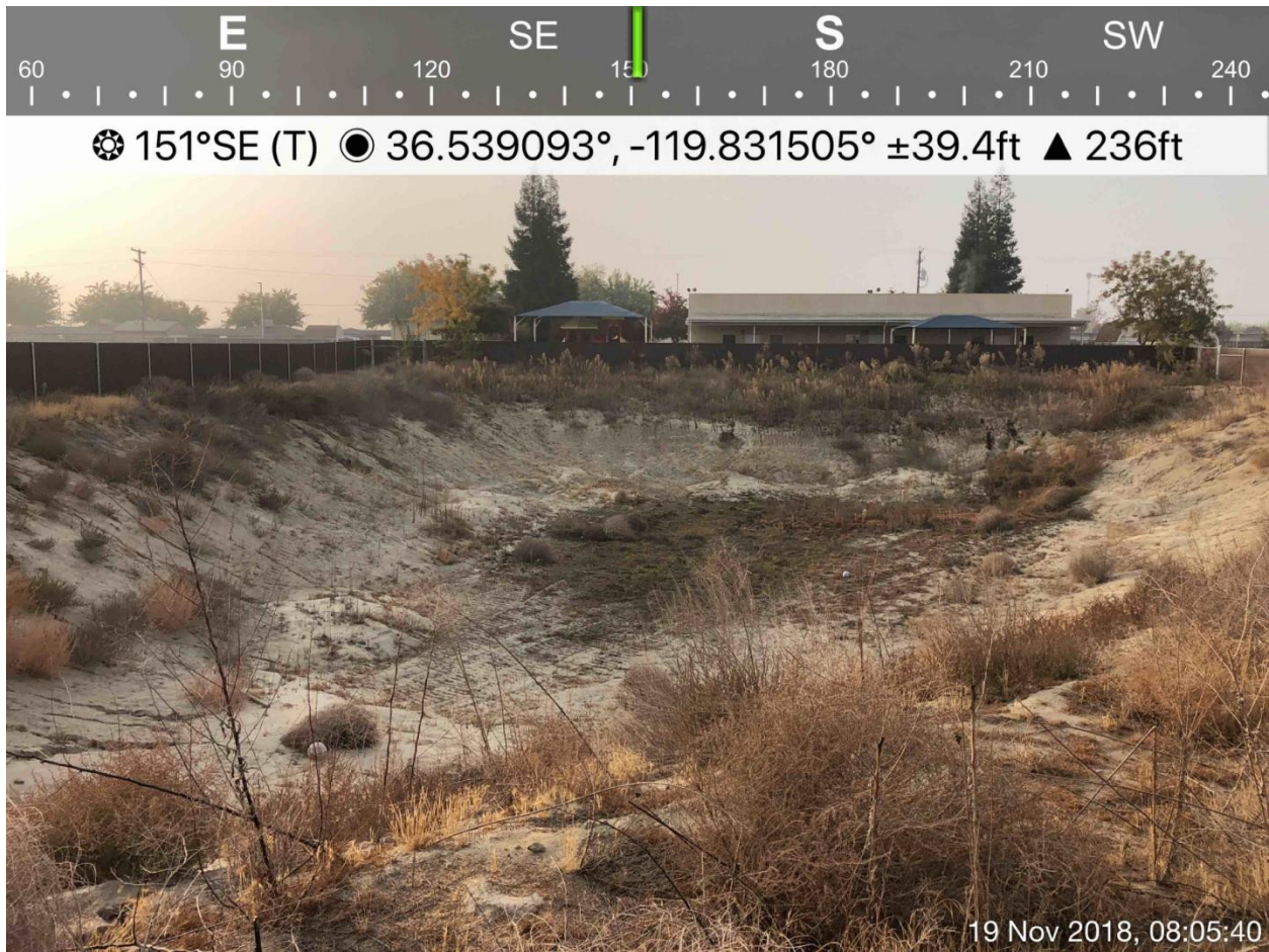
Photograph 26: Dry and ruderal ponding basin, enclosed with a slatted fence, adjacent to the elementary school campus. This ponding basin lies between Well No. 5 and Potential Connection No. 2, and is therefore outside of the area expected to be impacted by construction.
