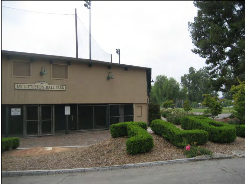
Photo 3: Jay Littleton Ballpark and other baseball fields are character-defining elements of the eastern portion of John Galvin Park.
