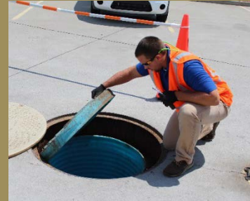
Inspecting a containment sump
