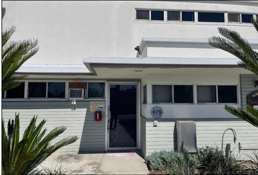
Photograph 2: Detail view of the main personnel entrance south façade of Fire Station No. 2. Note the brick cladding on the ground-level exterior. Camera facing north, October 14, 2021.
