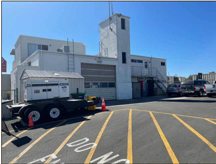
Photograph 6: Rear, north side of Fire Station No. 2. Camera facing southwest, October 14, 2021.
