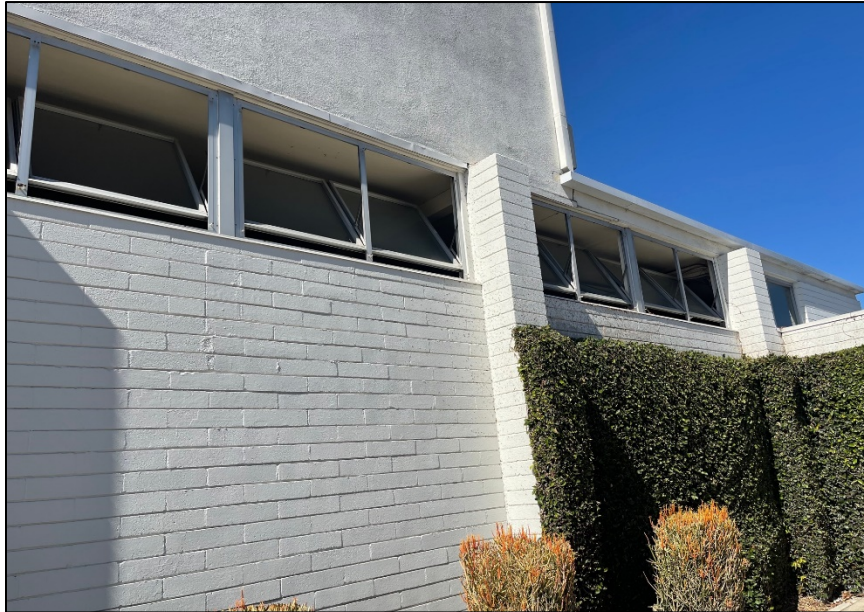
Photograph 4: Detail view of metal-sash hopper windows on the east side of Fire Station No. 2. Camera facing northwest, October 14, 2021.
