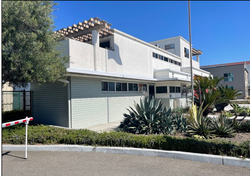
Photograph 5: Southwest corner of Fire Station No. 2, showing a portion of the west side. Camera facing northeast, October 14, 2021.
