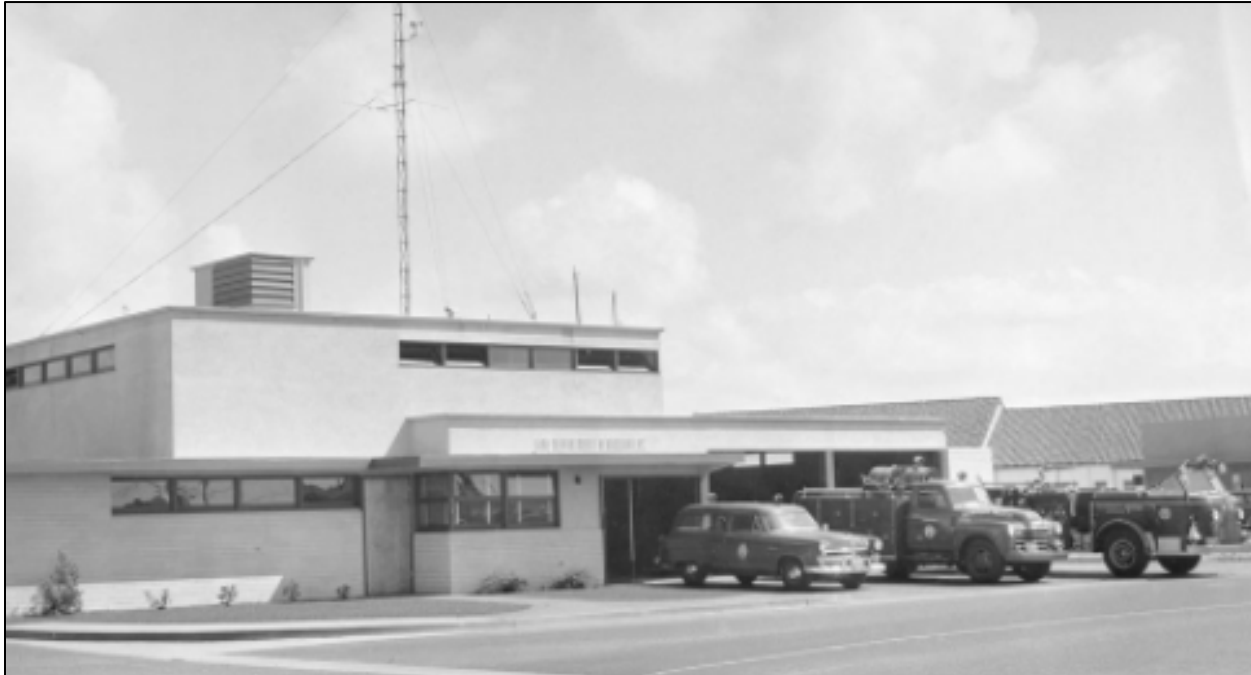
Figure 2: Undated photograph of Fire Station No. 2 showing appearance and fenestration arrangement subsequent to the construction of the first second-story addition in 1966 (Newport Beach Fire Department Archives n.d.).
