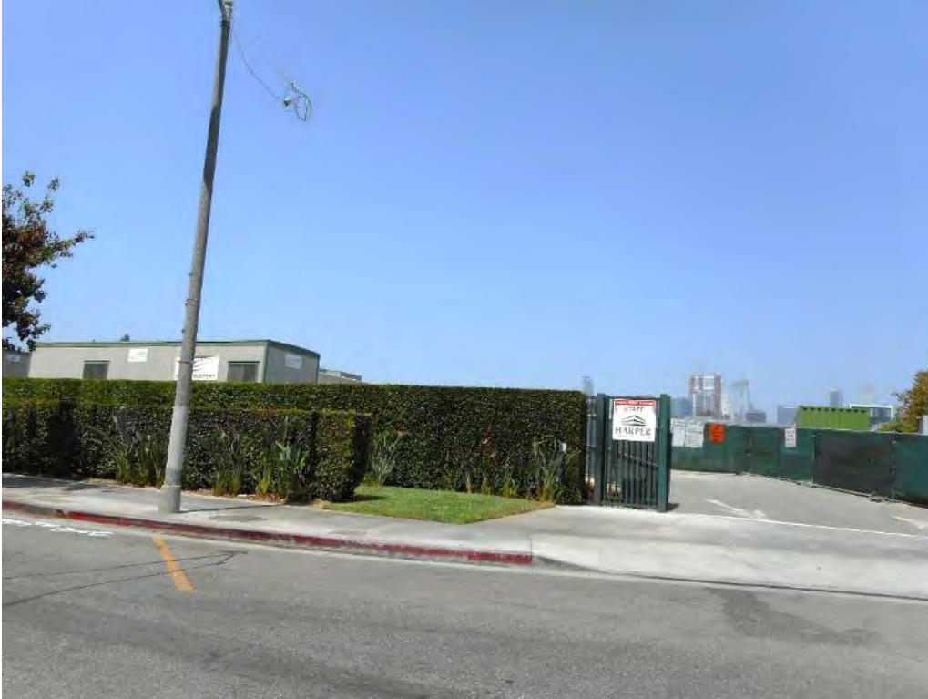
99. Construction area along 23 rd Street
