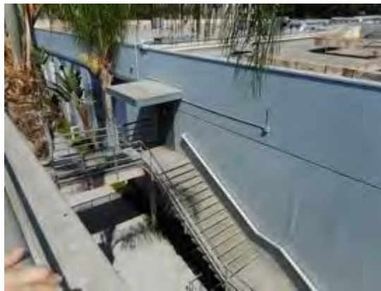
TBCSL/Redwood Hall west elevation with 1956 addition
