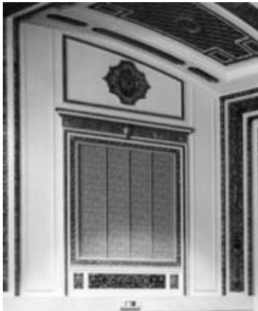
Detail of stage side wall c1978
