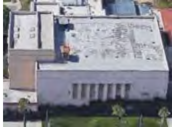
Aerial view of Auditorium Building and East Classroom Building (Google Earth)
