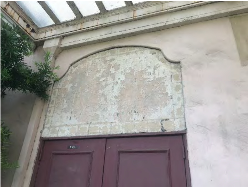
50. Auditorium Building, recessed area above door
