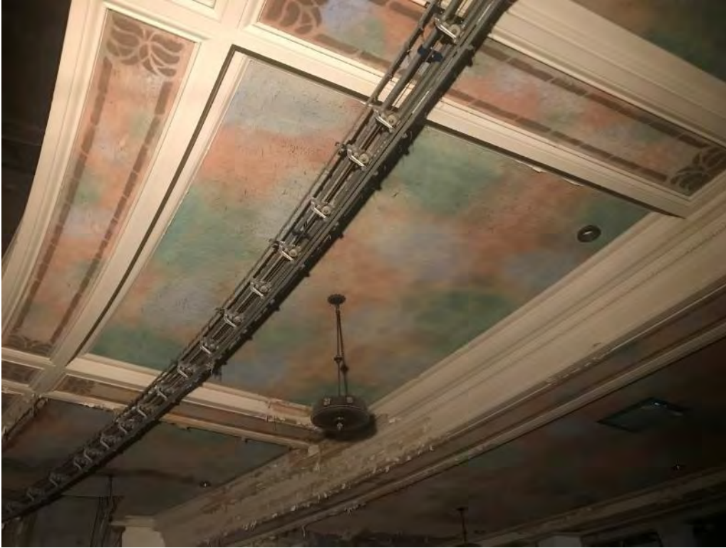
75. Auditorium Building, interior, ceiling under the balcony
