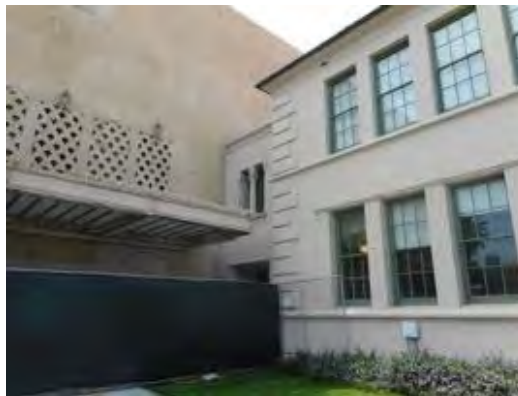
Transition where Auditorium meets west wing
