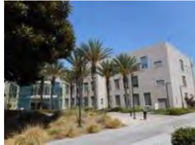
Magnolia Hall East Classroom Wing, west and south elevations
