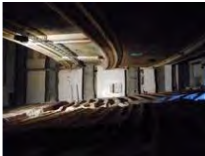
Left side (south) wall of theater with retrofit
