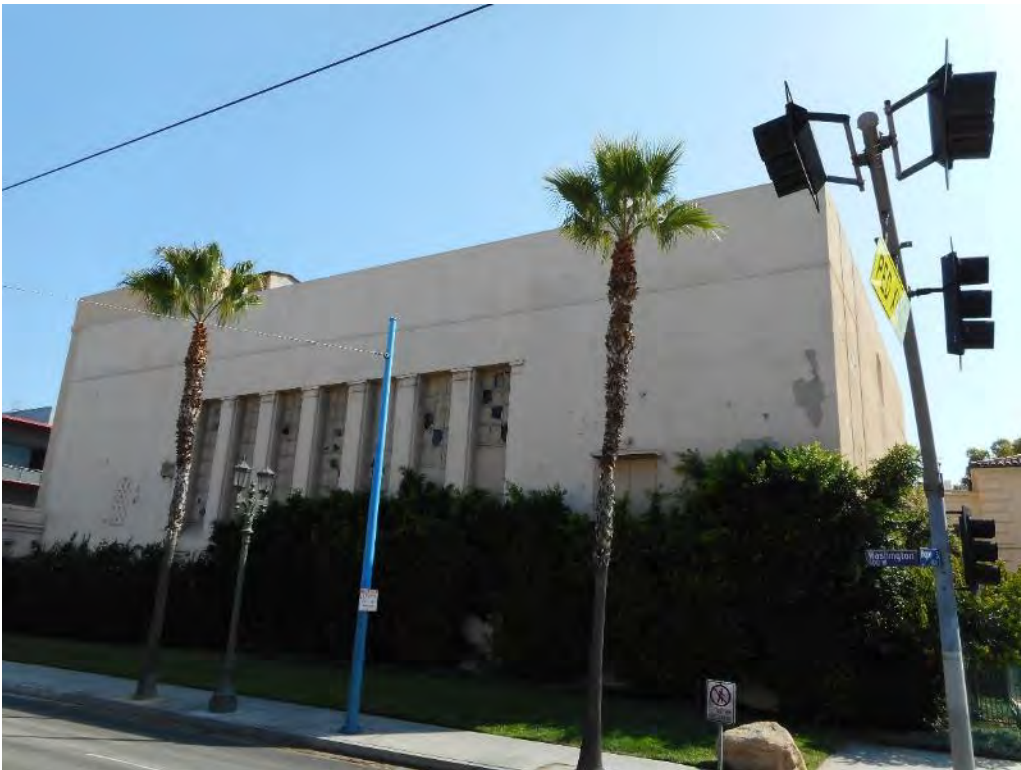
40. Auditorium Building, north elevation facing Washington Boulevard
