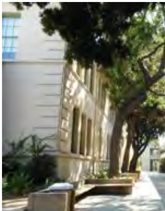
Magnolia Hall west wing, north and west elevations
