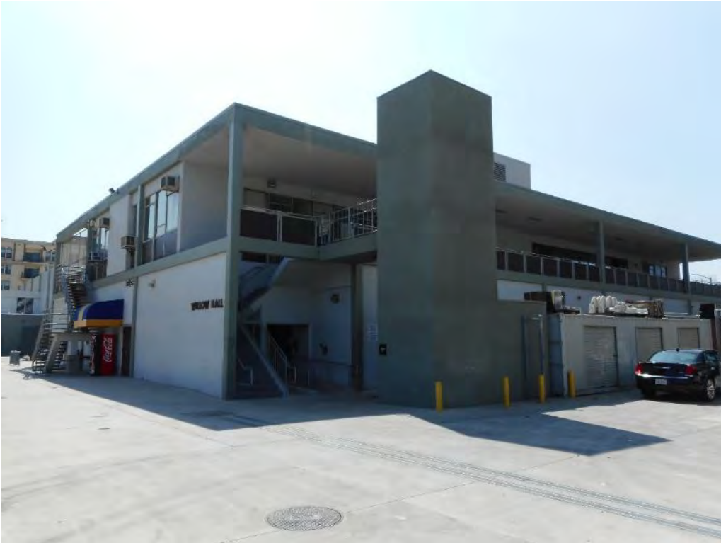
121. Willow Hall north and east elevations
