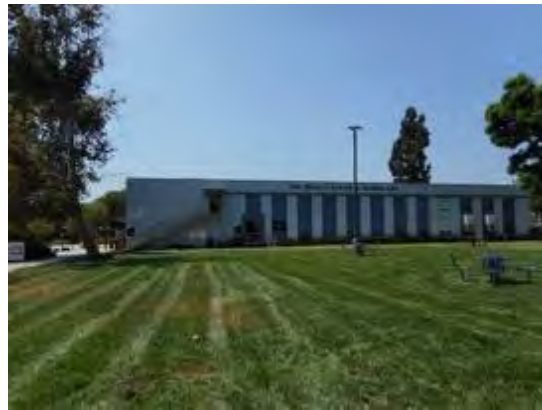
TBCSL/Redwood Hall east elevation; Addition at south end; North Quad in foreground
