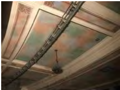
Ceiling under balcony
