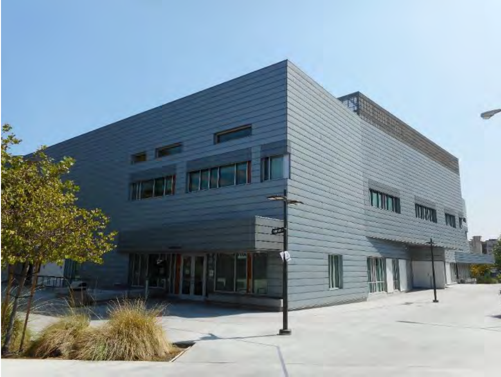
147. Mariposa Hall north and west elevations
