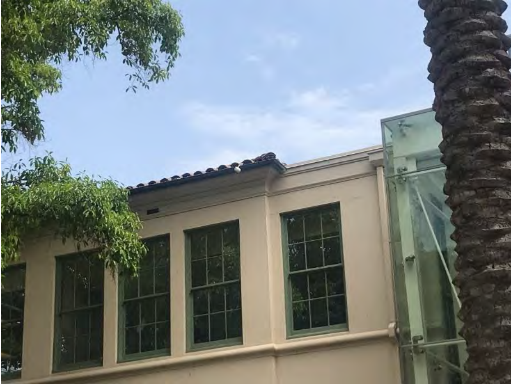
23. Magnolia Hall, south elevation of main wing, roof detail
