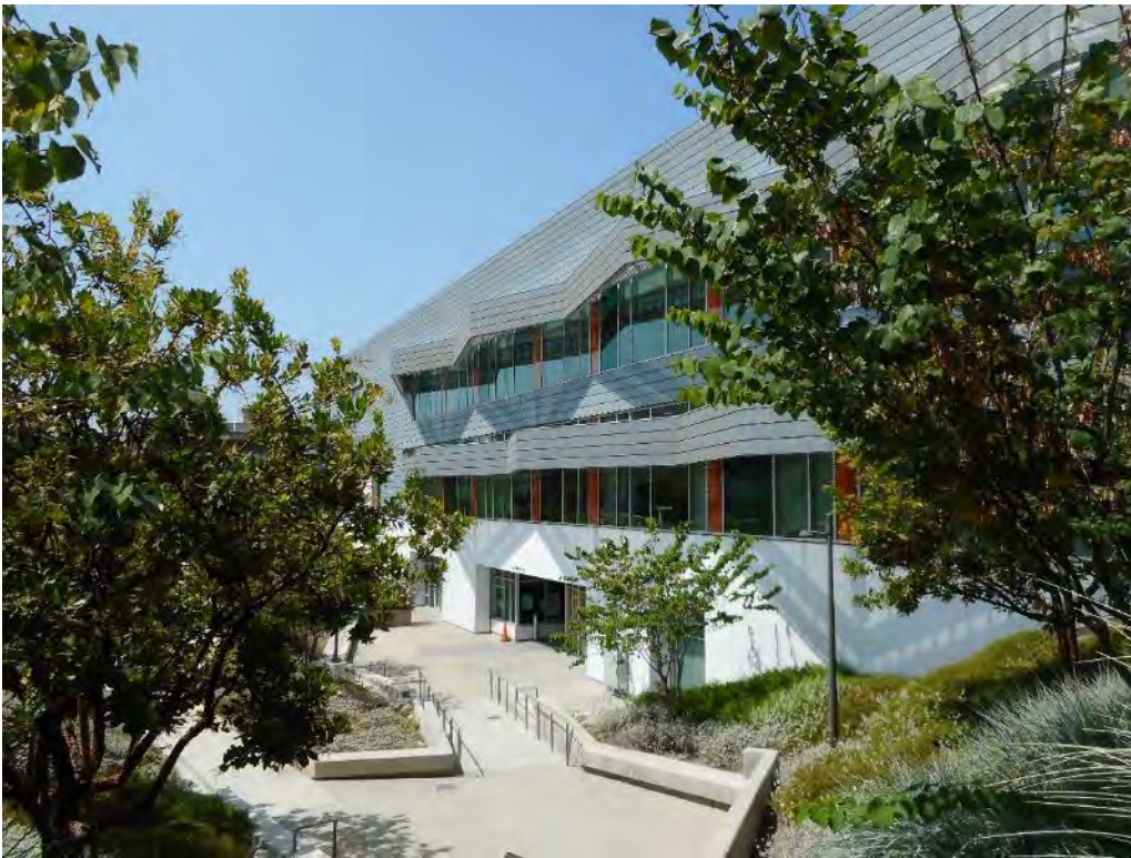
144. Mariposa Hall south elevation
