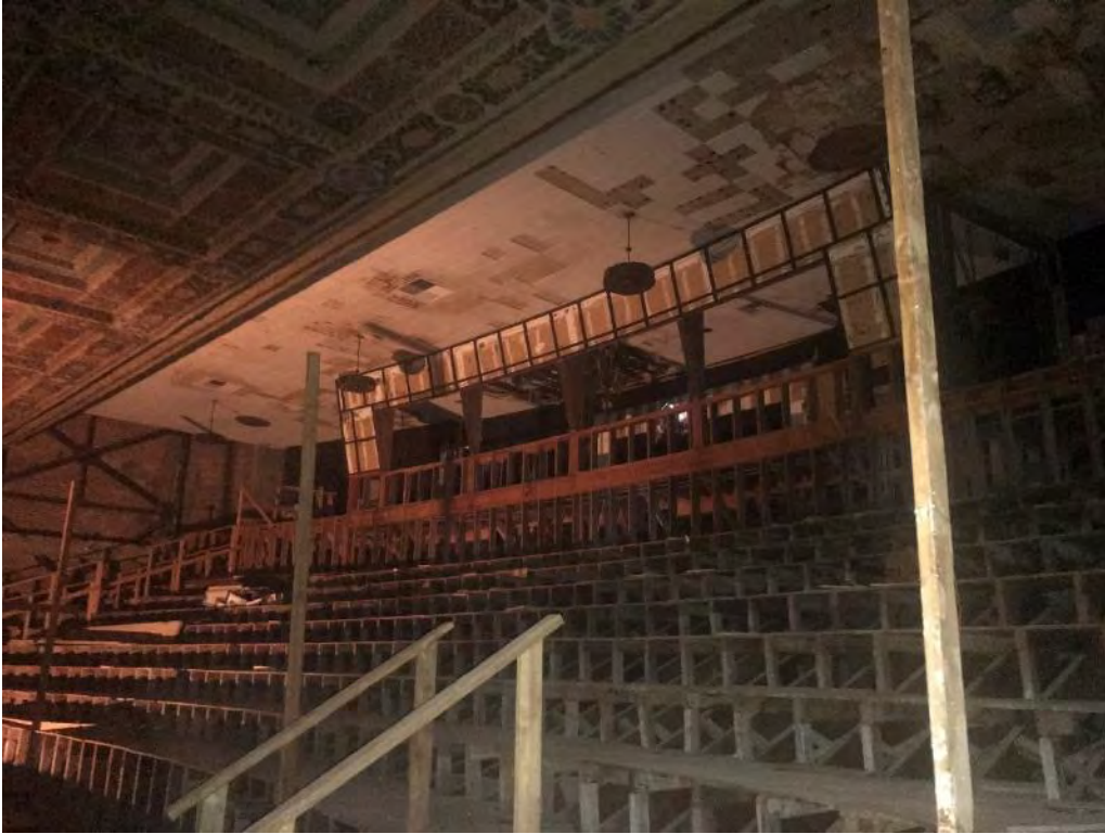
71. Auditorium Building, interior rear of balcony and seating
