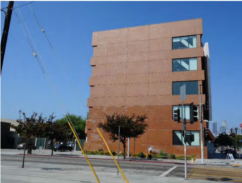
126. Aspen Hall south elevation
