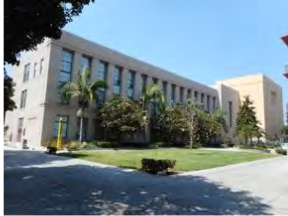
South and east elevations
