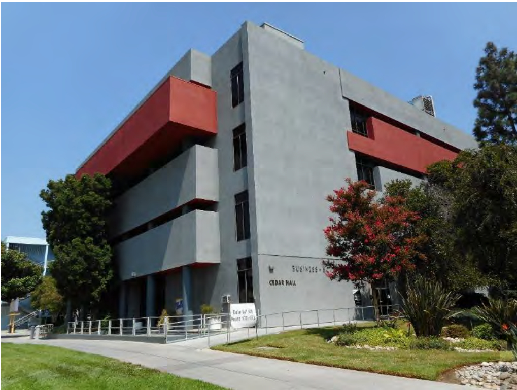
134. Cedar Hall south and west elevations
