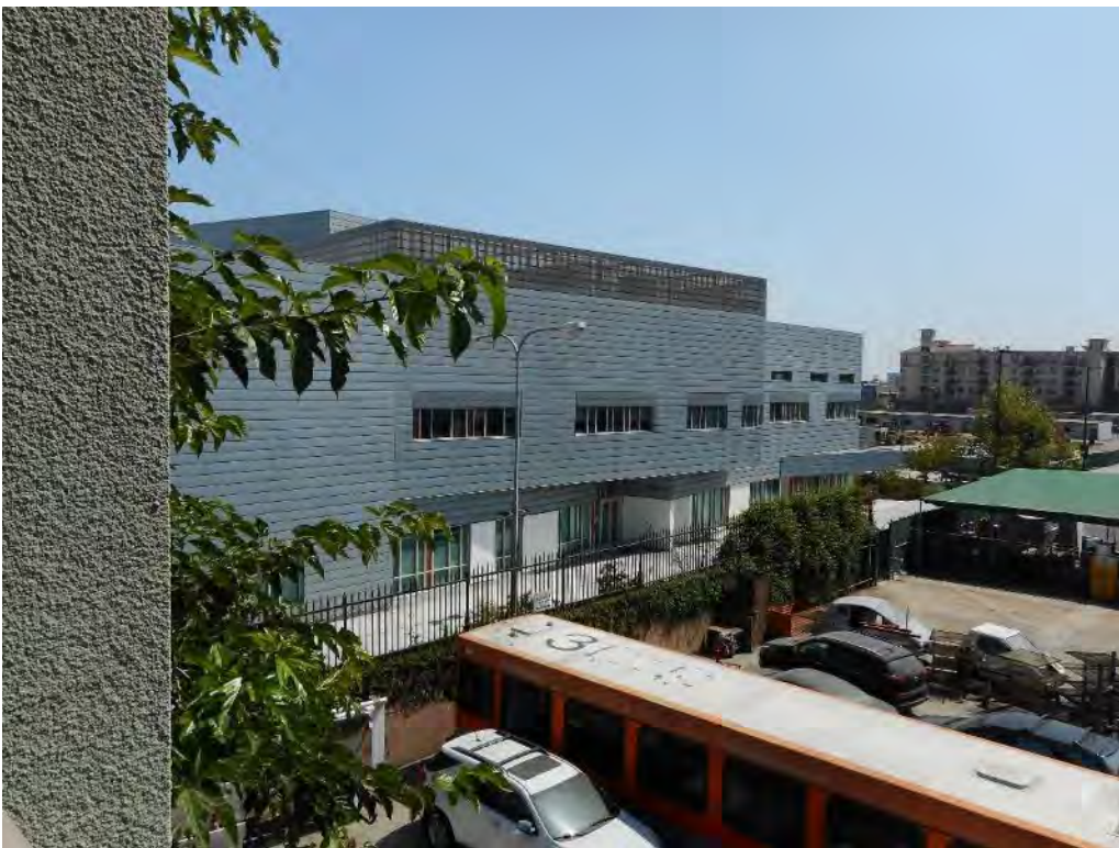
148. Mariposa Hall west elevation
