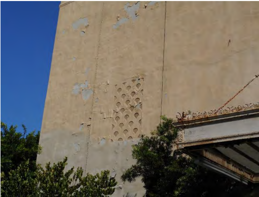
52. Auditorium Building, close up of west elevation
