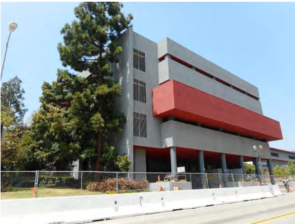
90. Cedar Hall along Grand Avenue
