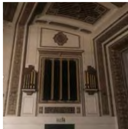
Detail of stage side wall 2018
