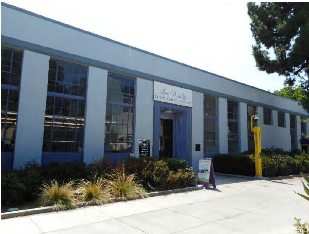
152. Tom Bradley Center for Student Life north elevation
