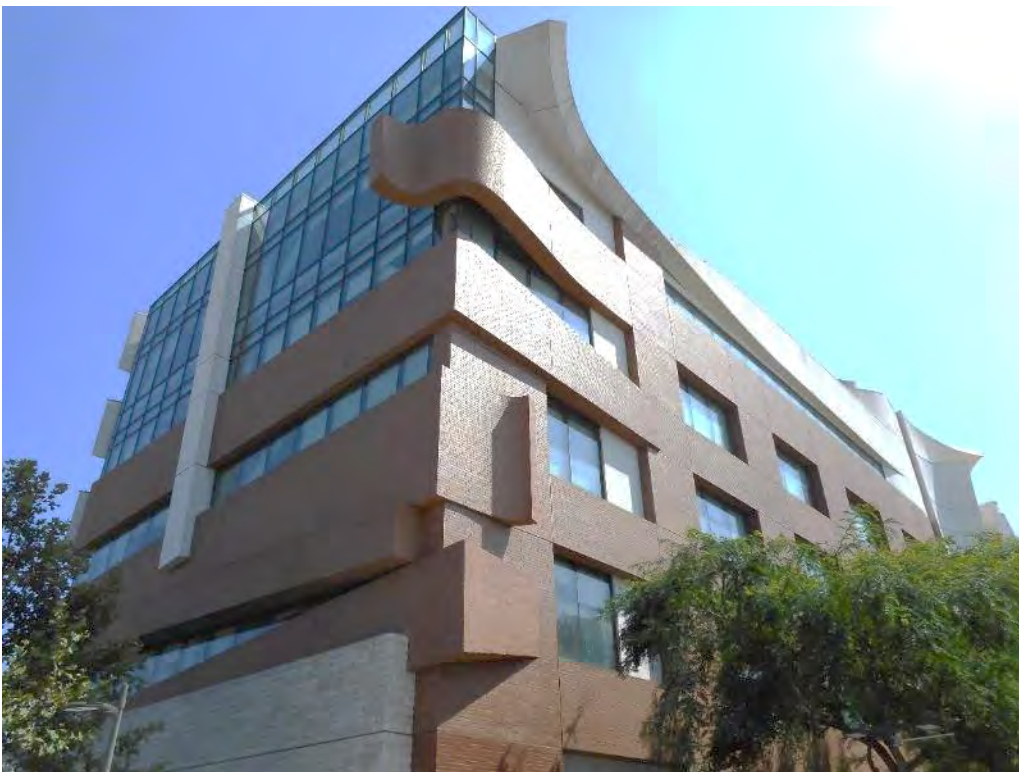
130. Juniper Hall north and west elevations
