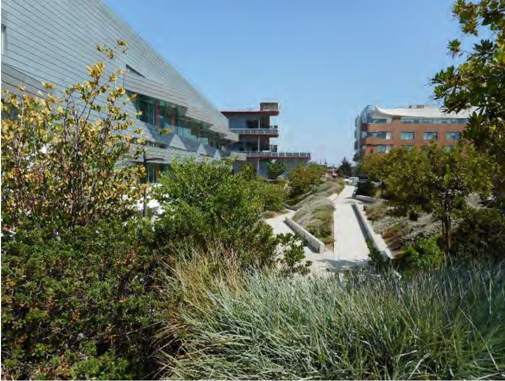
145. Mariposa Hall south elevation
