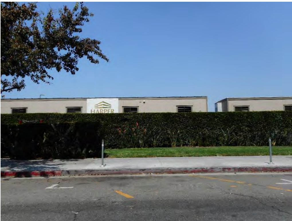
100. Construction area along 23 rd Street
