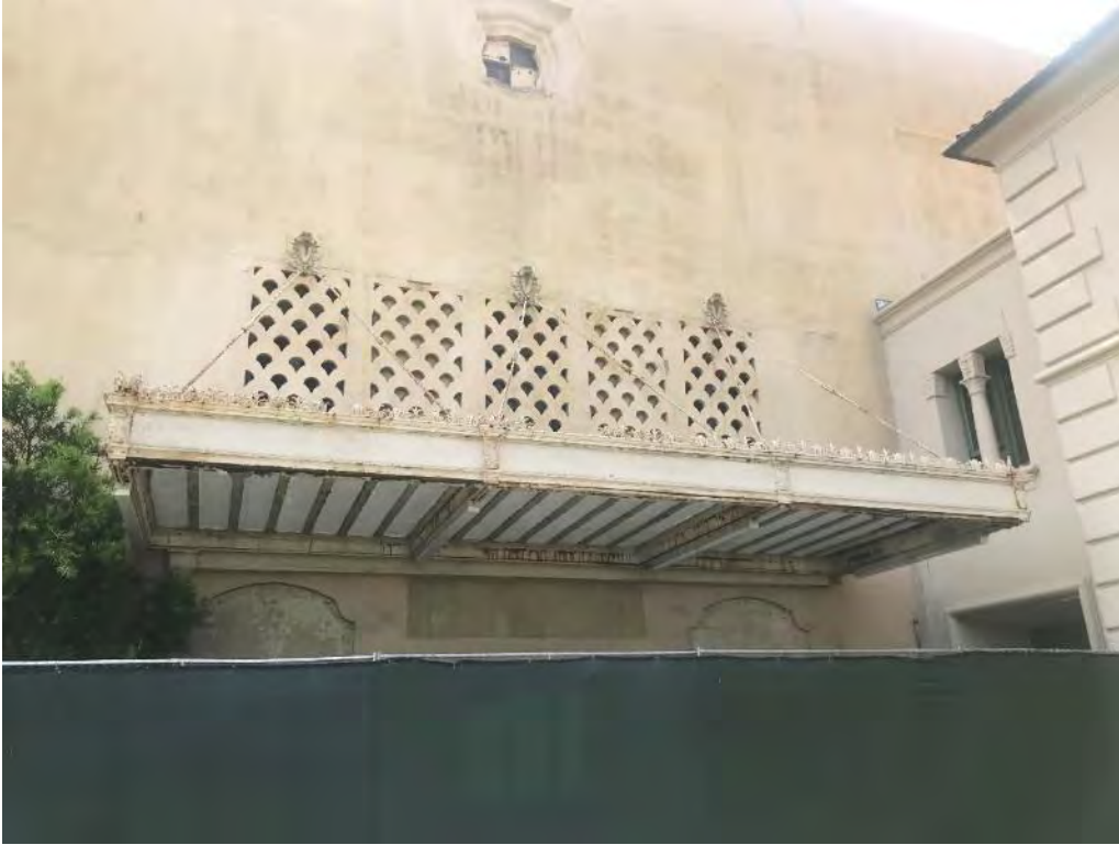
47. Auditorium Building, concrete screen and canopy
