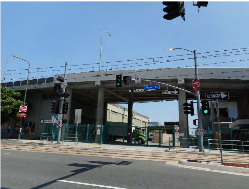
108. Oak Hall and Central Receiving along Flower Street
