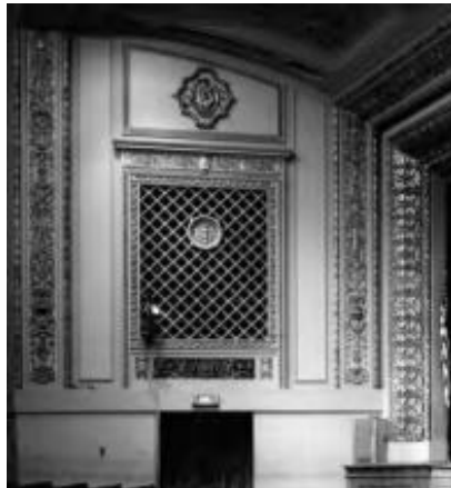
Detail of stage side wall c1981
