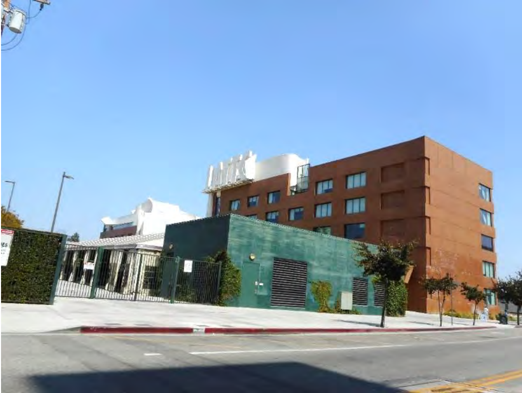
97. Aspen Hall and South Campus Utility building along 23 rd Street
