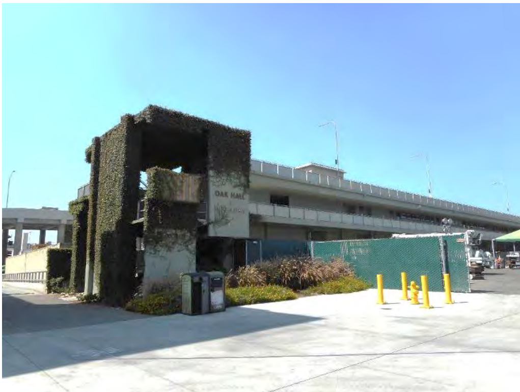
116. Oak Hall, south end, south and east elevations
