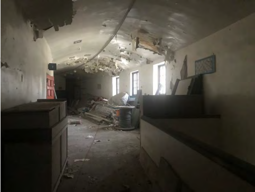
69. Auditorium Building, interior balcony lobby area
