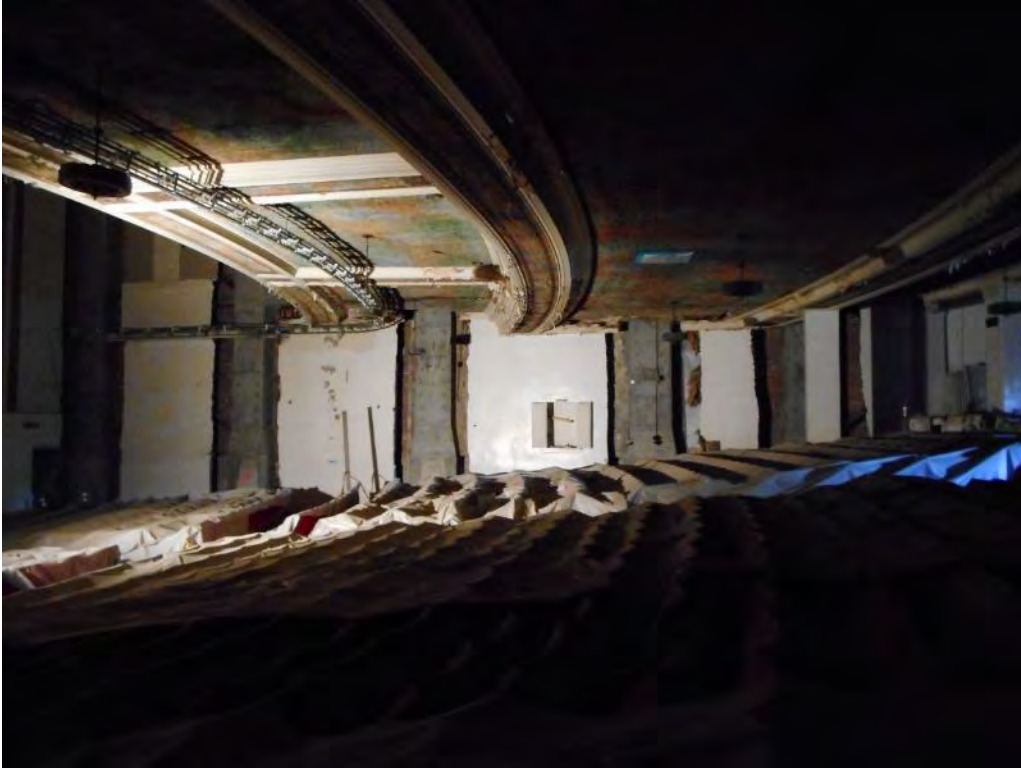
67. Auditorium Building, interior right side of auditorium
