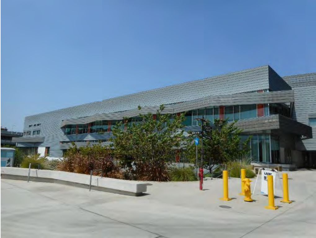
141. Mariposa Hall south elevation
