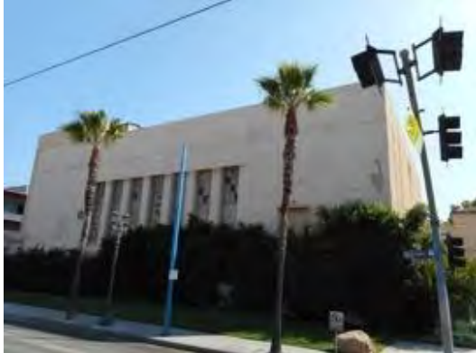
Washington Boulevard (north) elevation
