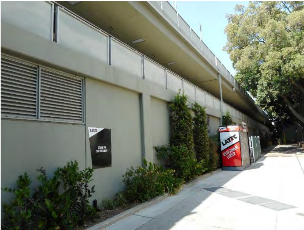
114. Oak Hall east elevation
