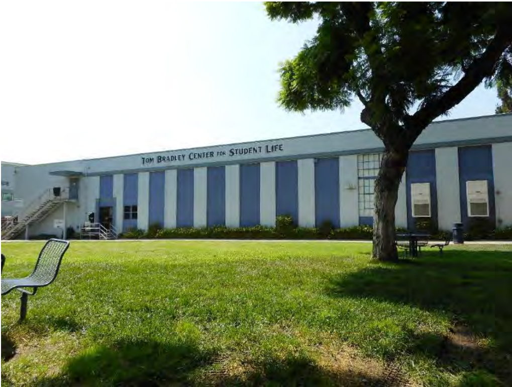
150. Tom Bradley Center for Student Life east elevation
