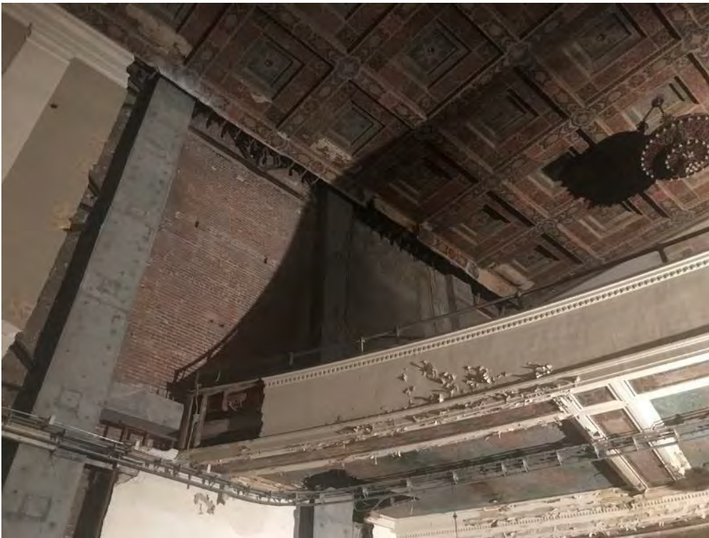
74. Auditorium Building, interior, wall and ceiling detail
