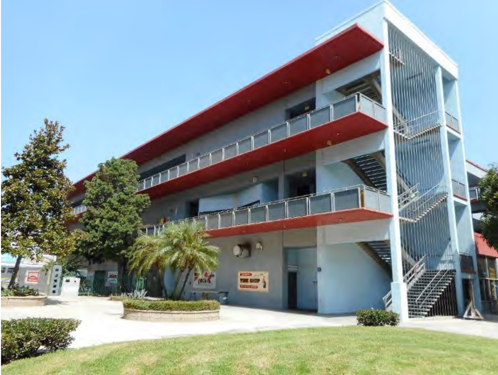
139. Sage Hall west and south elevation
