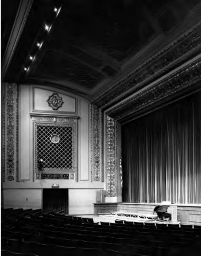
79. Auditorium Building, interior c1981
