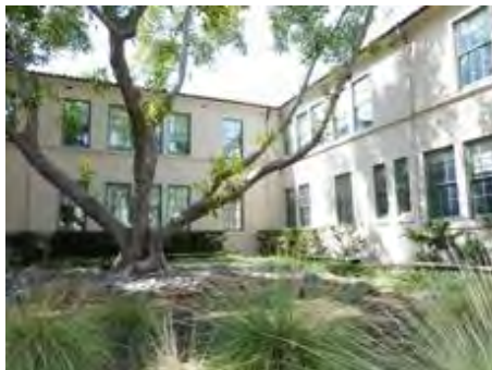
Magnolia Hall west wing, east and south elevations
