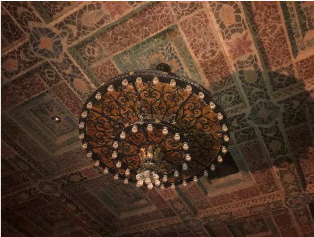
76. Auditorium Building, interior, ceiling and light fixture detail
