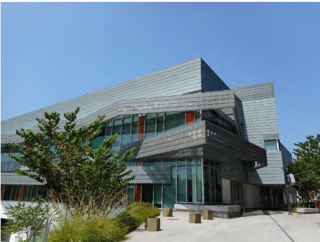
142. Mariposa Hall east end of south elevation
