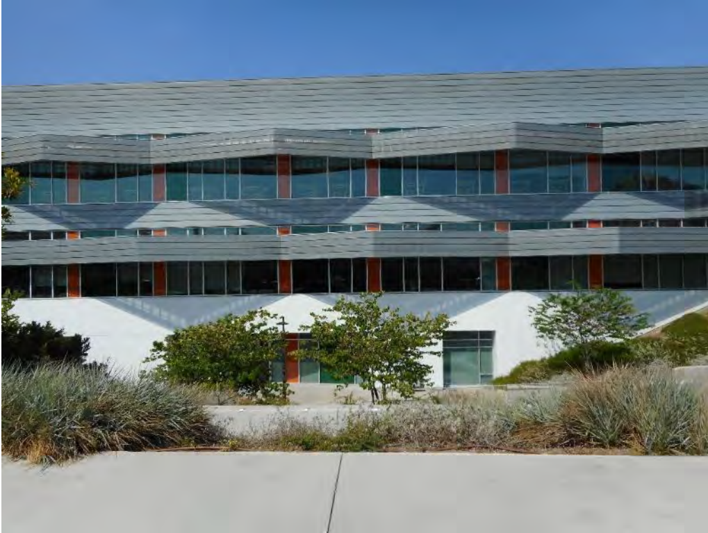
143. Mariposa Hall middle of south elevation
