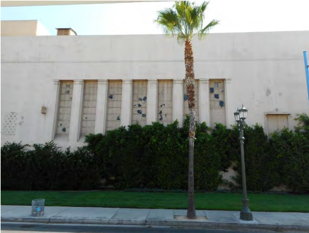
41. Auditorium Building, windows along north elevation
