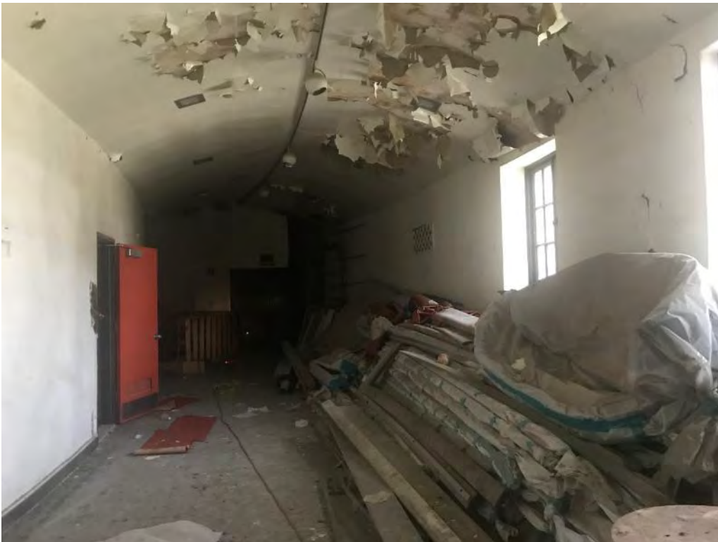
70. Auditorium Building, interior balcony lobby area
