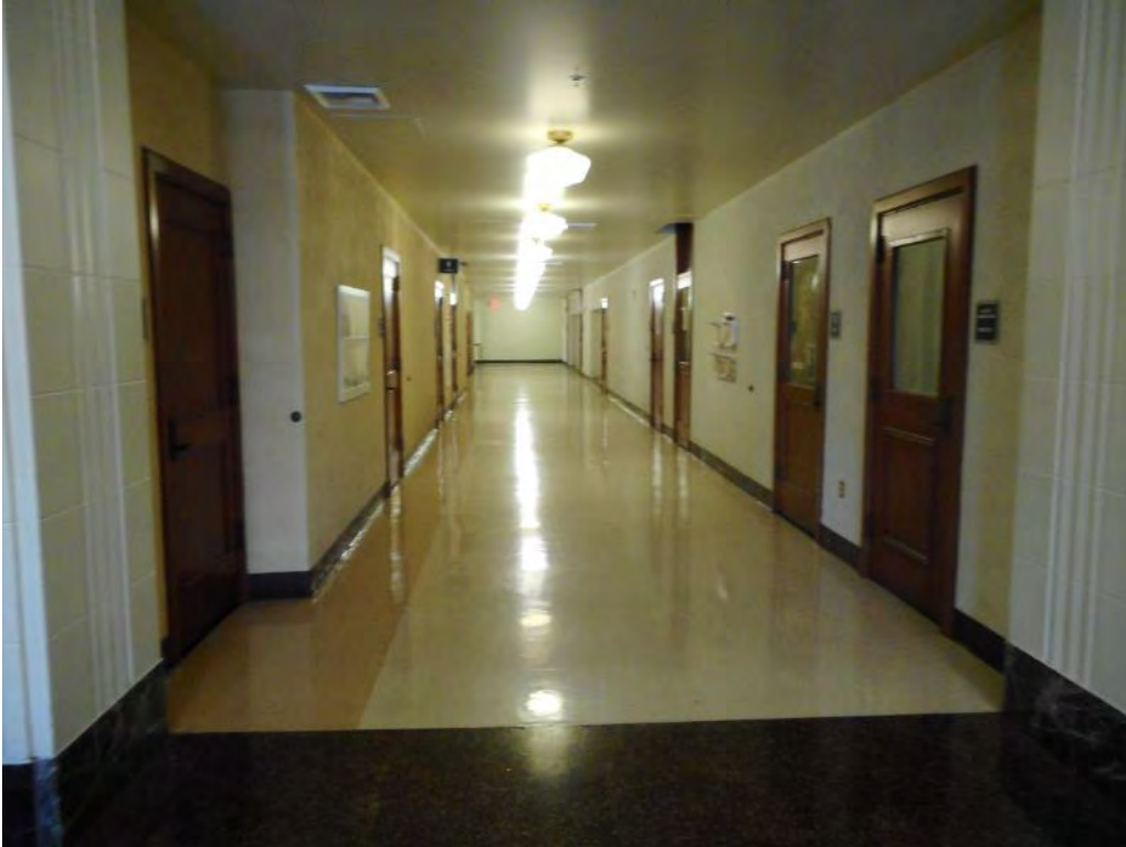
35. Magnolia Hall interior corridor
