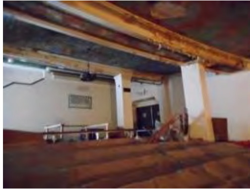
Area under balcony looking to lobby stairs
