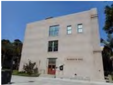
Magnolia Hall East Classroom Wing south elevation
