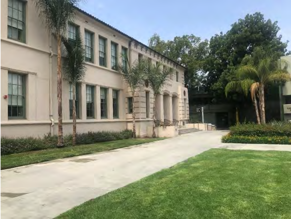
7. Magnolia Hall, north elevation
