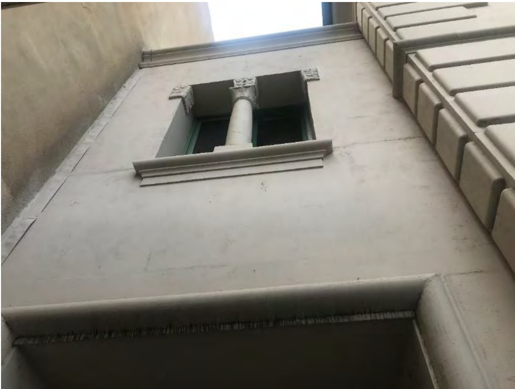
46. Connection between Auditorium Building and Magnolia Hall
