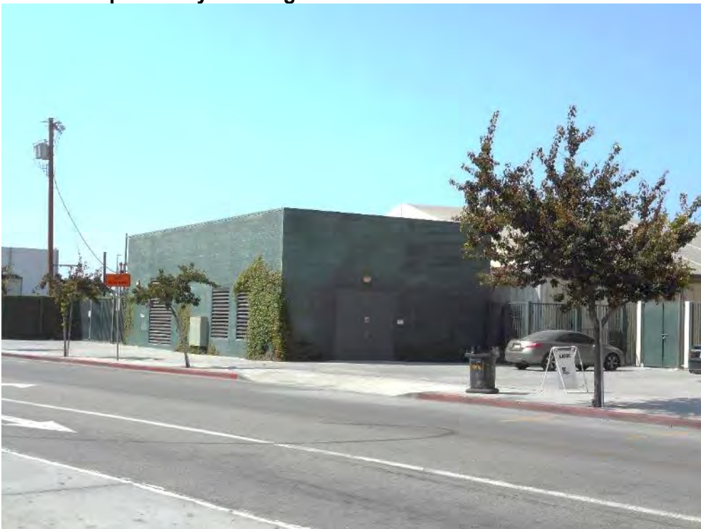
124. South Campus Utility Building south and east elevations Aspen Hall and Juniper Hall
