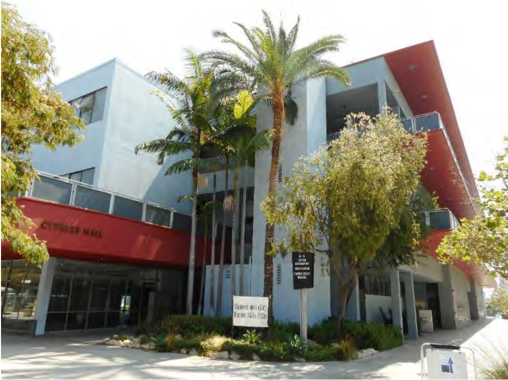
133. Cypress Hall north and west elevations
