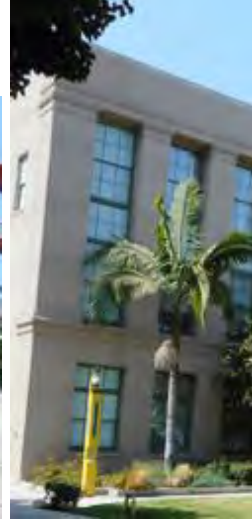
Window detail on east elevation
