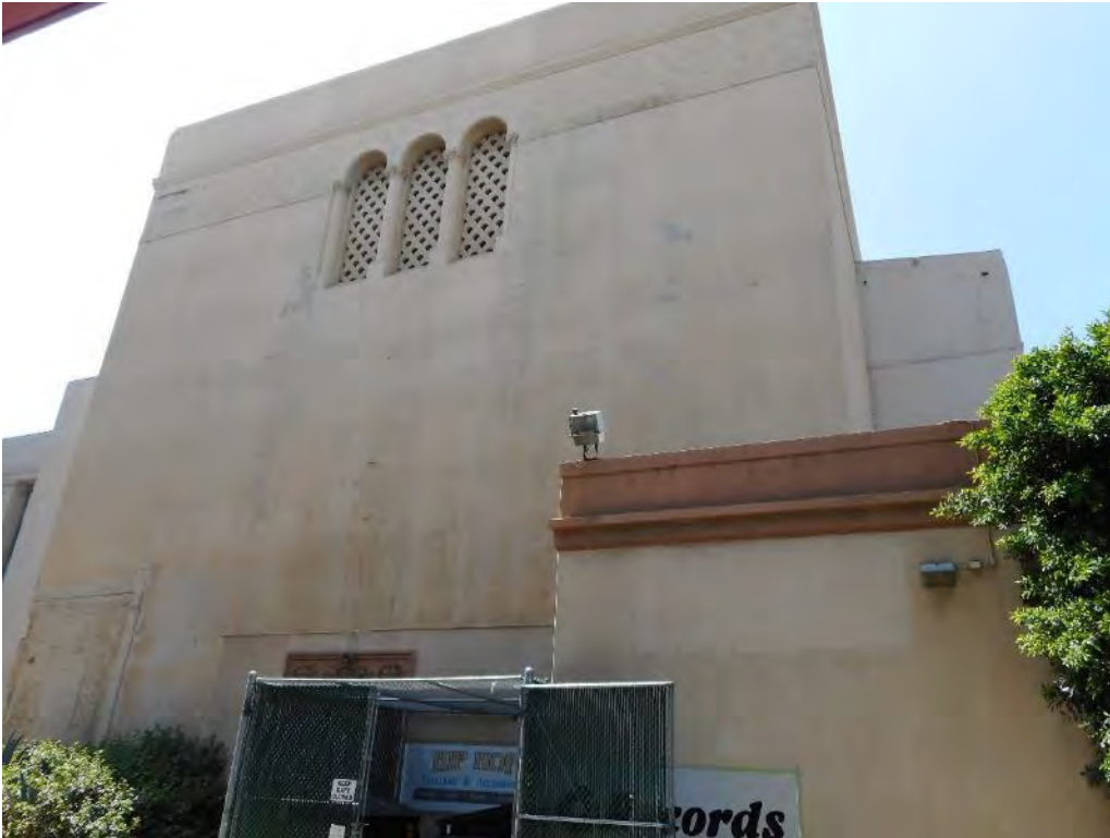
37. Auditorium Building, east elevation
