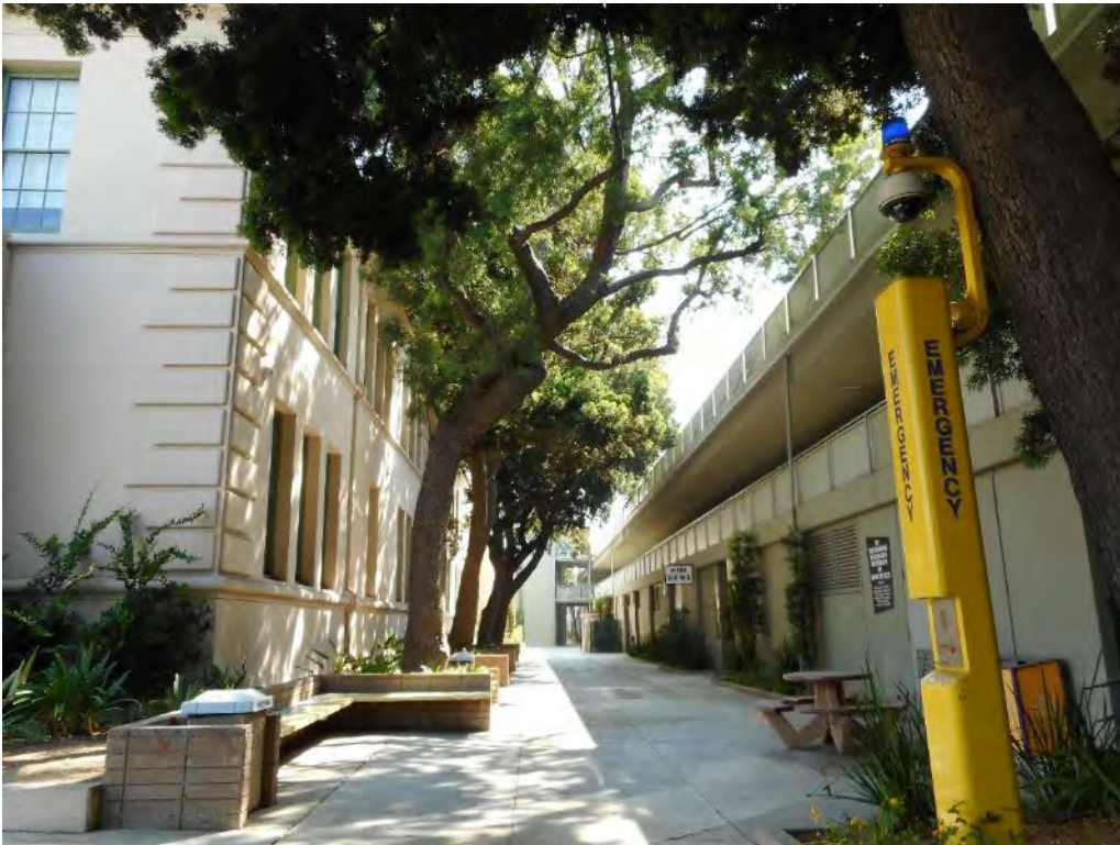
112. Oak Hall east elevation
