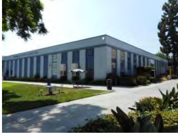
TBCSL/Redwood Hall east and north elevations
