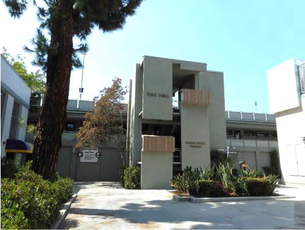
113. Oak Hall east elevation
