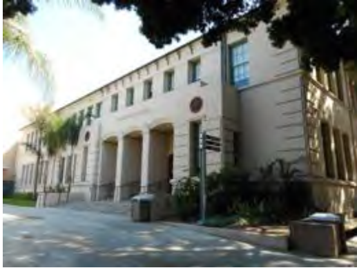
Magnolia Hall west wing, front (north) elevation
