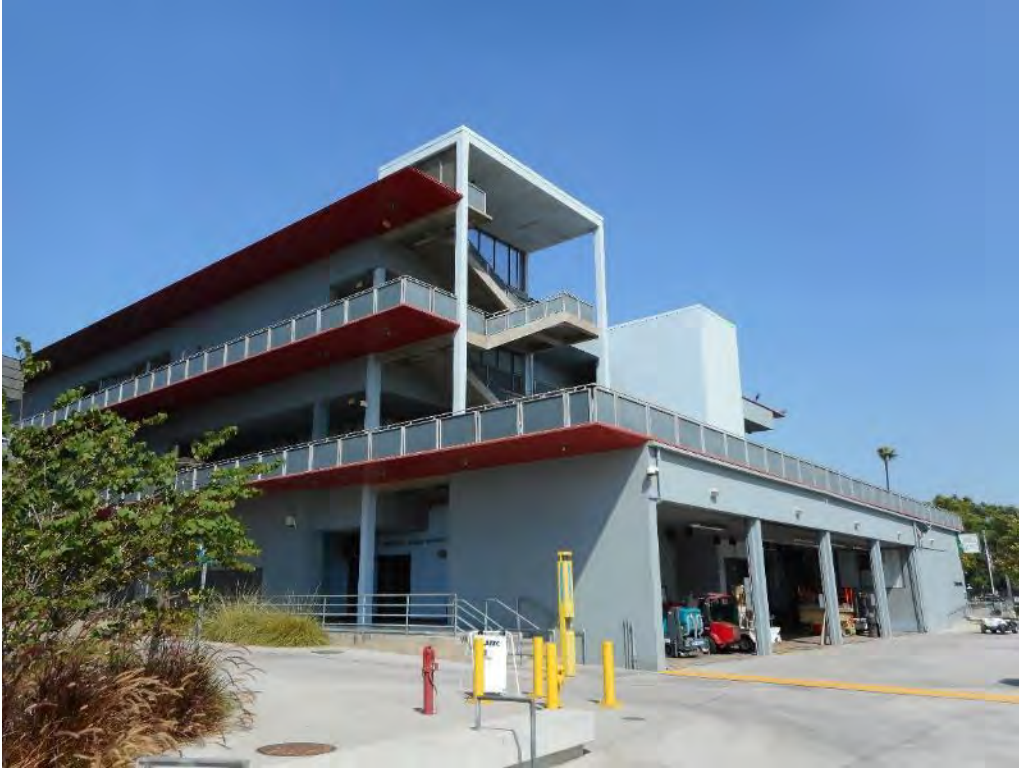
131. Cypress Hall south and west elevations
