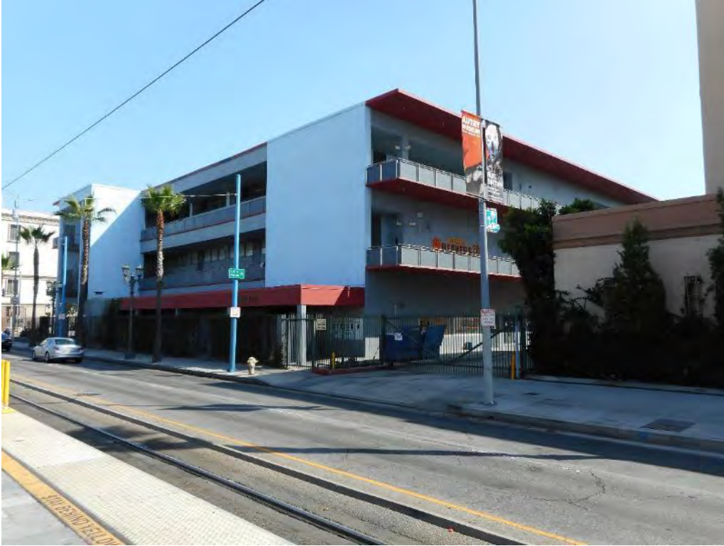
87. Sage Hall along Washington Boulevard
