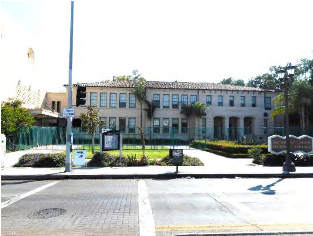
5. Magnolia Hall, north elevation facing Washington Boulevard
