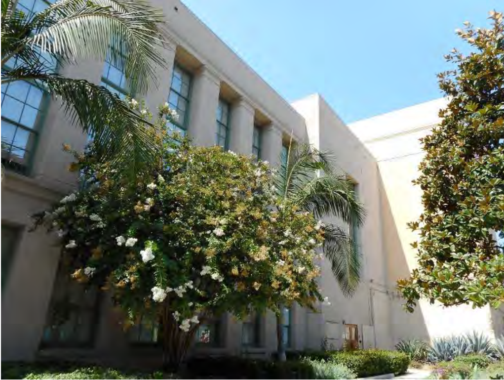
29. Magnolia Hall, east elevation of east wing where it meets the auditorium
