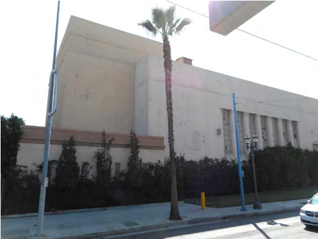
39. Auditorium Building, north elevation facing Washington Boulevard
