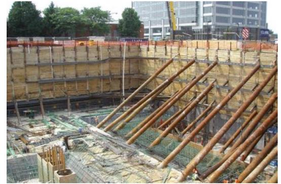
*Rakers and tiebacks provide temporary support during construction.*
