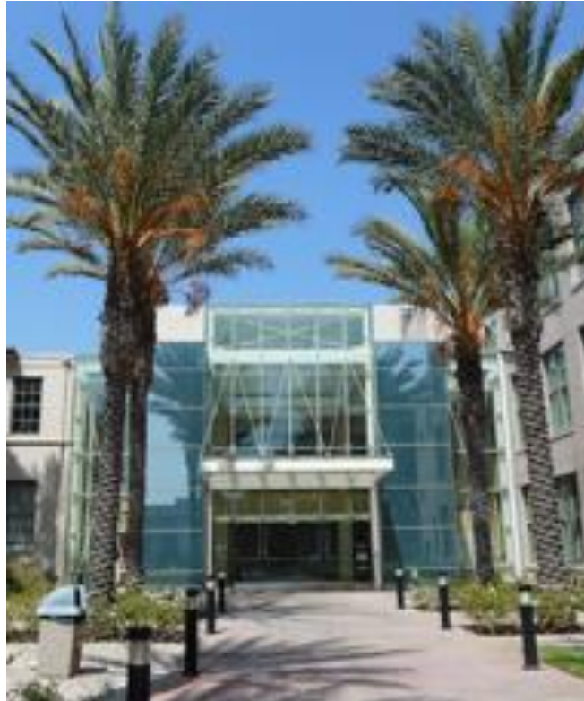
New south entrance to Magnolia Hall connecting 1935 Classroom building with the 1924 East Classroom wing
