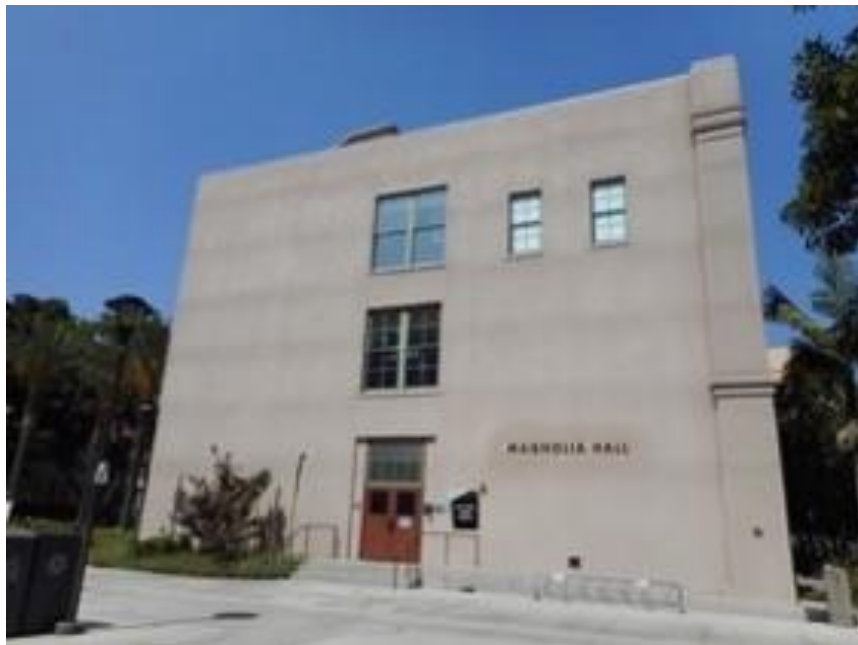
Magnolia Hall East Classroom Wing, south elevation
