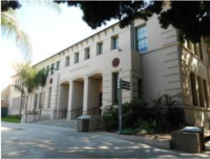
Magnolia Hall West Wing, front (north) elevation
