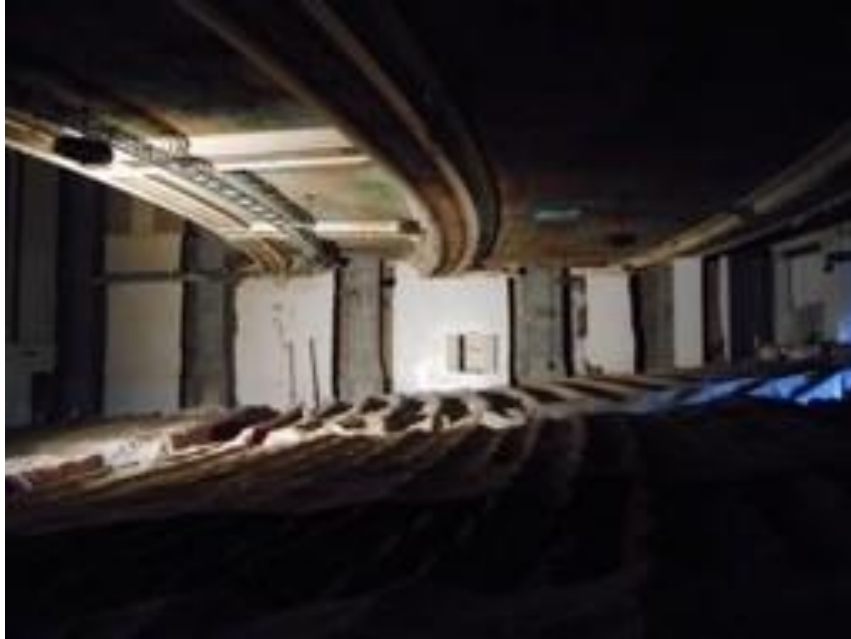
Left side (south) wall of theater with retrofit, 2018
