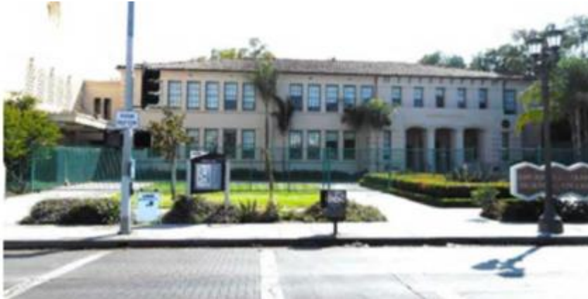
Magnolia Hall, north elevation facing Washington Boulevard; Auditorium to the left
