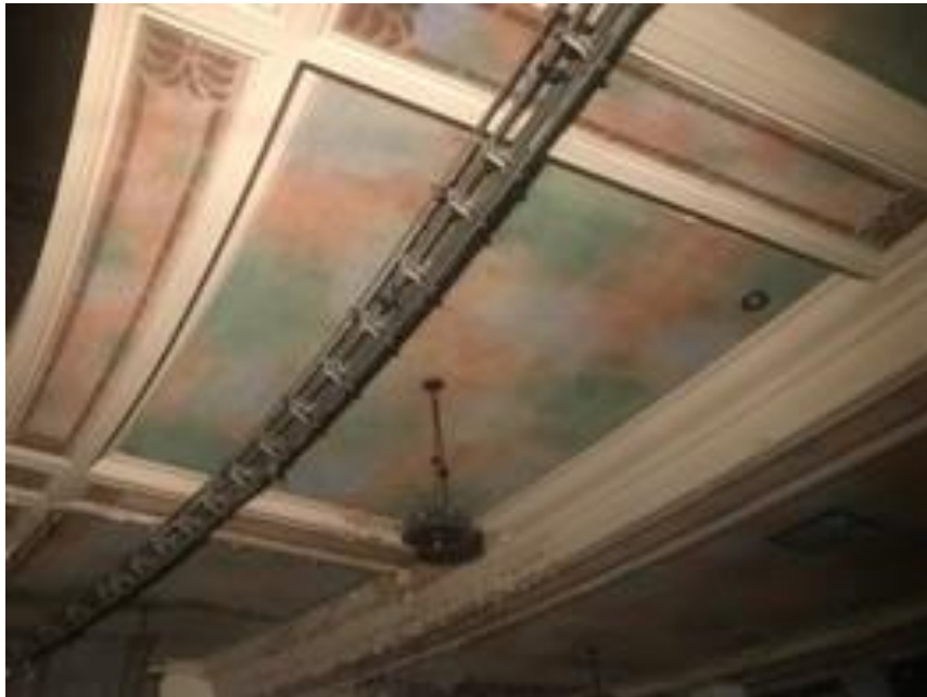
Ceiling under balcony, 2018
