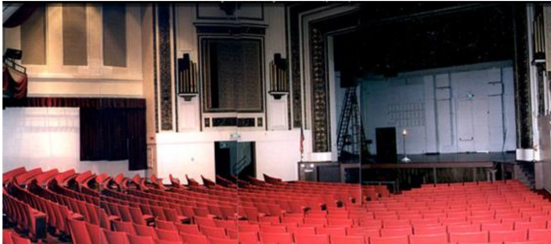
Grand Theater renovation, main floor, c1978 ( https://ca.reel-scout.com/loc_detail.aspx?id=3124&g=0&cid=50 )
