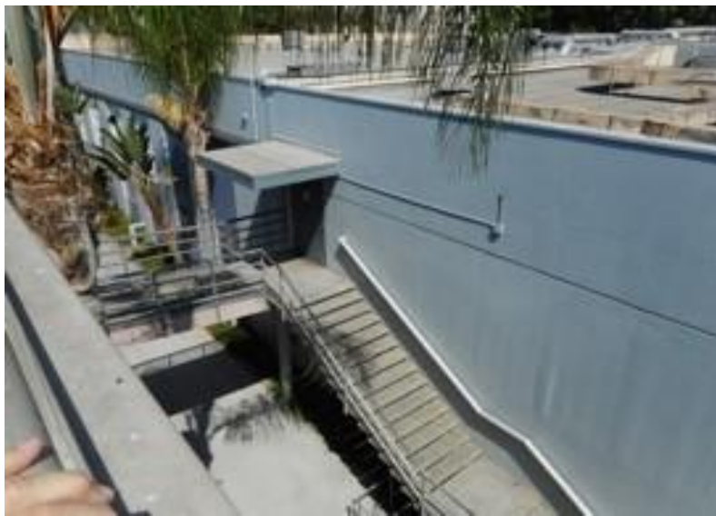
TBCSL/Redwood Hall west elevation with 1956 addition
