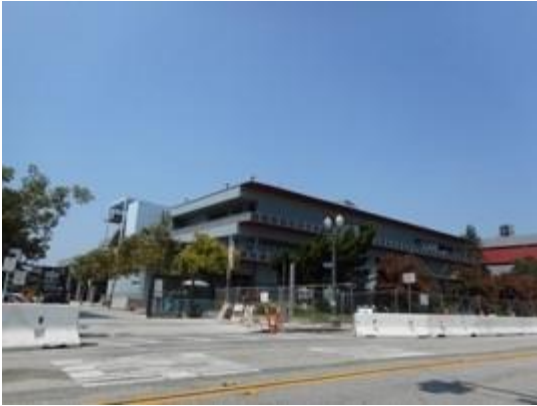
Toyon Hall, south and east elevations
