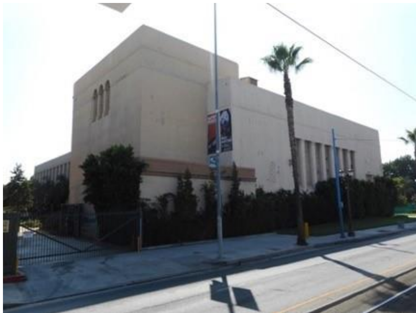
Auditorium, east and north elevations
