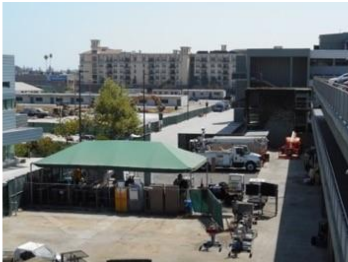
Construction area on south end of LATTC campus
