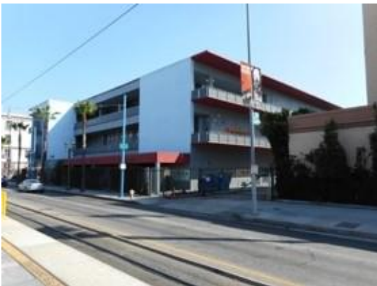
Sage Hall, north and west elevations
