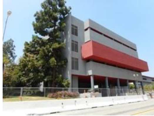
Cedar Hall, south and east elevations
