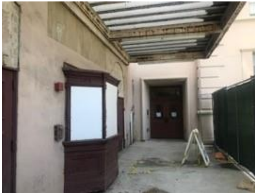
Theater entrance/ticket booth on west elevation
