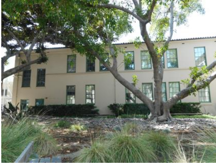
East elevation of Magnolia Hall West Classroom Building
