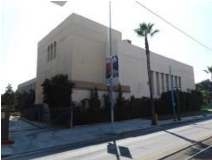
Auditorium, east and north elevations
