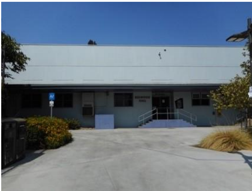
Tom Bradley Center for Student Life/Redwood Hall, 1956 addition, south elevations
