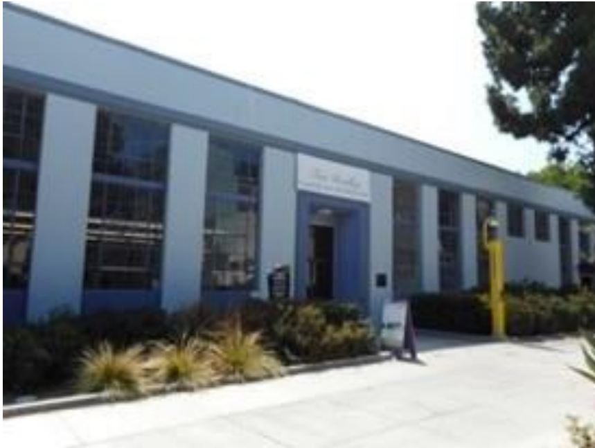
TBCSL/Redwood Hall north elevation
