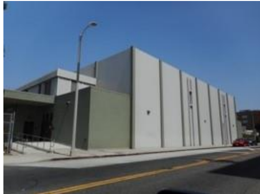
Laurel Gymnasium, west and south elevation
