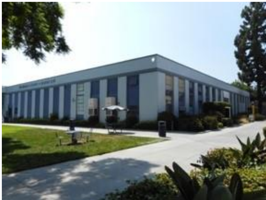
TBCSL/Redwood Hall east and north elevations
