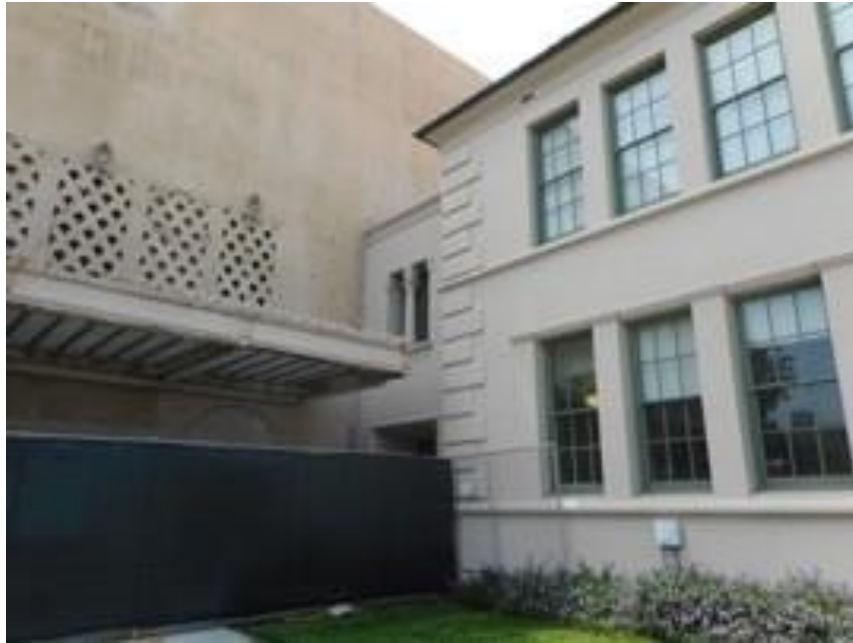
Transition where Auditorium meets west wing
