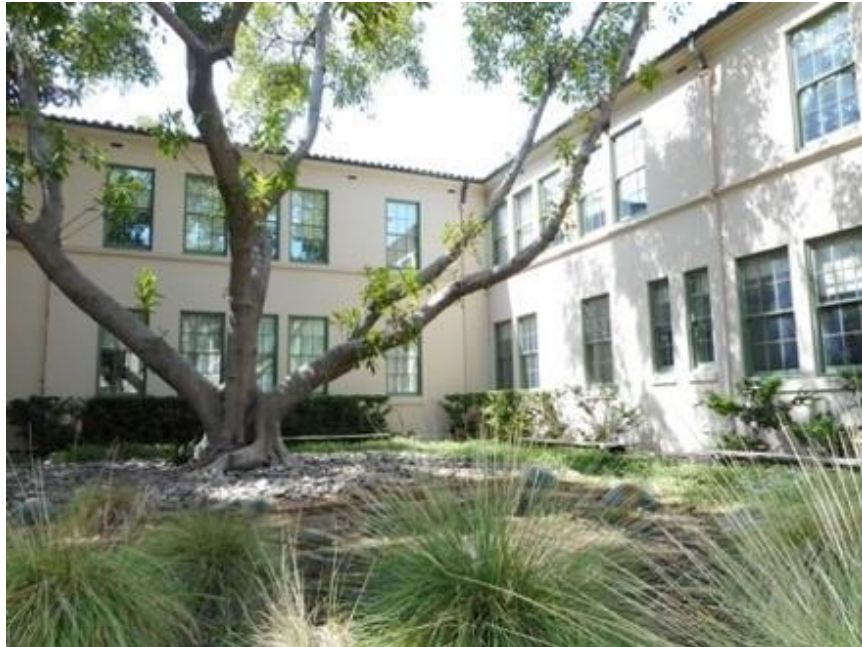
Magnolia Hall (west wing), south and east elevations
