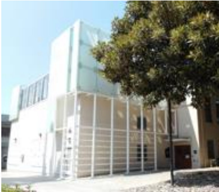
Contemporary addition to south end of the west wing of the 1935 classroom building
