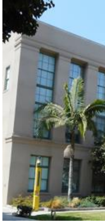
Window detail on east side
