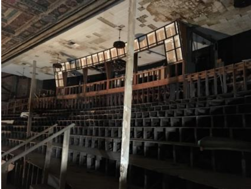
Balcony and ceiling above balcony, 2018
