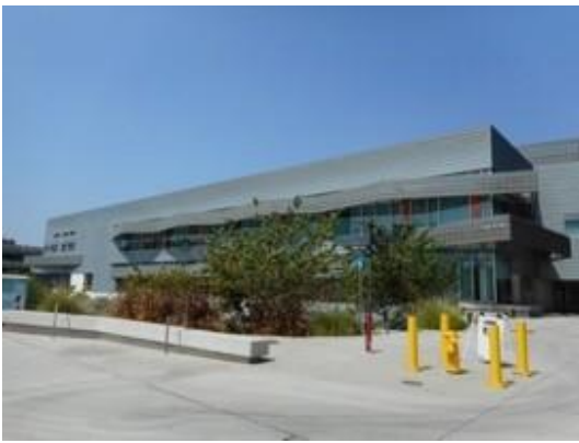
Mariposa Hall, south elevation
