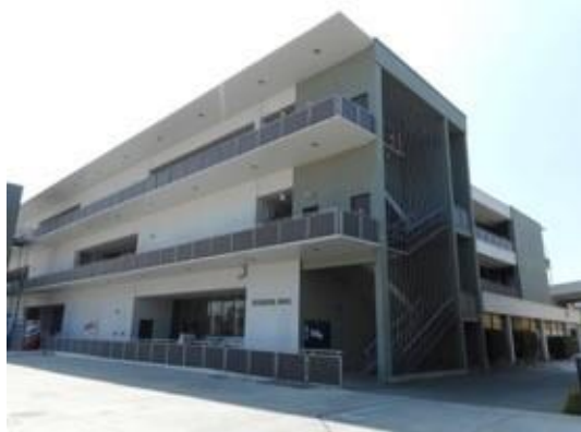
Sequoia Hall, east and north elevations
