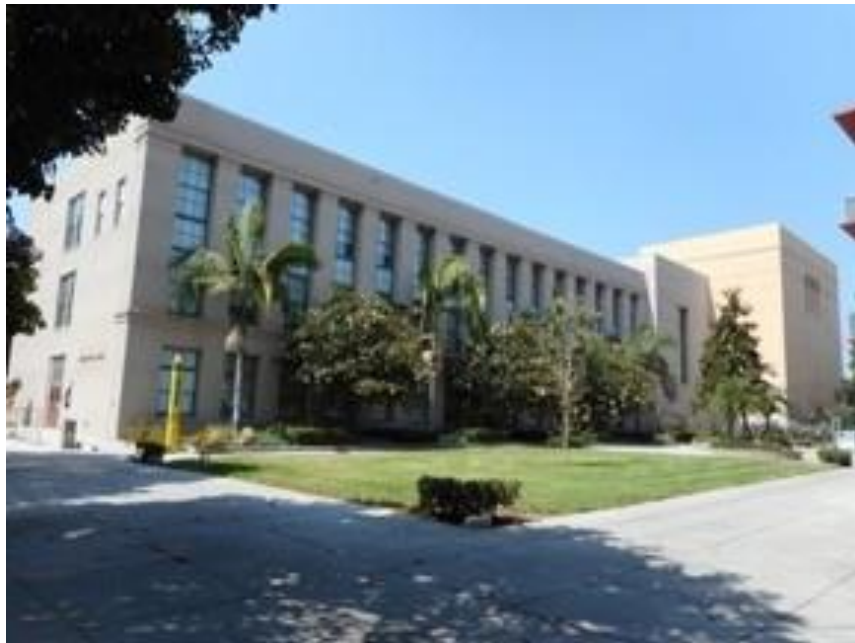
Magnolia Hall East Classroom Wing, south and east elevations
