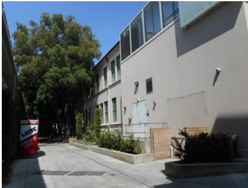
West elevation of south addition to west wing of the 1935 classroom building
