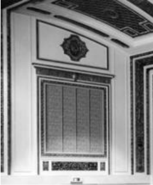
Detail of stage side wall c1978
