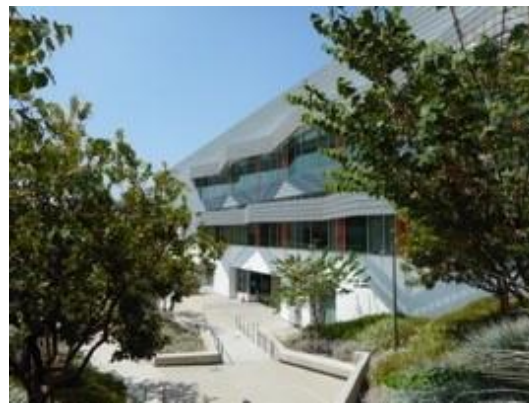
Mariposa Hall, south elevation
