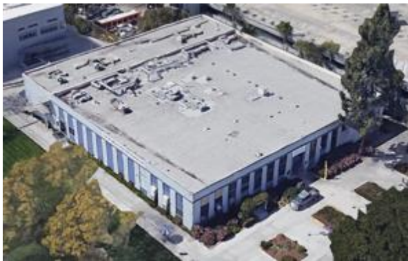
TBCSL/Redwood Hall east and north elevations (Google Earth)
