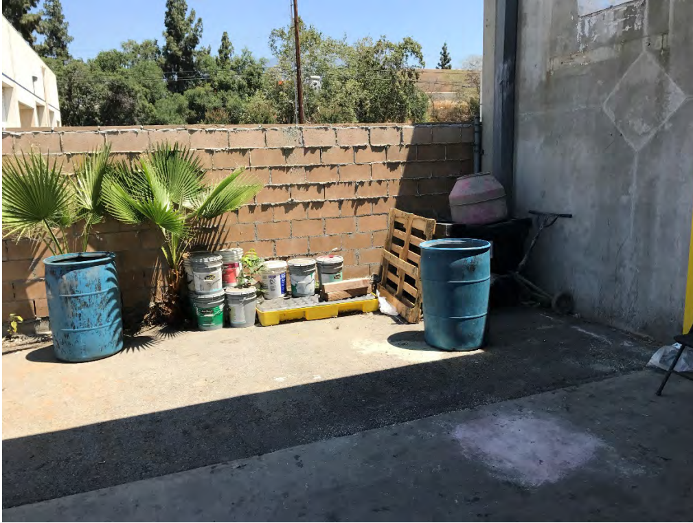
Open-top 55-gallon drums used for trash and paint buckets outside of the automotive maintenance building
