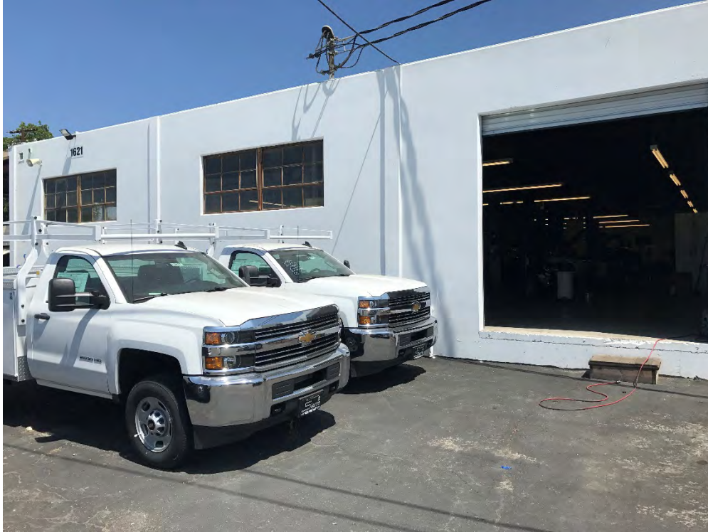
Outside view of the Sierra Chevrolet automotive maintenance building
