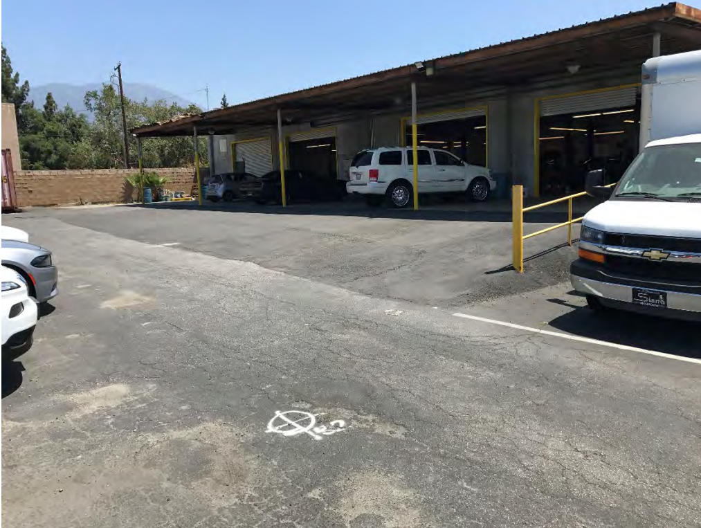
View of the automotive maintenance building from outside facing northeast with a USA marking
