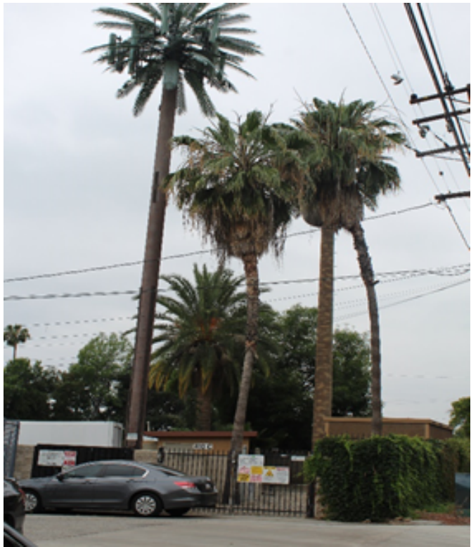
Photo 1 One of the cell towers (a monotree) in Alexan Foothills Specific Plan area.
