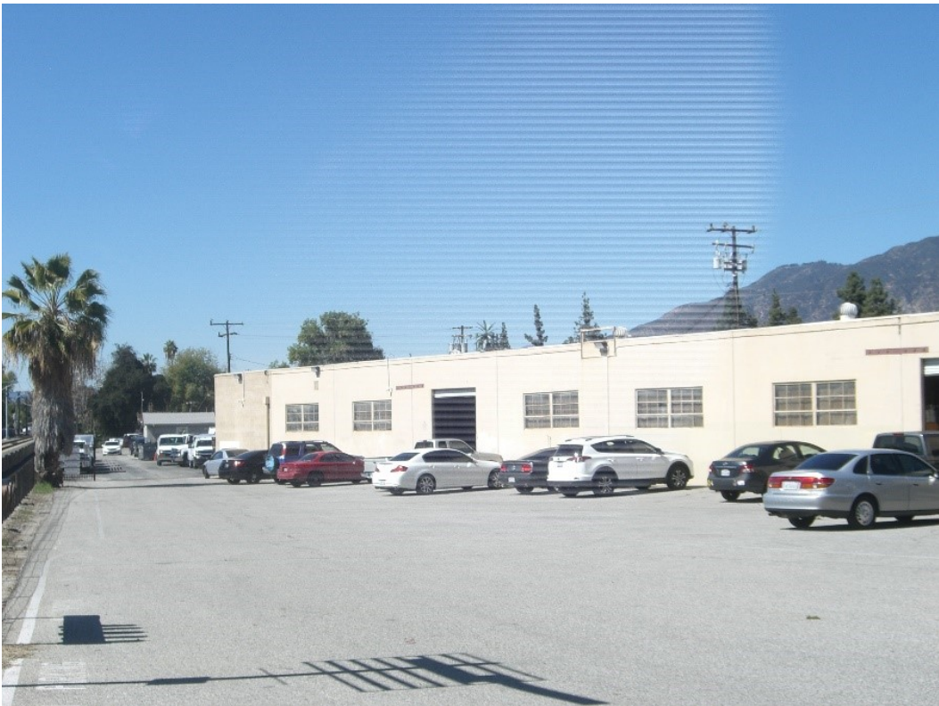
Photograph 10 1625 South Magnolia Avenue, West-looking View
