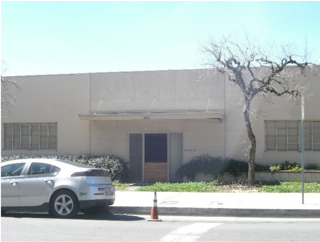
Photograph 3 1625 South Magnolia Avenue, West-looking View
