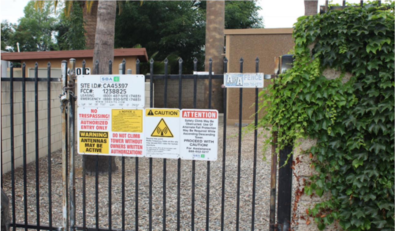
Photo 2 Protective fencing around cell towers in Alexan Foothills Specific Plan area.
