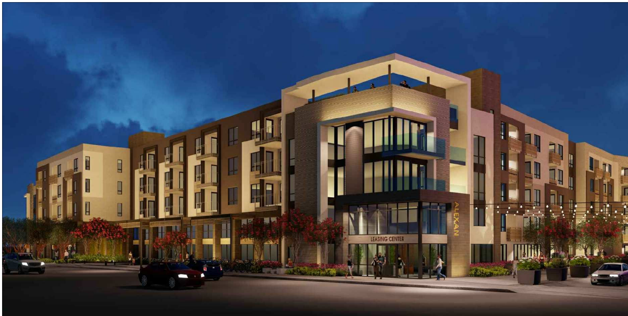
LOOKING SOUTHWEST AT LEASING AREA / ROOF DECK AMENITY
