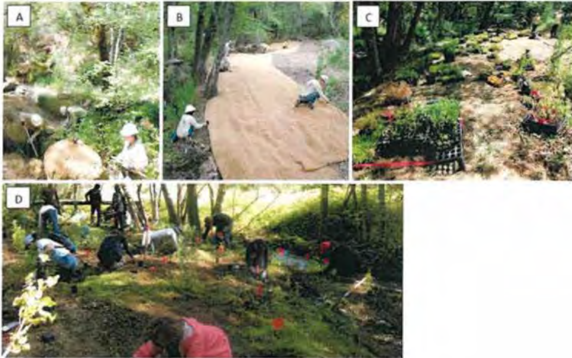
Figure 1. (A) American Conservation Experience (ACE) crew removes invasive species within the LTNC's Conn Creek riparian project area on the Linda Falls Preserve. (B) ACE crew installs erosion control blanket along Conn Creek after removing invasive Himalayan blackberry, which dominated the site. (C) Native plants, propagated from material collected within the project area, staged for planting in previously invaded areas. (D) Land Trust volunteers plant native species in a previously invaded site.
