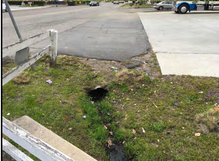
Representative Photograph 2. Facing W. Inlet
