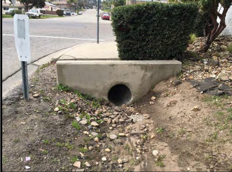
Representative Photograph 2. Facing W. Outlet
