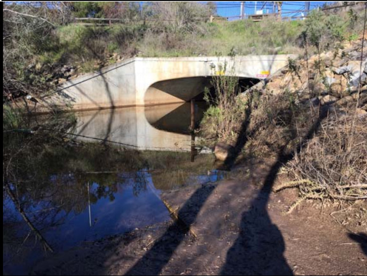
Representative Photograph 1. Facing NW. Large box culvert outlet at upstream portion of channel.
