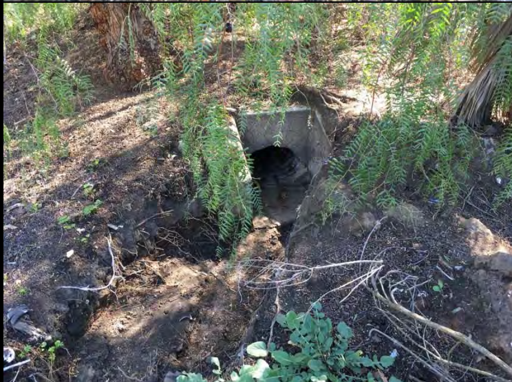
Representative Photograph 3. Facing E. Outfall
