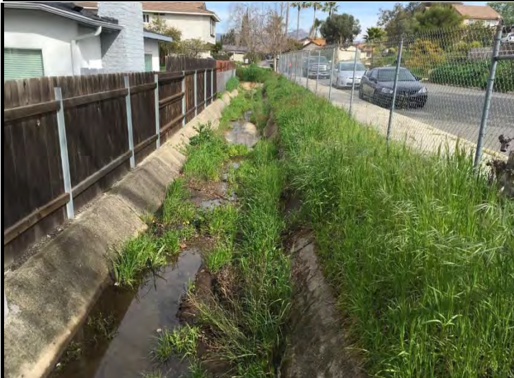
Representative Photograph 1. Facing N. Concrete-lined channel
