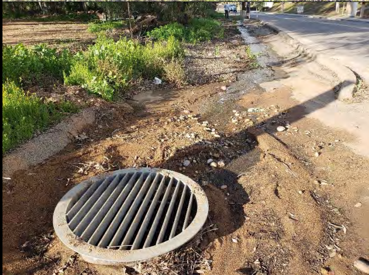
Representative Photograph 3. Facing N. Storm drain at downstream end of channel
