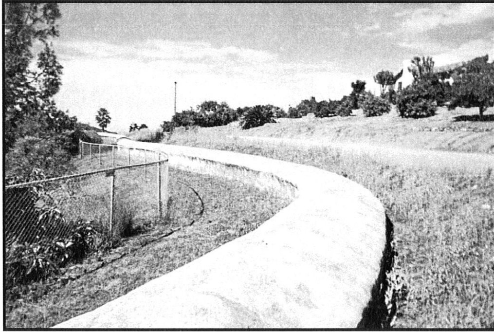
Figure 10: Typical flume section east of Pechstein Reservoir
