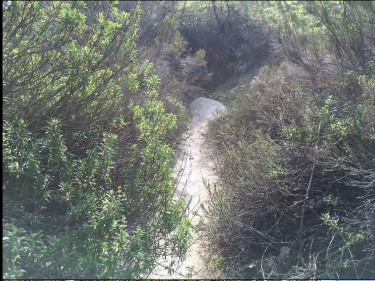
Representative Photograph 1. Facing SE. Concrete-lined channel facing downstream
