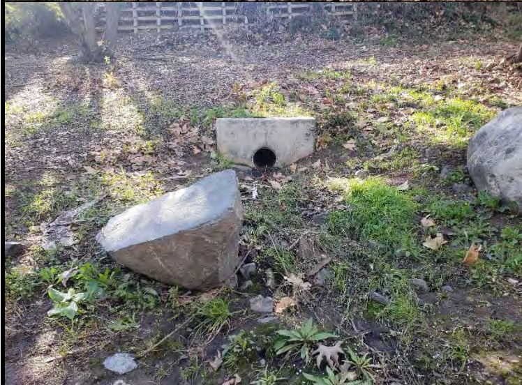
Representative Photograph 3. Facing W. Open outfall that will be maintained
