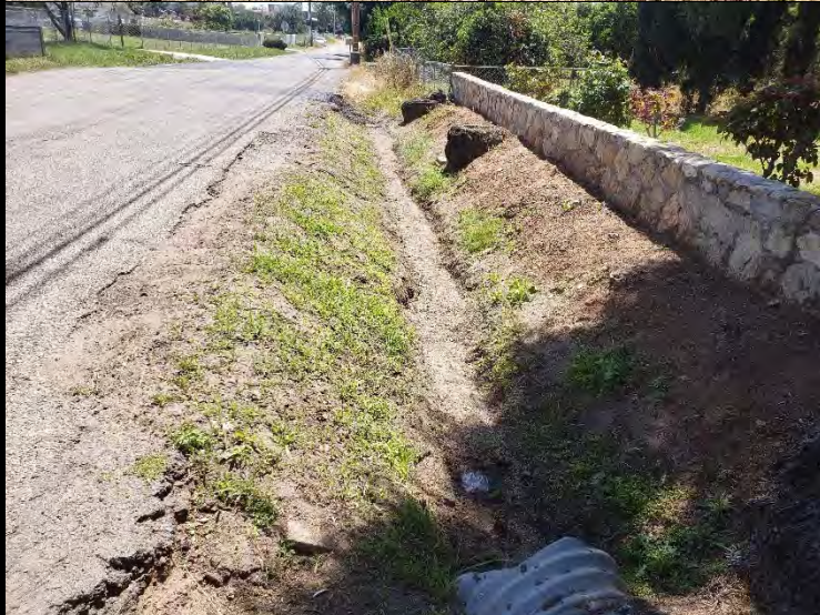
Representative Photograph 2. Facing S. Downstream segment of roadside drainage.
