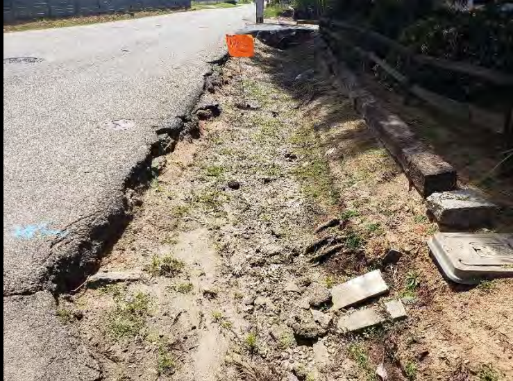
Representative Photograph 1. Facing S. Roadside drainage, mostly unvegetated.
