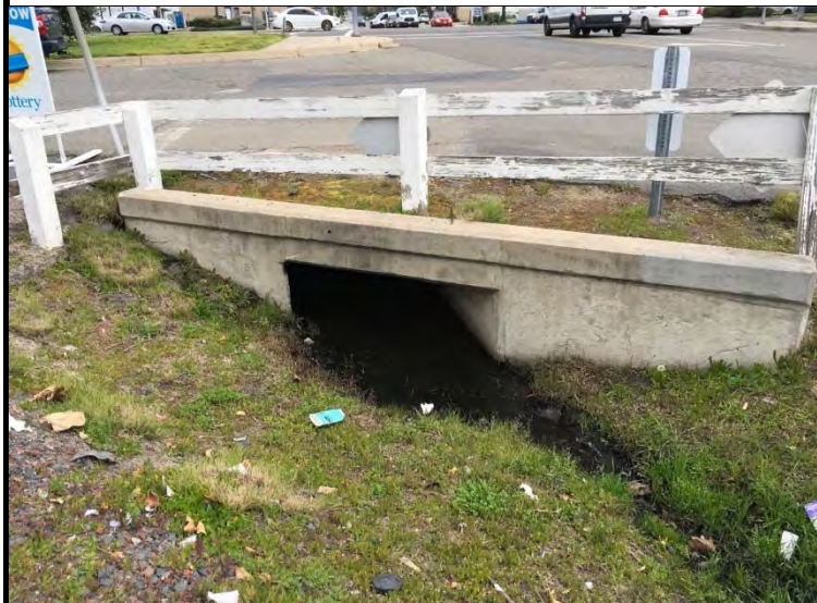
Representative Photograph 1. Facing E. Culvert
