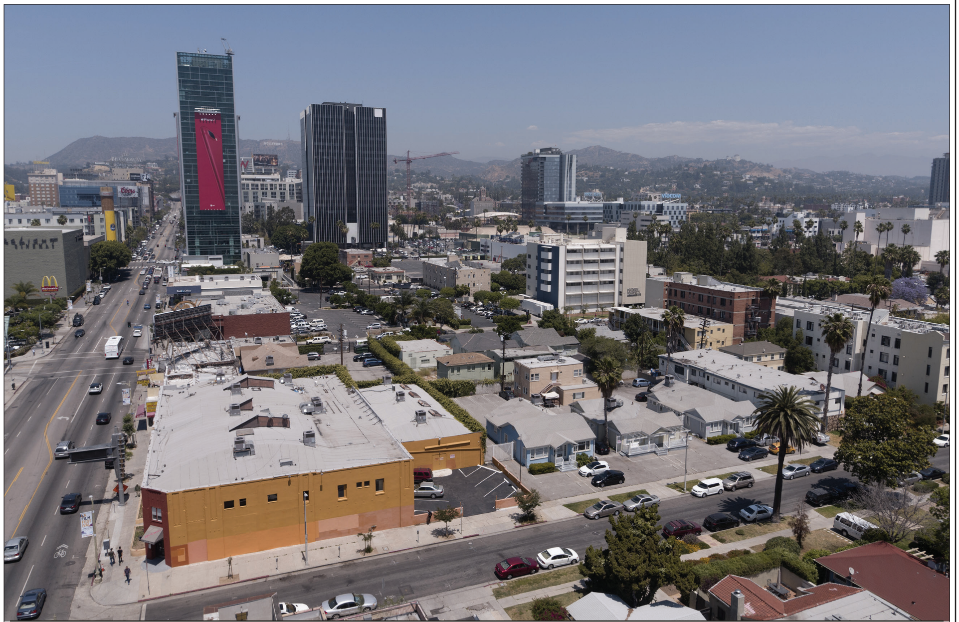
Figure II-3 Aerial of Project Site and Existing Uses Along Afton Place (North)
