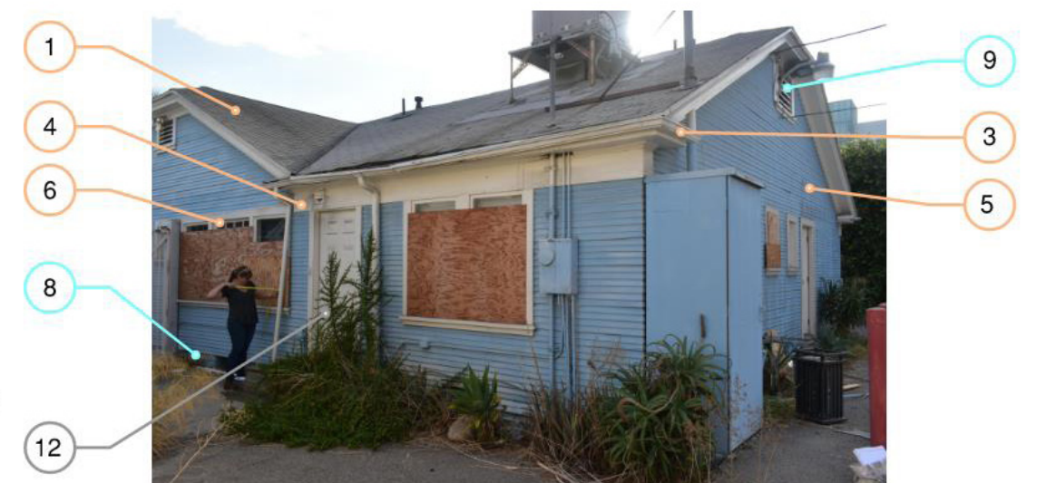
Figure 2: Bungalow 1, North-East corner
