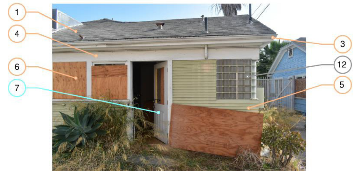
Figure 4: Bungalow 2, North-West Elevation.
