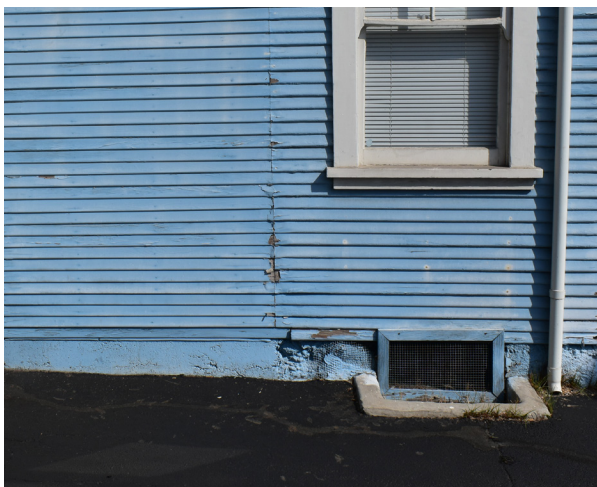
Figure 13: Visible clapboard siding seam.
