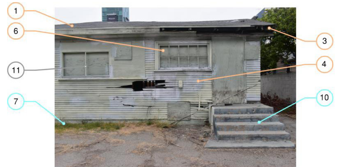
Figure 8: Bungalow 4, South Elevation
