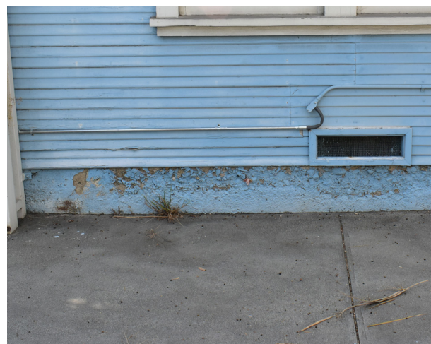
Figure 14: Concrete footing w/ visible aggregate
