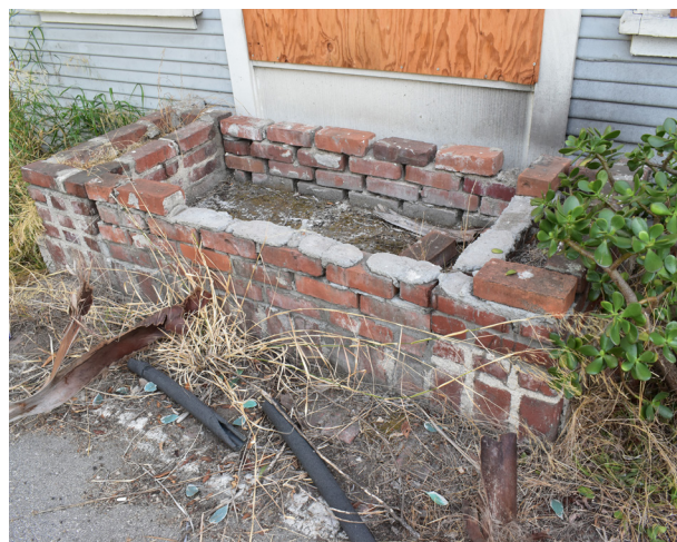
Figure 20: Remains of original brick chimney.
