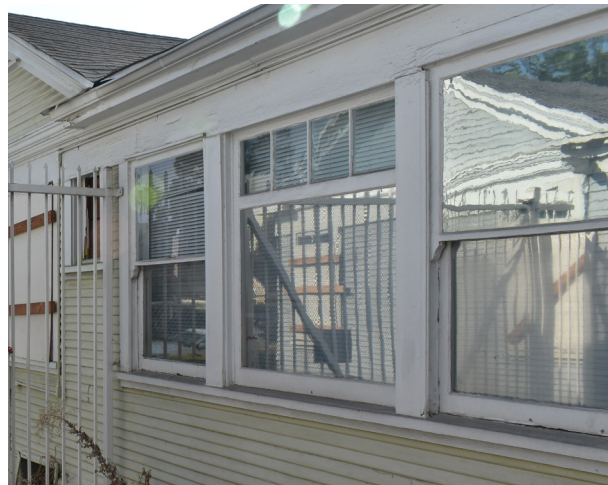
Figure 18: Original wood windows.
