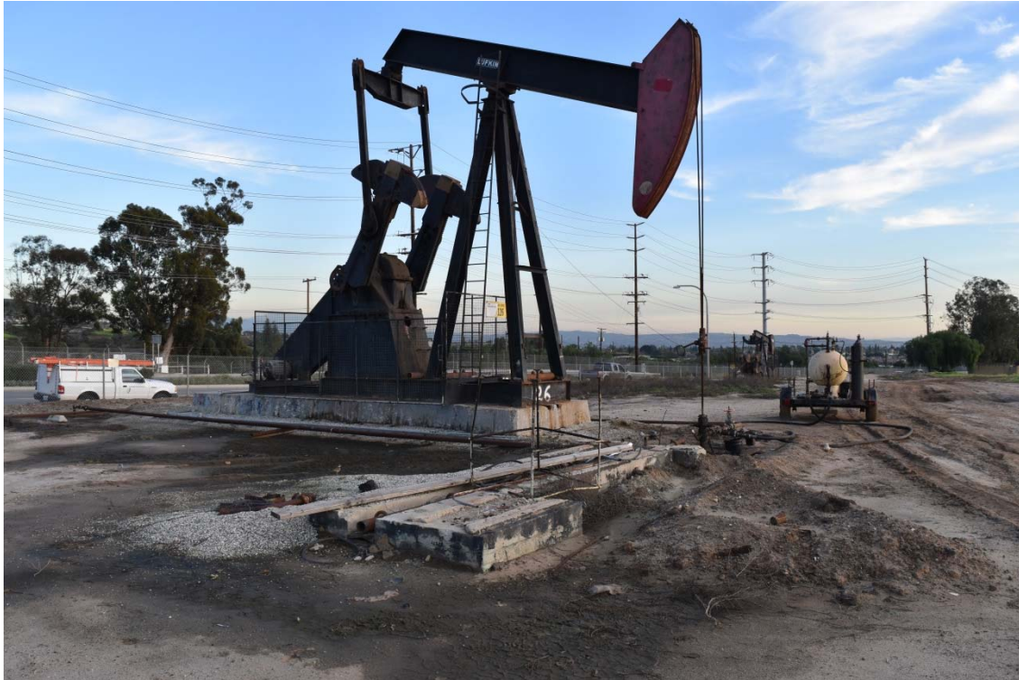
13. Significant staining observed around oil well 126 located on the southern portion of the 100-Acre Parcel near the entry gate from Valencia Avenue..
