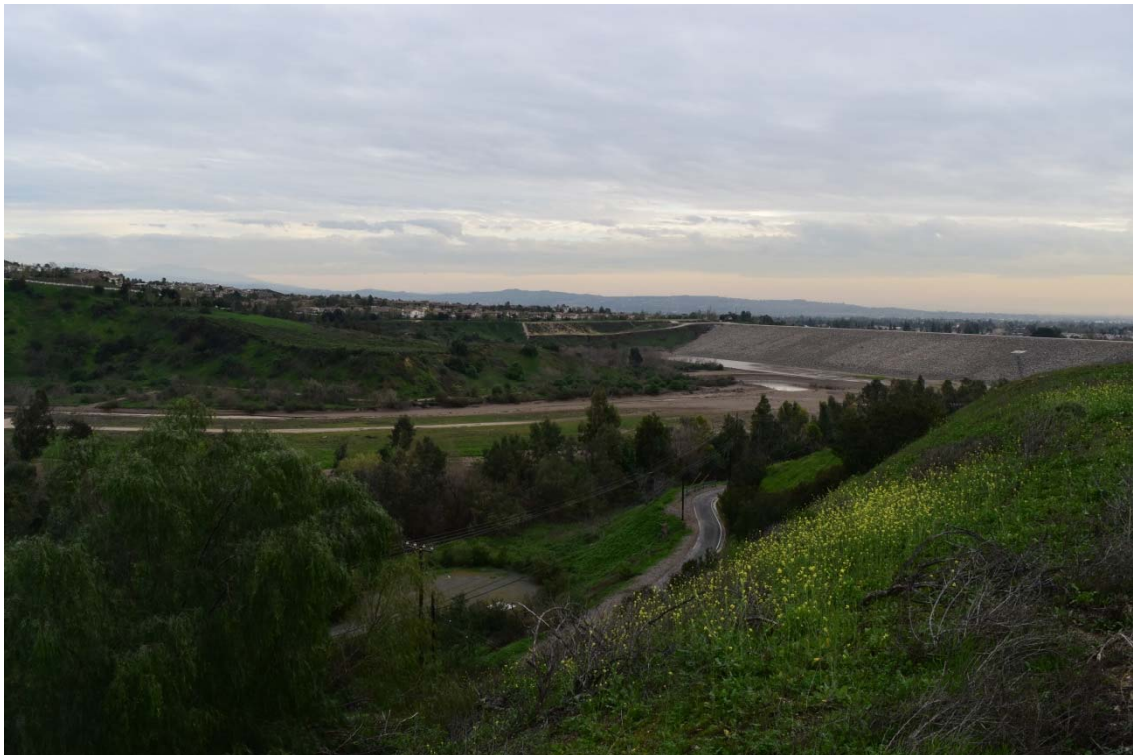
58. Carbon Canyon Dam located east of the 165-Acre Parcel.
