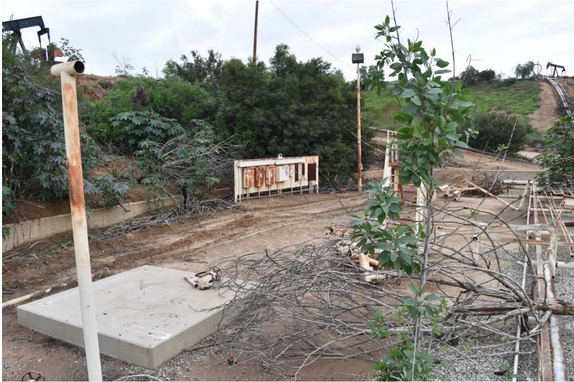
53. Former tank farm location in the south central portion of the 165-Acre Parcel.
