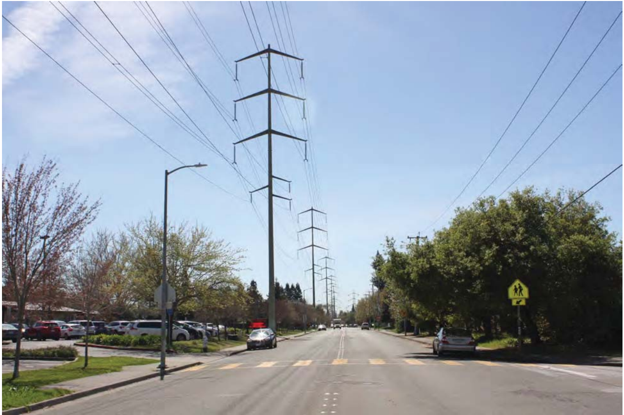
A8. Faught Road at San Miguel Elementary School and Corbett Circle looking south
