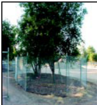
IMAGE 2.15-1 Tree Protection Fence at the Dripline
