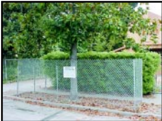
IMAGE 2.15-3 Tree Protection within a Planter Strip
