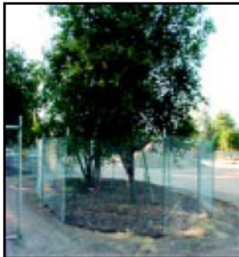
IMAGE 2.15-1 Tree Protection Fence at the Dripline
