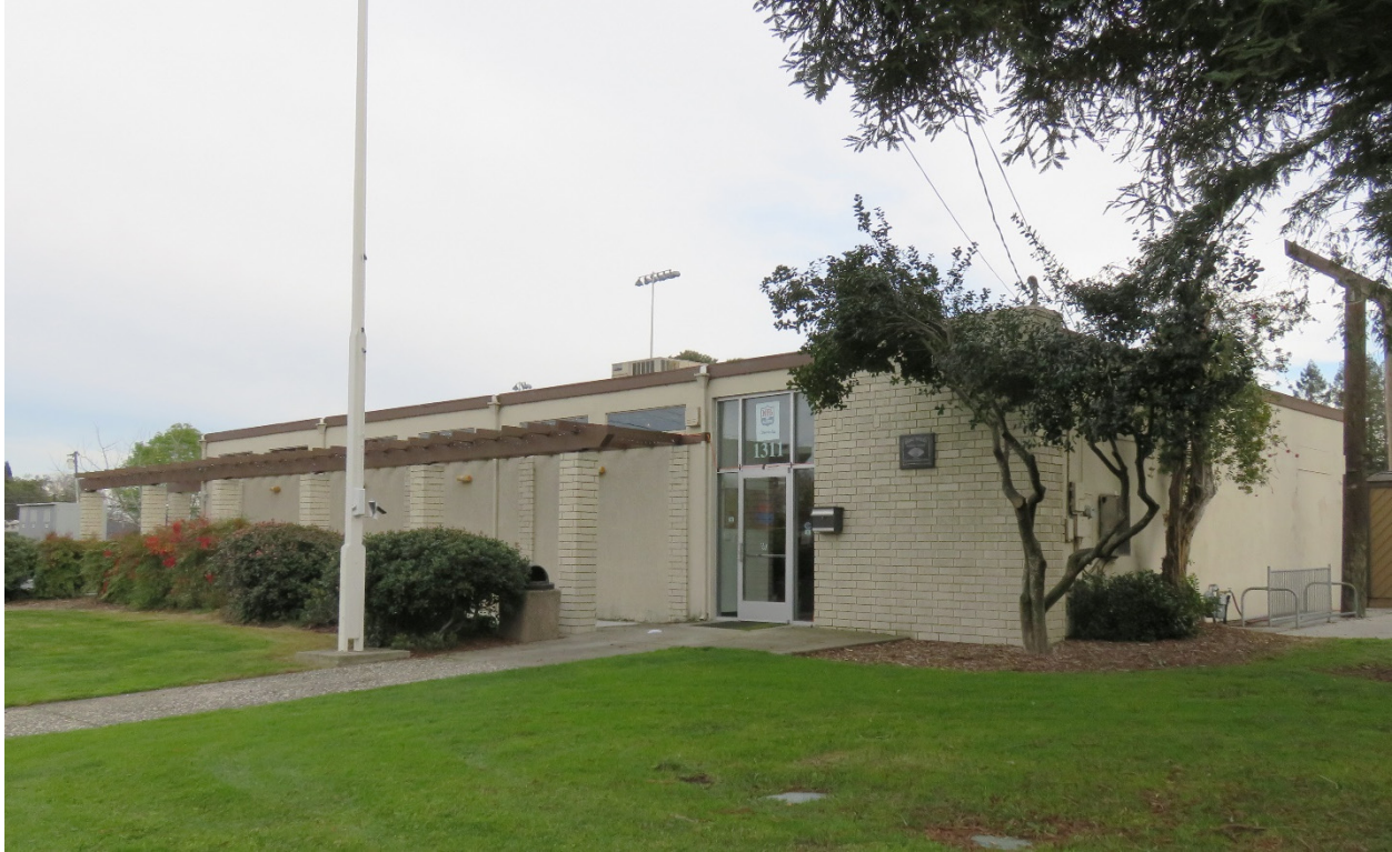
Figure A13. NFL Alumni Building, looking east (Architectural Resources Group, January 2017).
