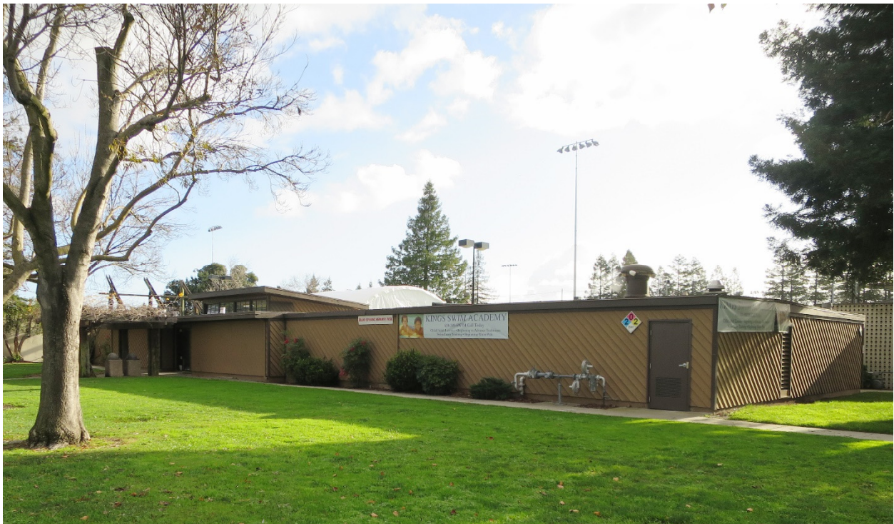
Figure A12. Herkner Memorial Swim Center, looking east (Architectural Resources Group, December 2016).
