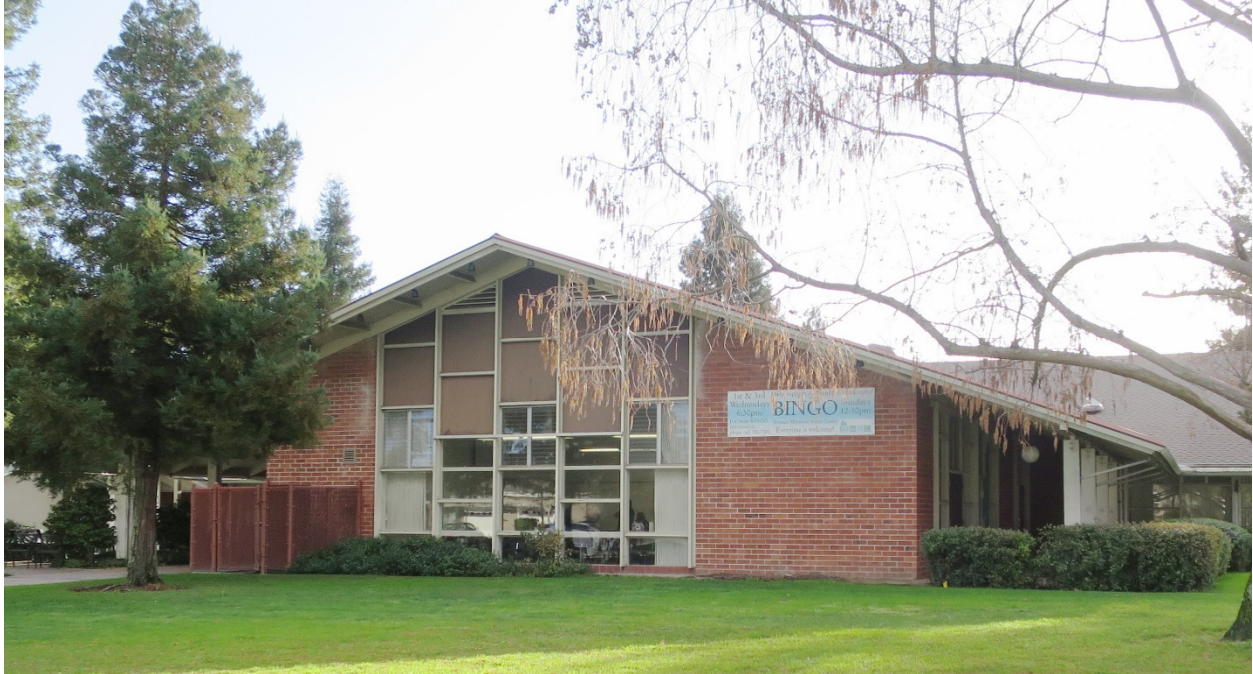
Figure A3. Veterans Memorial Building, northwest wing (Architectural Resources Group, December 2016).
