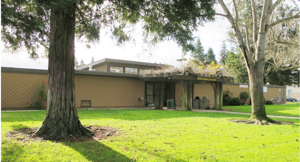
Figure A11. Herkner Memorial Swim Center, looking south (Architectural Resources Group, December 2016).
