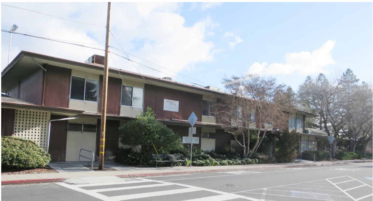
Figure A10. Senior Center Annex, looking east (Architectural Resources Group, December 2016).
