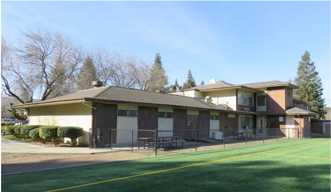
Figure A9. Senior Center Annex, looking west (Architectural Resources Group, January 2017).
