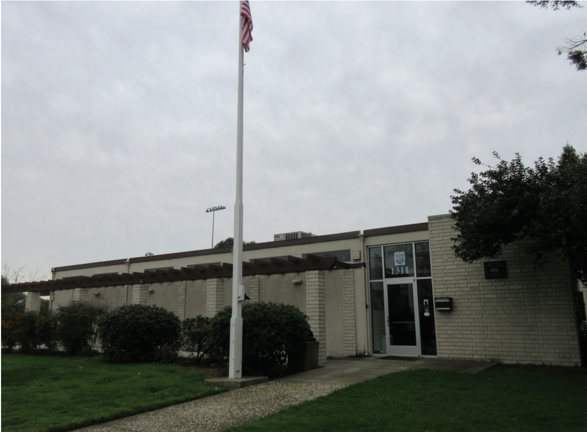
Photo 3: View of NFL Alumni Association Building from sidewalk on Madison Avenue, facing south.
