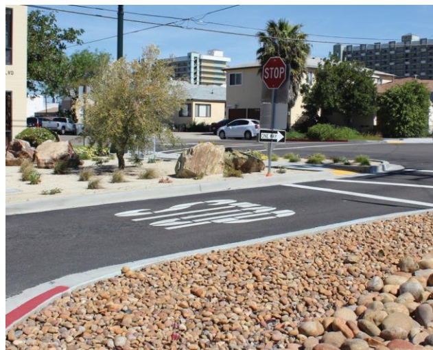
Curb extension and bioswale on Plaza Boulevard
