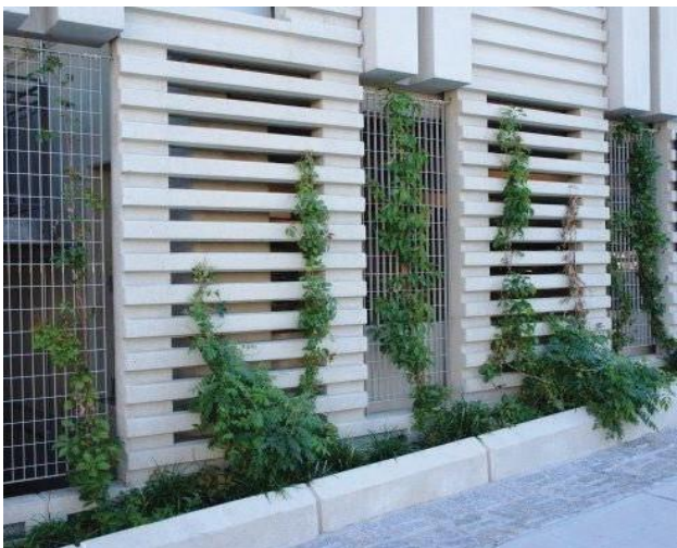
Planted divider improves a parking structure facade
