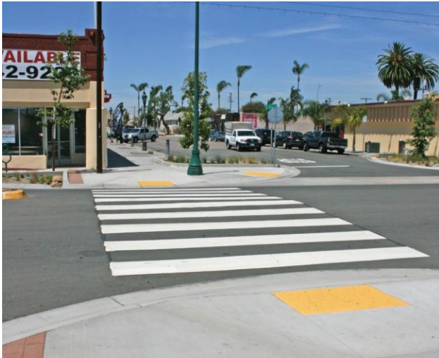
Curb extension on 8th Street
