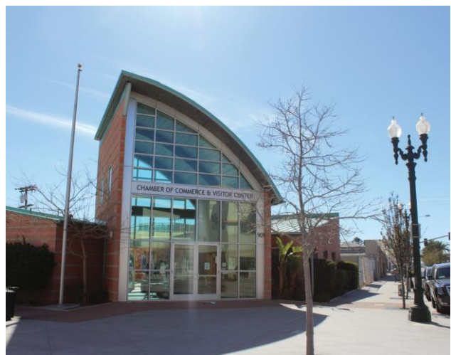
Chamber of Commerce glass façade uses clear non-reflective glass creating a desirable street-level building transparency
