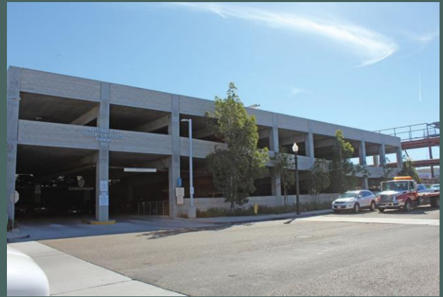
National City Education Village Parking Garage
