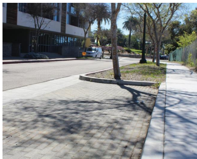
Permeable paving on A Avenue
