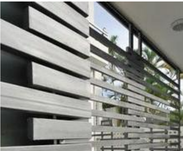
Concealing building facade treatment
