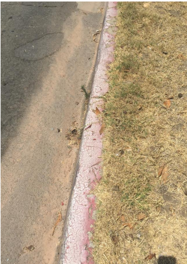
Figure 5-8: Inadequate Curb Marking Example
