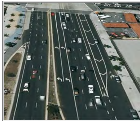
Shared bicycle-right turn lanes require warning signage as well as pavement markings.
