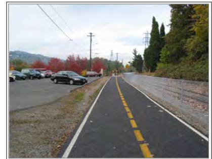
Open boundaries can be created where users may be entering the trail.
