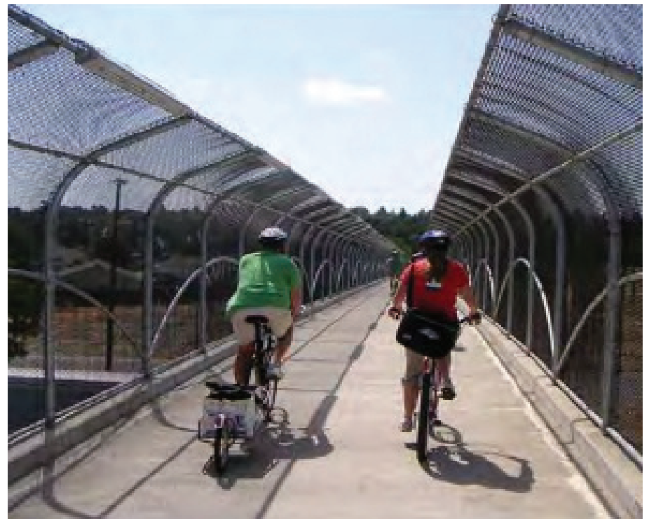
Crossing over a freeway
