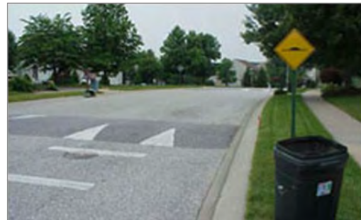
Speed humps are a common traffic calming treatment.
