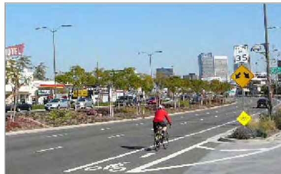
Where on-street parking is not allowed adjacent to a bicycle lane, bicyclists do not require additional space to avoid opened car doors.
