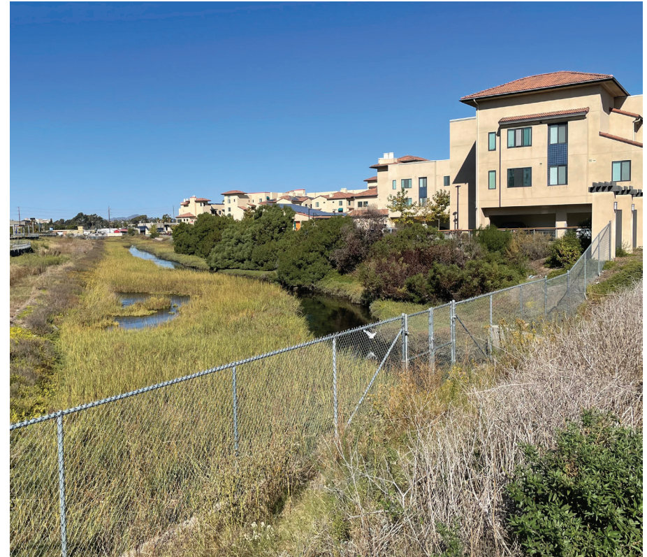
Multi-family residential development adjacent to Paradise Creek
