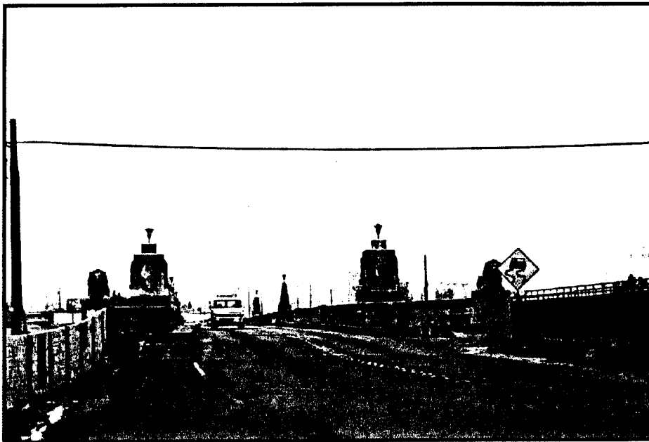
Photo 6. View northwest of Seventh Street Bridge with SPRR Bridge to right.
