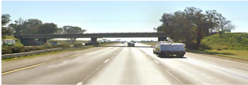
South view of American Avenue over State Route 99
